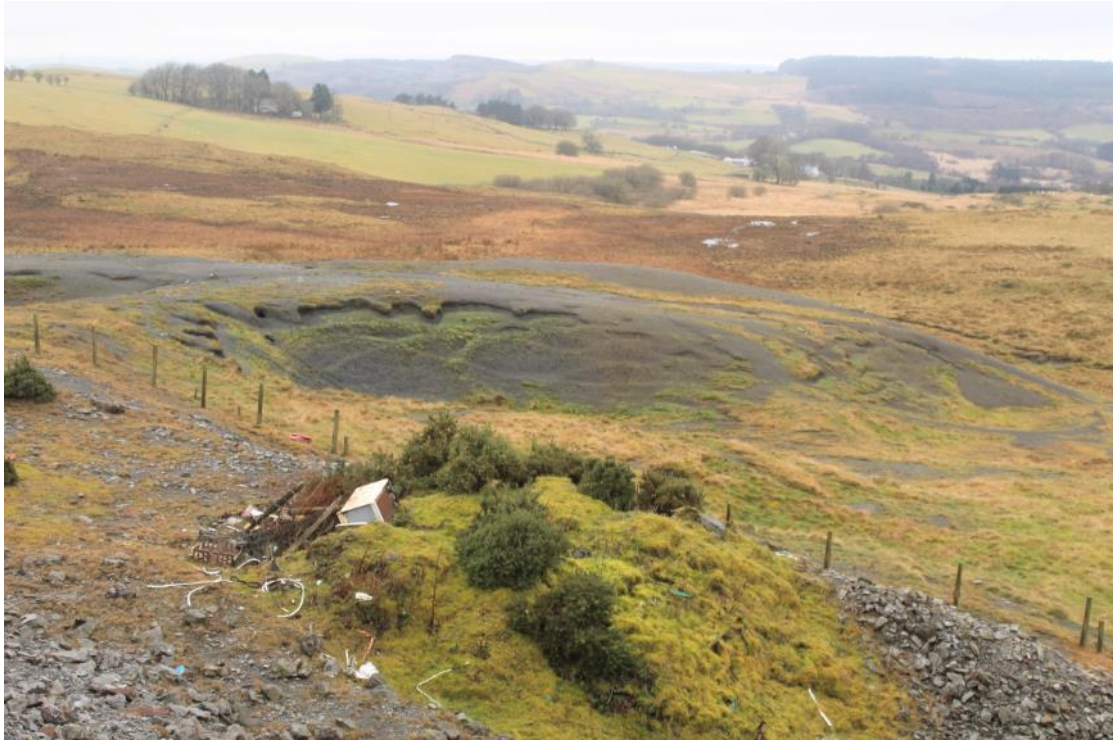
Photo 47: Looking west across the depression that may represent a collapsed shaft GF03 .
