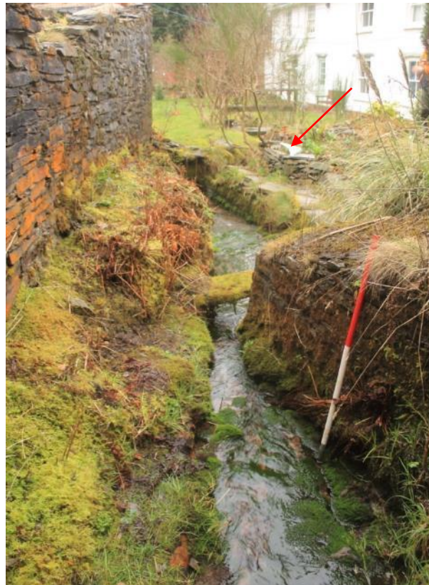
Photo 9: View northwest along the line of leat LF01 as it emerges from Level Fawr adit. On the right the brick built modern culvert intrudes, with the diverted water course heading to the left, the original line lies to the right (arrow). 1m scale.
