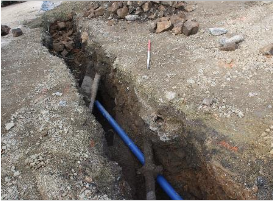
Photo 119: Showing service pipes revealed in cable trenches south of the wharf. View north-west. 1m scale.
