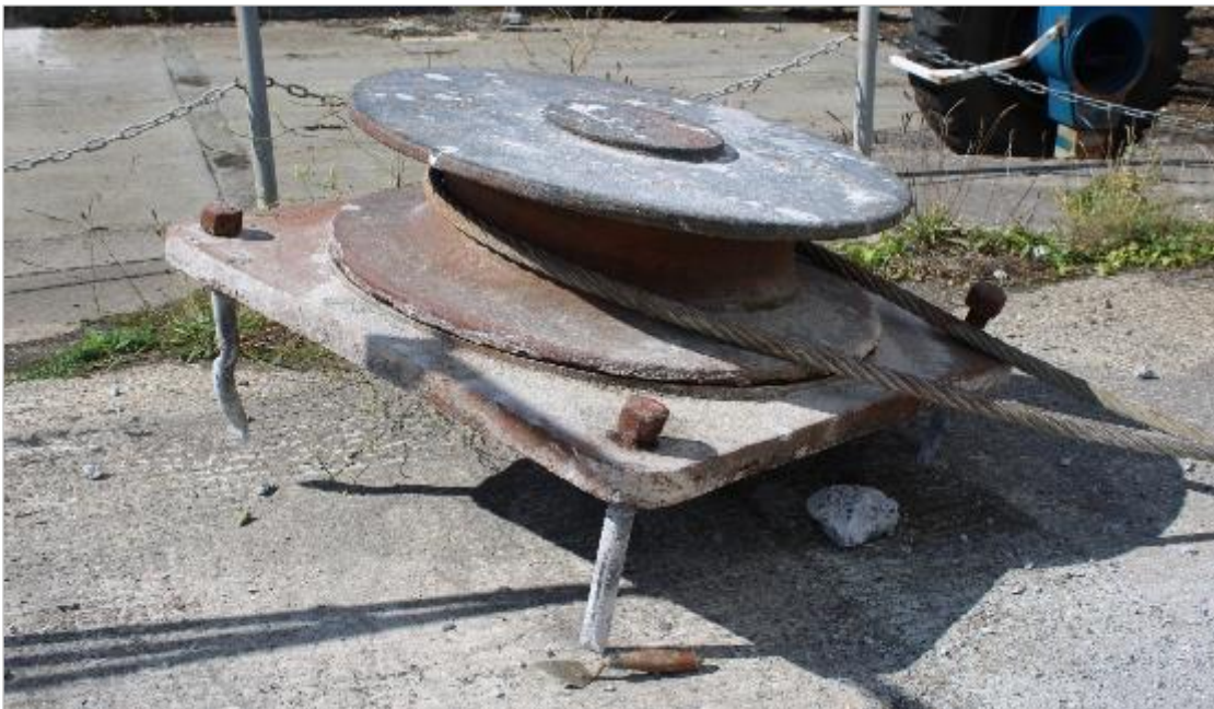
Photo 113: Showing a mooring fairlead roller removed from the front of the wharf. No scale.
