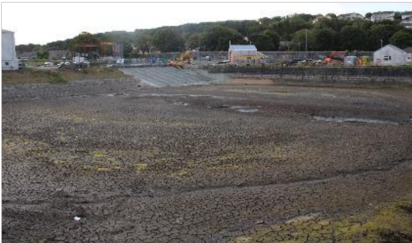
Photo 89: Protective sheeting placed on the eastern slope of the timber pond, where the vehicle access ramp will be constructed. View south-east. No scale.
