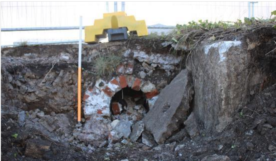
Photo 22: Showing a brick drain revealed by removal of part of the wharf east of Slipway 2. View east. 1m scale.
