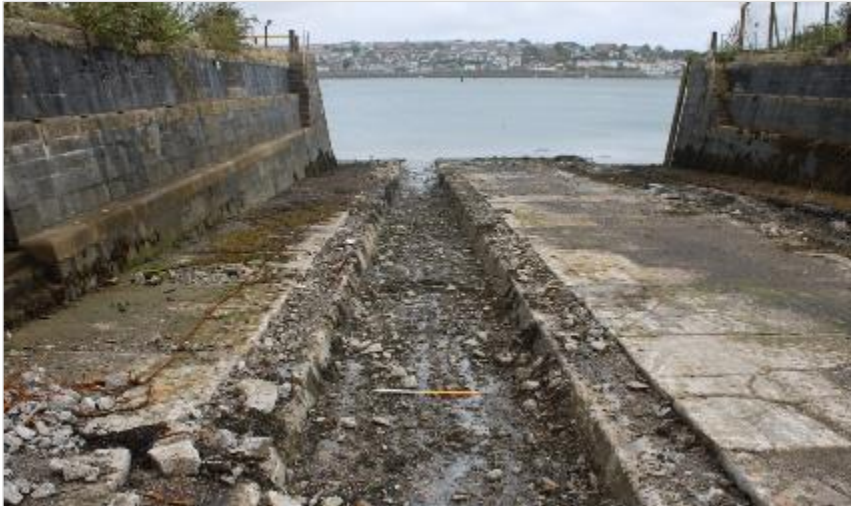
Photo 10: Channels revealed within Slipway 2 following removal of concrete runners. View north. 1m scale.
