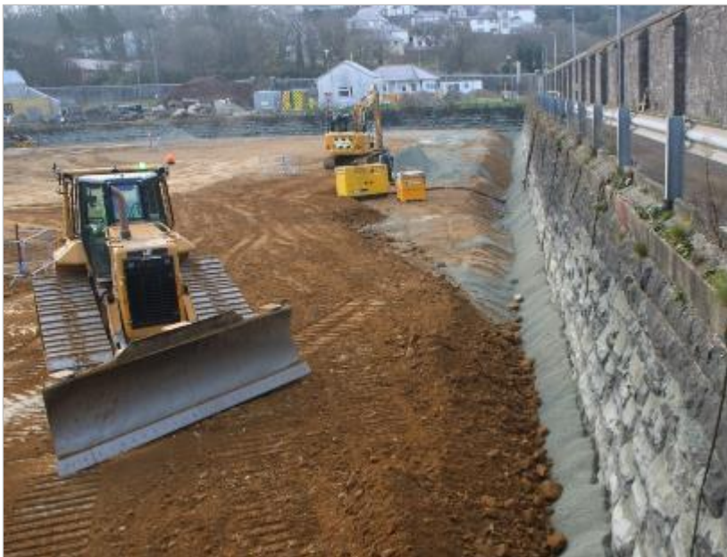
Photo 101: Close-up of work to infill the timber pond. The drain in the west wall is now completely covered up. View south. No scale.
