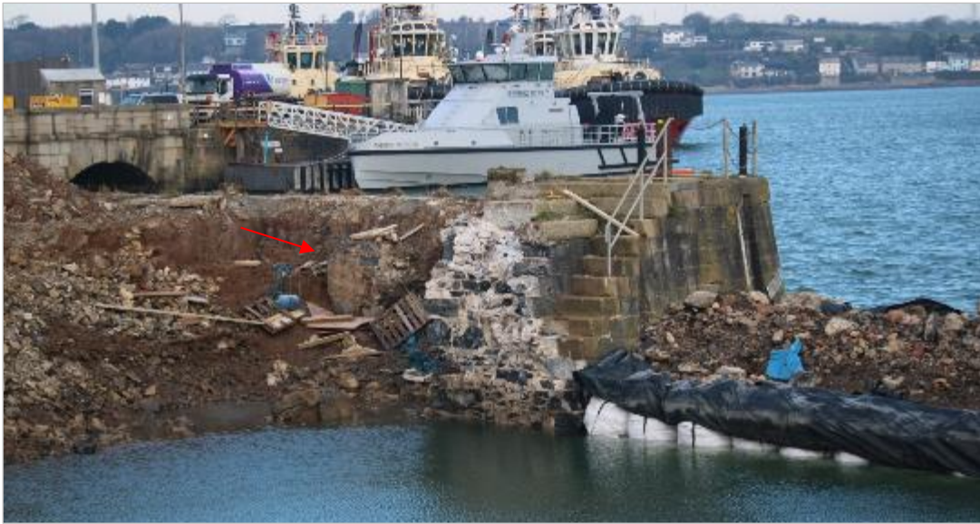
Photo 45: Showing the internal structure of the eastern wall and the end of the wharf, following demolition of the remainder of the wall. The remains of the privy are just becoming visible (red arrow) View north-west. No scale.
