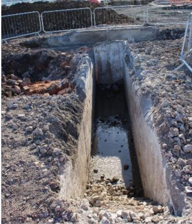
Photo 74: The concrete inspection pit which truncated the brick drain (visible to the left of shot). View east, 1m scale.
