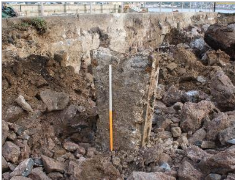
Photo 50: Remains of metal stanchion after removal of surrounding plinth. View north-west. 1m scale.
