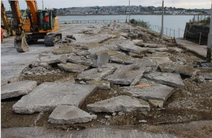
Photo 67: Sandy levelling deposit emerging below the concrete at the north end of the wharf. View north. 1m scale.
