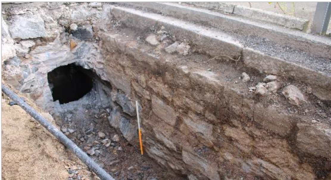
Photo 107: Showing the sluice gate housing revealed during excavation of a pipe trench west of the timber pond. View north-east, 1m scale.
