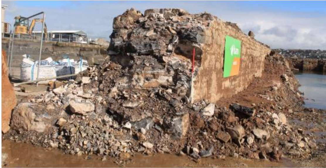
Photo 42: Close up showing the structure of the western wall of the wharf/eastern wall during Slipway 1 demolition. View north. 1m scale.
