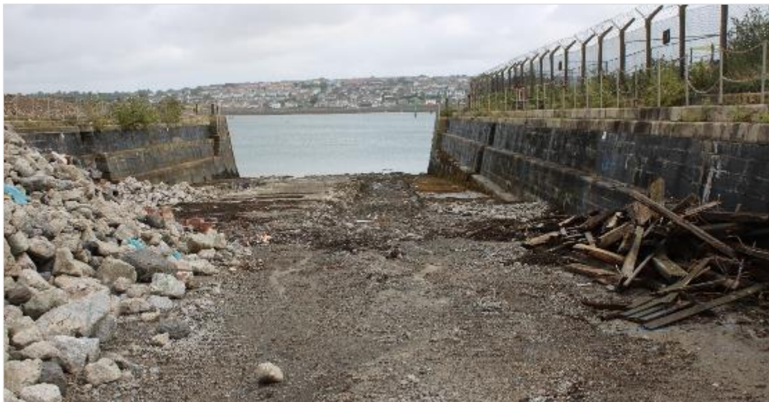
Photo 14: Slipway 2 following removal of the concrete runners. View north. 1m scale.
