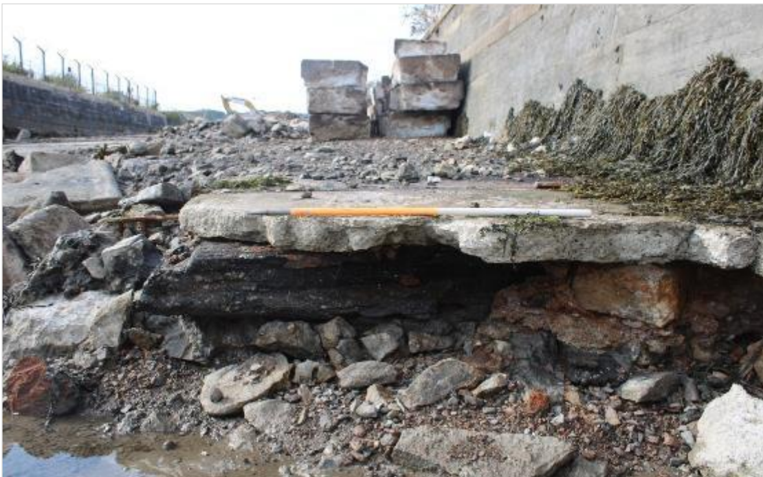
Photo 05: Showing a large timber beneath the concrete slab surface at the northern end of Slipway 2. View south. 1m scale.
