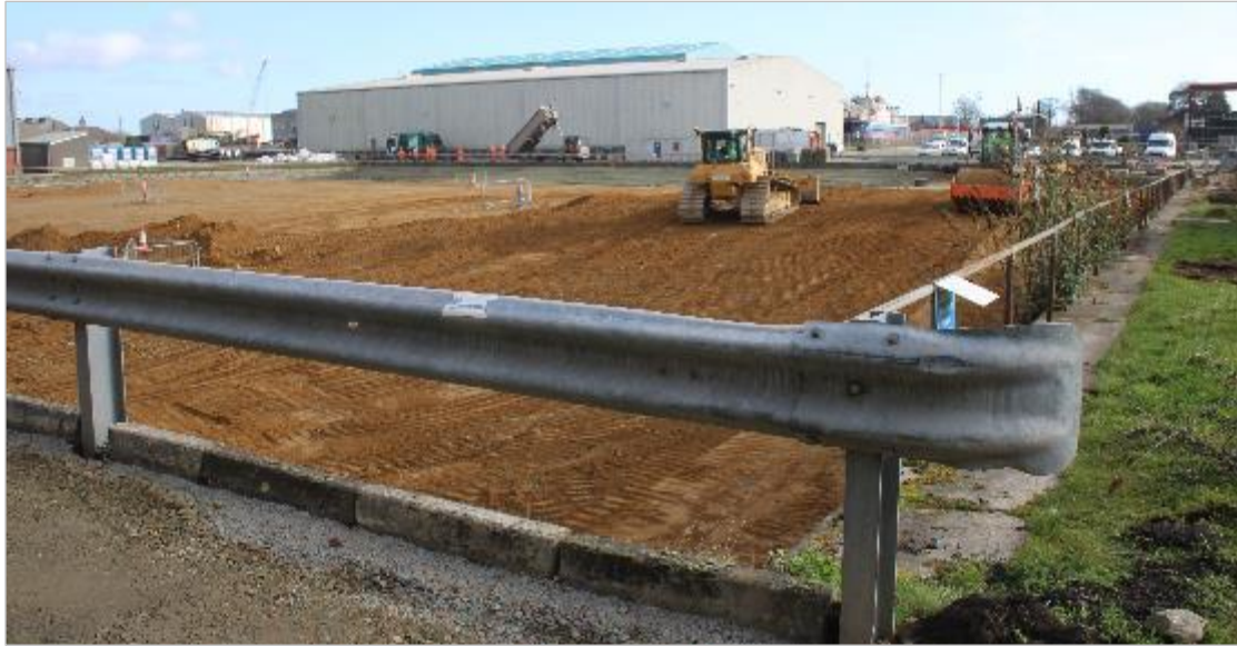
Photo 106: Infill of the timber pond nearing completion. View north-west. No scale.
