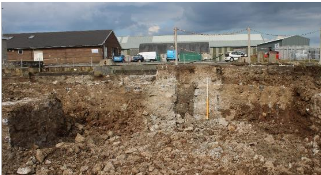
Photo 48: Showing a vertical notch in the internal face of the wharf wall. View west. 1m scale.
