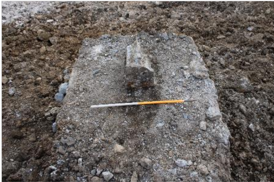
Photo 52: Close-up showing a sheared-off metal stanchion set into one of the plinths revealed within the wharf. View east, 1m scale.
