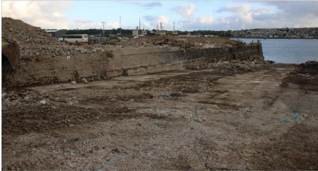
Photo 47: Showing a change of build/phase in the south end of the eastern wall of the wharf/western wall of Slipway 2. View north-west. 1m scale.
