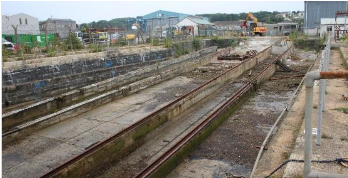
Photo 08: Slipway 2 prior to demolition work commencing. Signs at the top of the slipway read 'Slip 1' (right) and 'Slip 2' (left). Concrete runners and metal track can be seen. View south-east. No scale.
