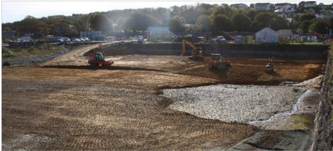
Photo 97: Showing deposits at the bottom of the timber pond almost completely covered with the first layer of sand and aggregate. View south-south-east. No scale.
