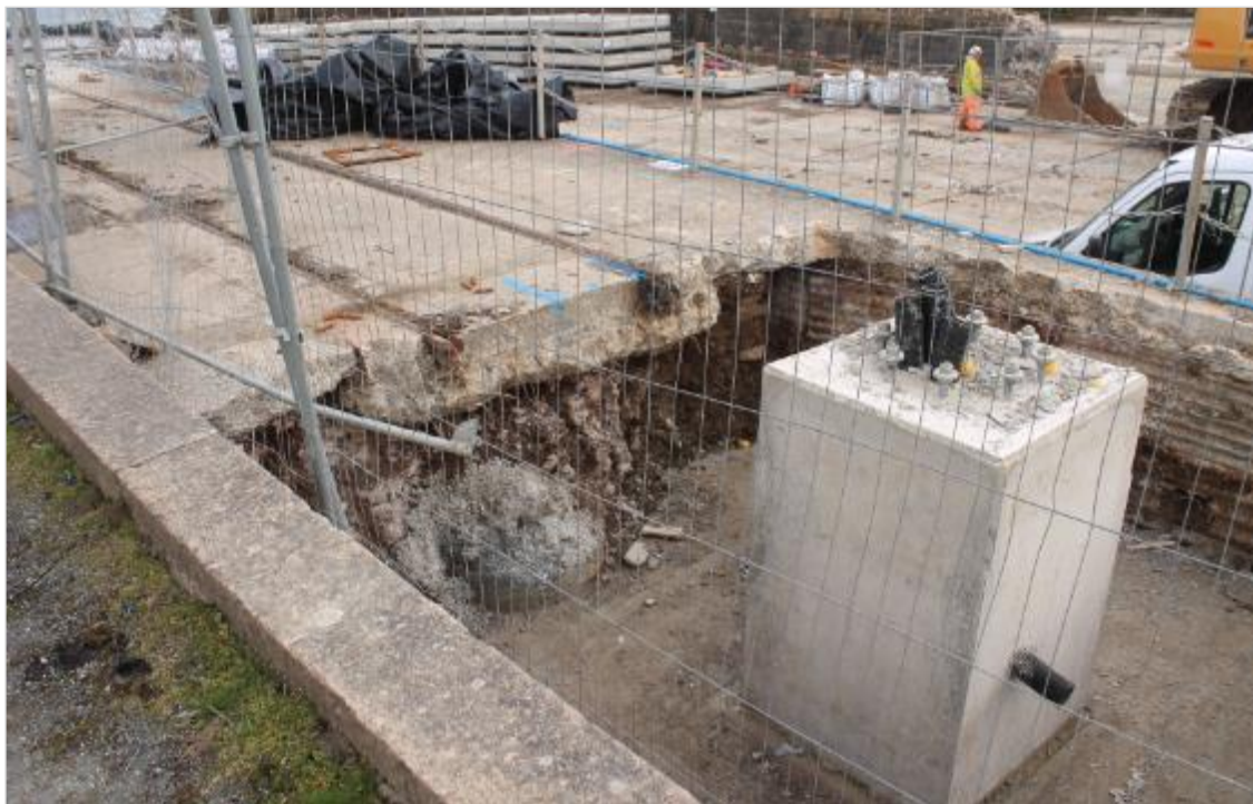
Photo 36: Showing differing deposits below Slipway 1 during work to install floodlights. View north-east. No scale.
