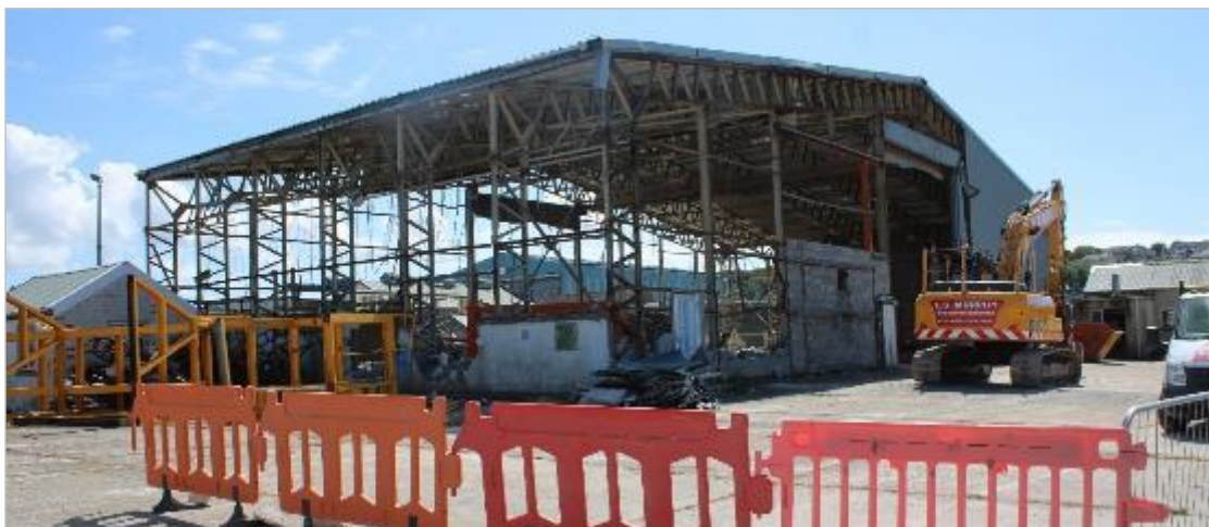
Photo 80: The shed following removal of corrugated sheets on the western, northern and eastern sides. View south-east. No scale.
