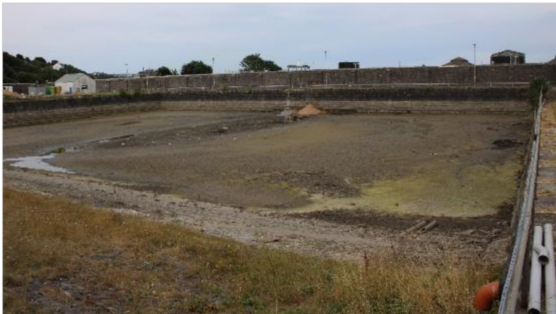
Photo 84: The timber pond prior to infilling. The opening for the sluice gate in the west wall has been blocked with sand. View south-west. No scale.
