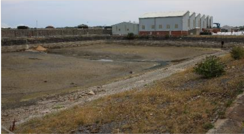
Photo 85: The timber pond prior to infilling. The drain in the west wall has been blocked with sand. The drain in the north wall is visible. View north-west. No scale.
