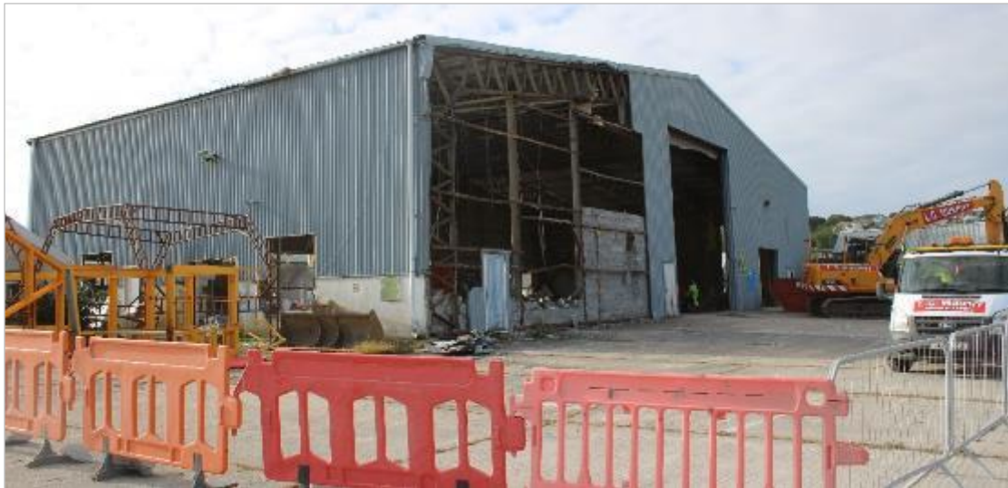
Photo 79: The shed following removal of windows and doors, and part of the western side. View south-east. No scale.
