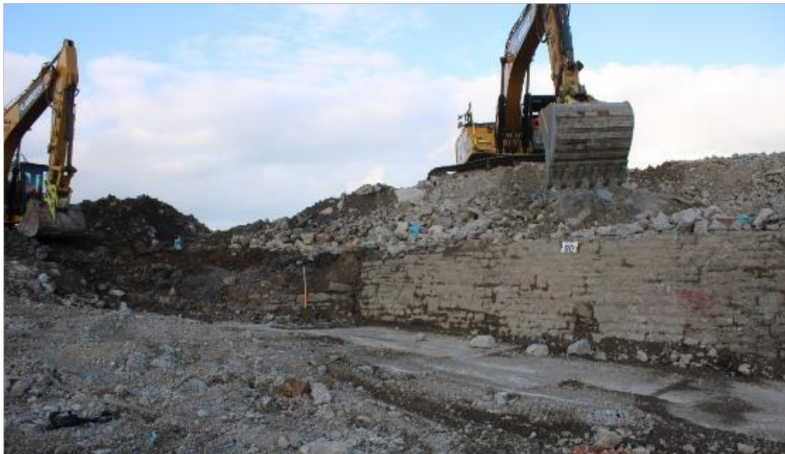
Photo 46: Showing a dogleg in the eastern wall of the wharf/western wall of Slipway 2. View south-west. 1m scale.
