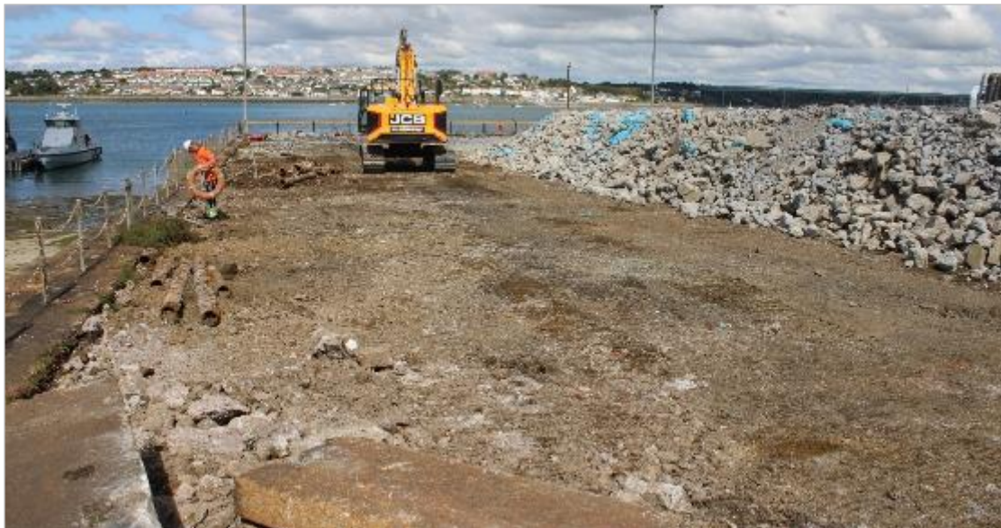
Photo 66: Sandy levelling deposit below the concrete surface at the north end of the wharf. Note that several sections of iron pipe have been removed. View north. No scale.
