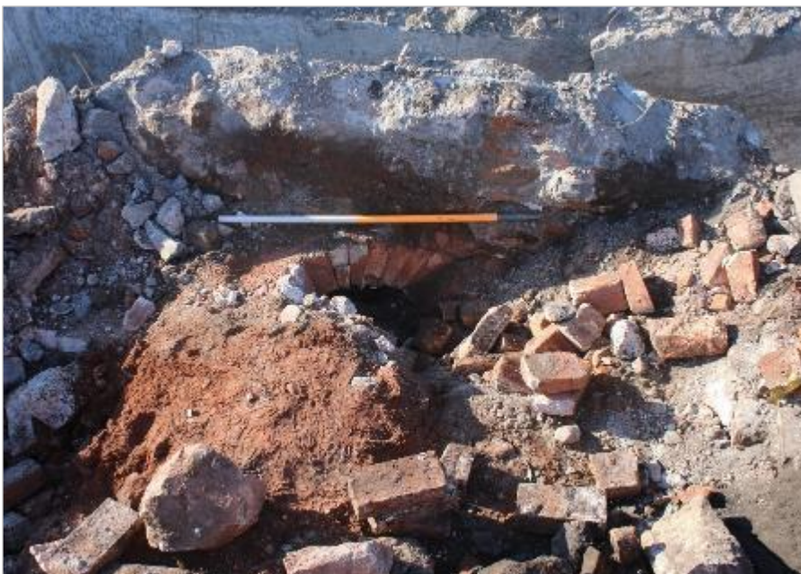
Photo 73: Detail of an arched brick structure truncated by a concrete inspection pit, revealed below-ground following removal of the shed. View south, 1m scale.
