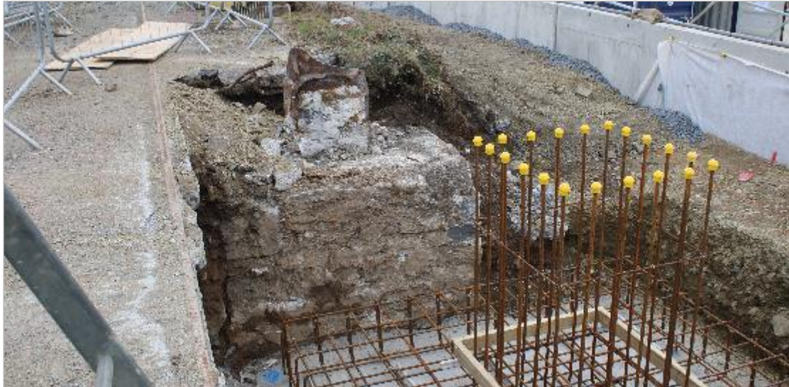
Photo 117: Showing a rail and one of two blockwork plinths containing a metal stanchion revealed within the wharf between Slipway 2 and the graving dock. View south-west. No scale.
