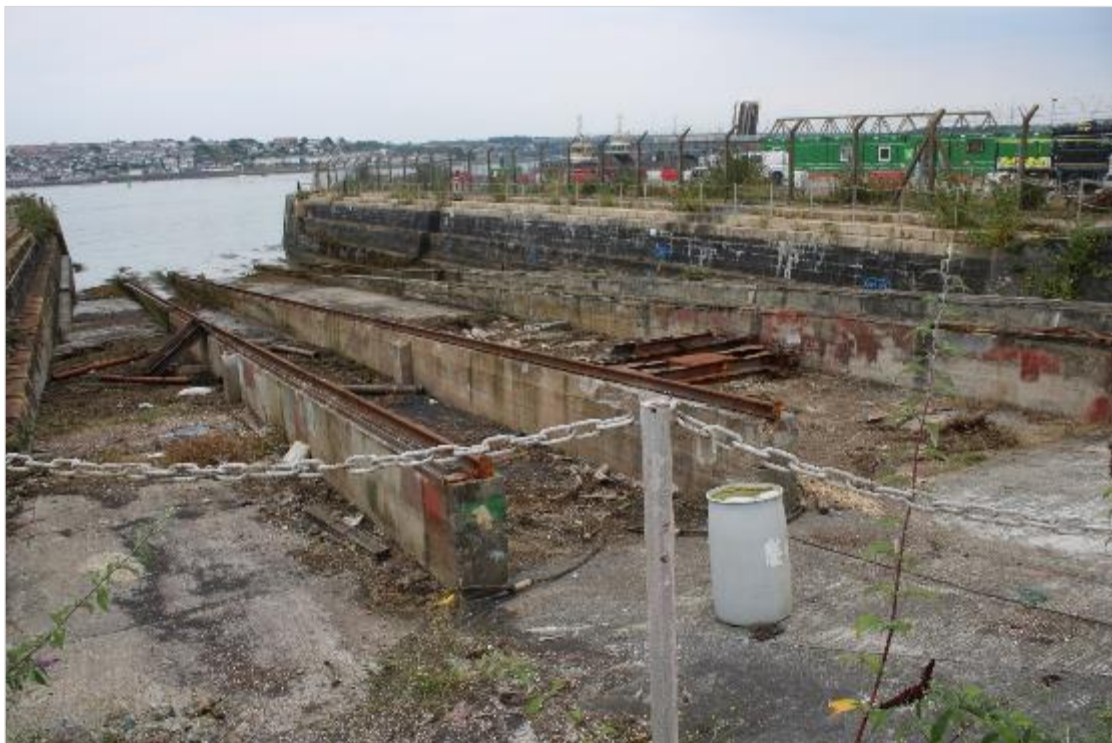
Photo 09: Showing both pairs of concrete runners and metal tracks on Slipway 2. View north-east. No scale.
