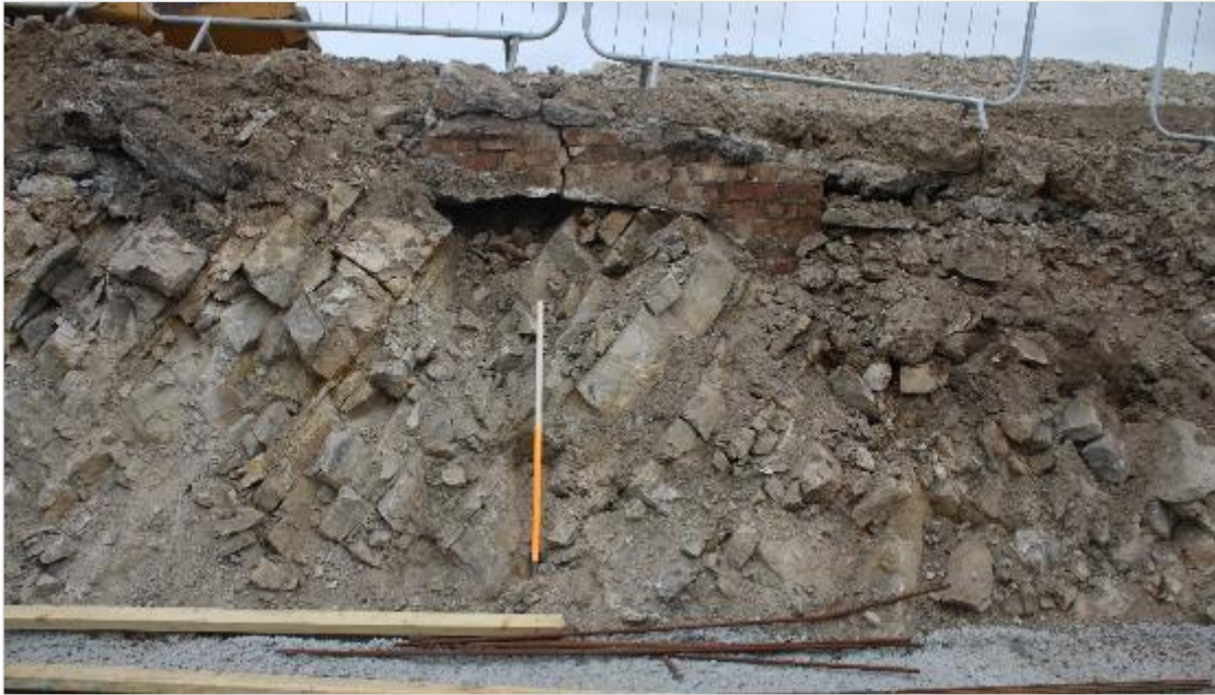
Photo 04: Showing brickwork constructed over bedrock below the surface of Slipway 2. View west. 1m scale.
