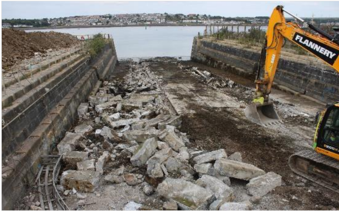
Photo 13: Demolition of concrete runners on Slipway 2. View north.
