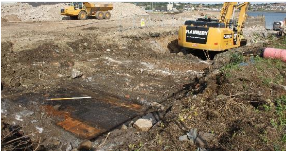
Photo 07: Showing a pair of substantial timbers set in coal dust/masonry at the top (south end) of Slipway 2. View north-west. 1m scale.
