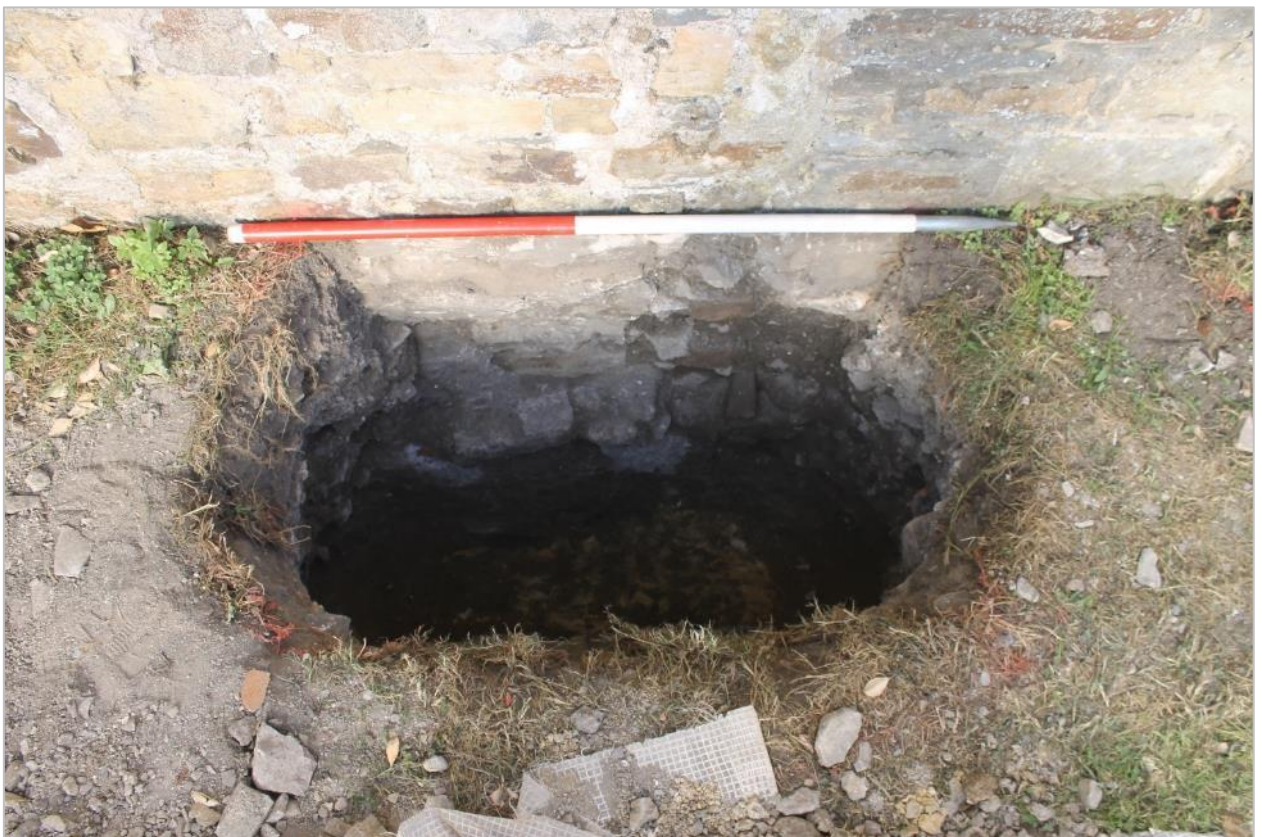
Photo 18: Test Pit 5, showing a poorly bricked up hole in the eastern gable wall of the gaol. Looking west, 1m scale.
