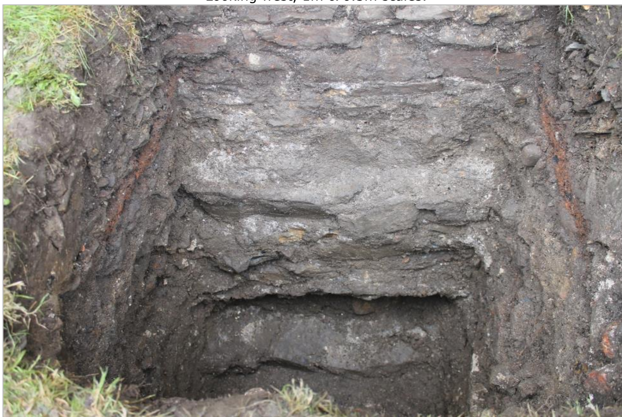
Photo 11: Close-up of the relationship between the gaol wall and an earlier wall in Test Pit 1. Looking south, no scale.
