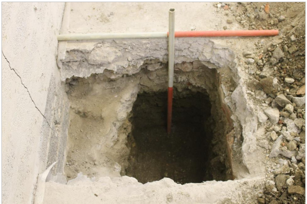
Photo 9: Showing earlier red brick floor and concrete bedding below the modern floor in Test Pit 11. Looking west, 2 x 1m scales.
