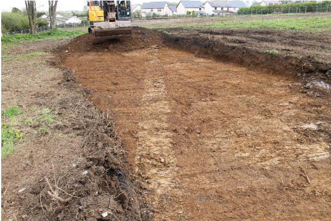
Photograph 6: Fill of land drain crossing base of road-cut. Looking east.
