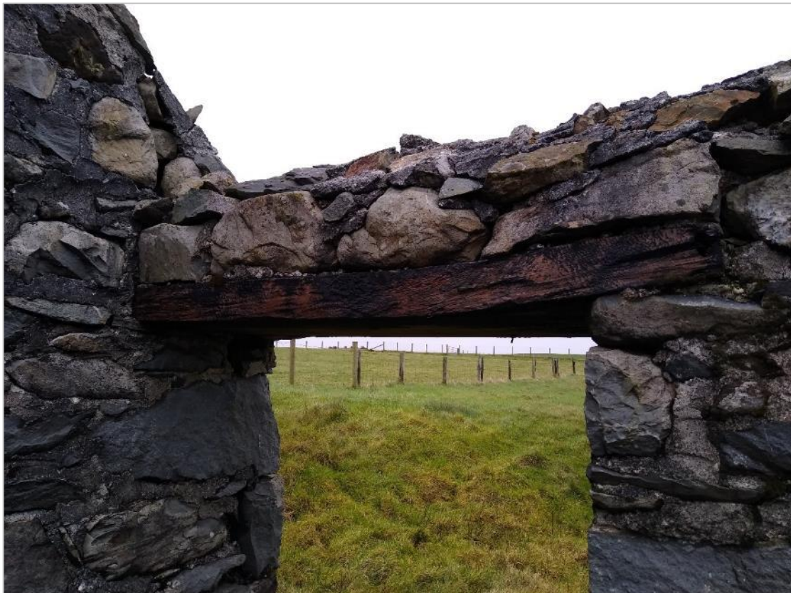
Photo 12: Detail of timber lintel in entrance.
