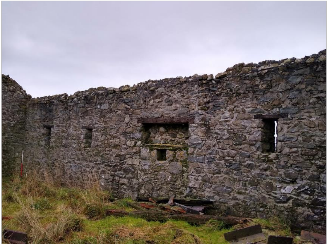
Photo 21: West wall, blocked entrance (with slate shelf) and ventilation slits.
