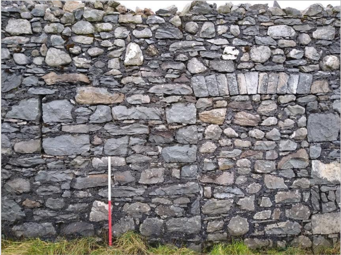
Photo 7: Ventilation slit and blocked entrance in Bay 2, east elevation.
