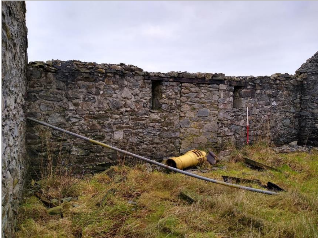
Photo 15: Blocked entrance and ventilation slits in west wall.
