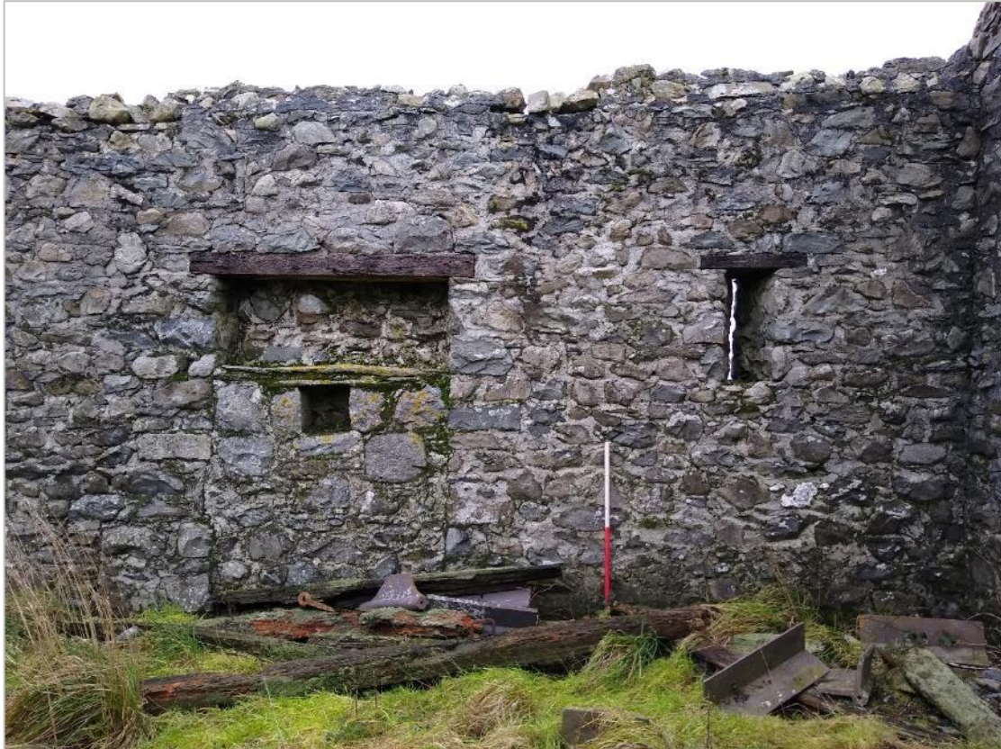
Photo 22: Close-up of shelf and square recess incorporated into blocked entrance.
