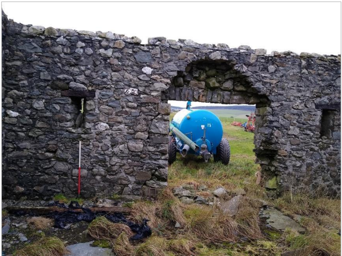
Photo 19: Lintel, inner voussoirs and base at south side missing
