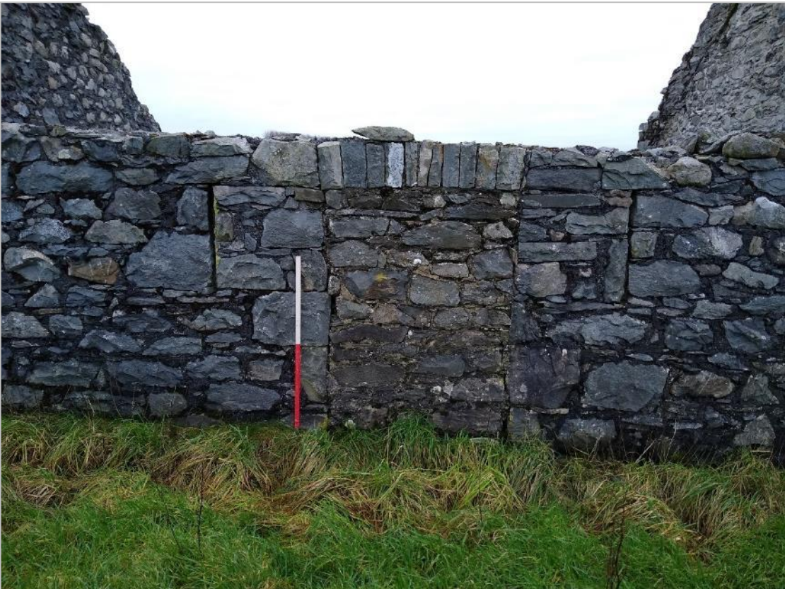
Photo 8: Ventilation slits and blocked entrance in Bay 1, east elevation.
