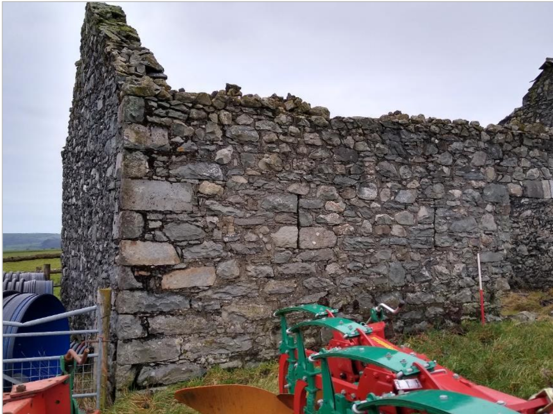
Photo 4: Ventilation slits and quoins in the east elevation of Bay 2.
