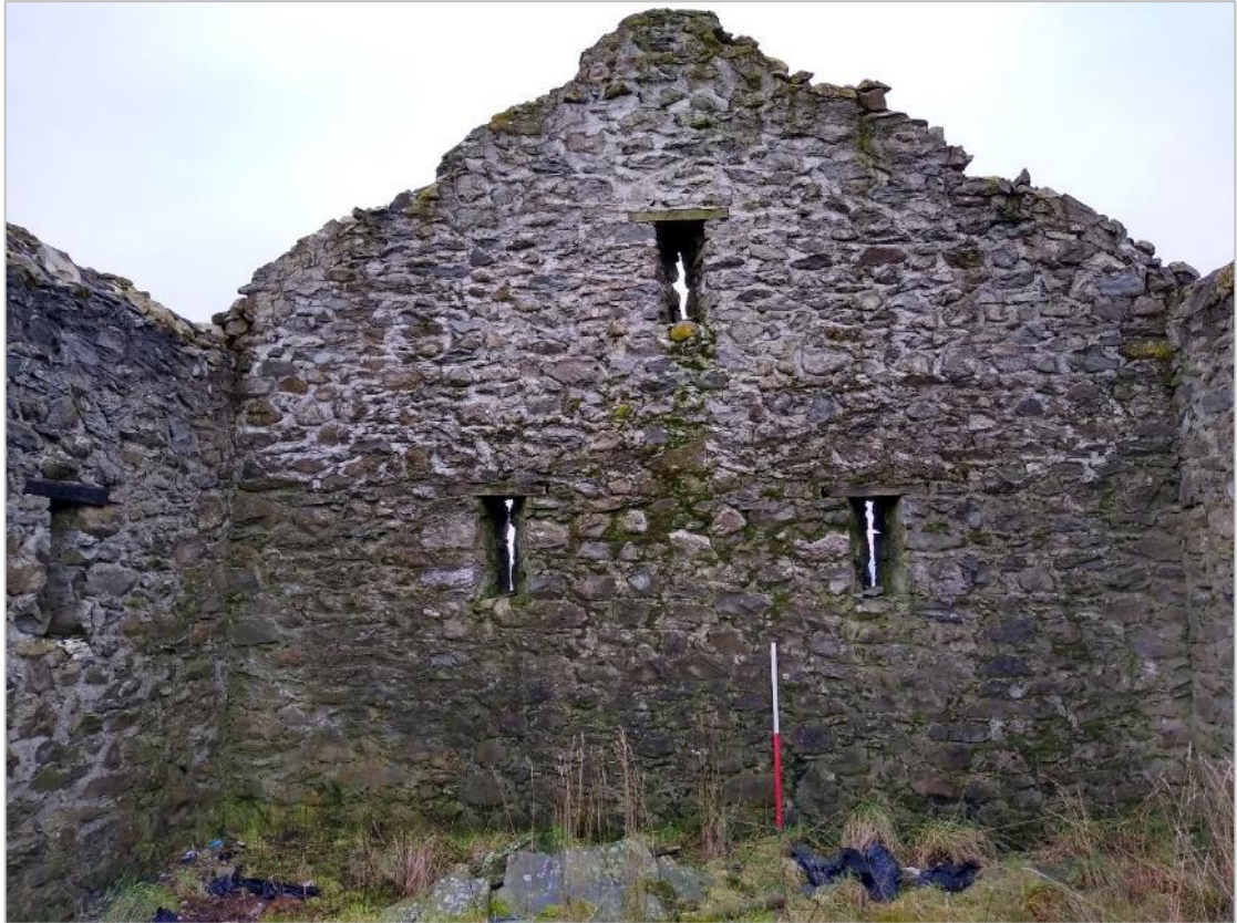
Photo 20: South gable wall and ventilation slits.
