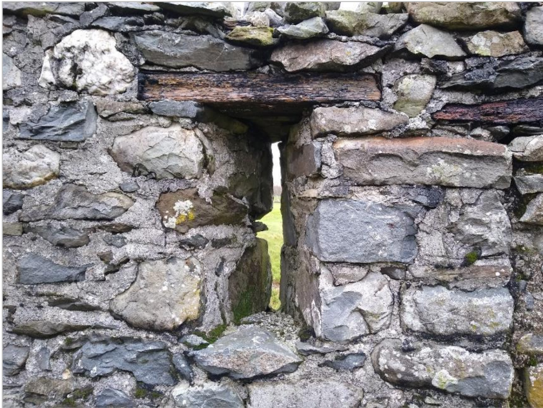
Photo 13: Close-up of ventilation slit and timber lintel.
