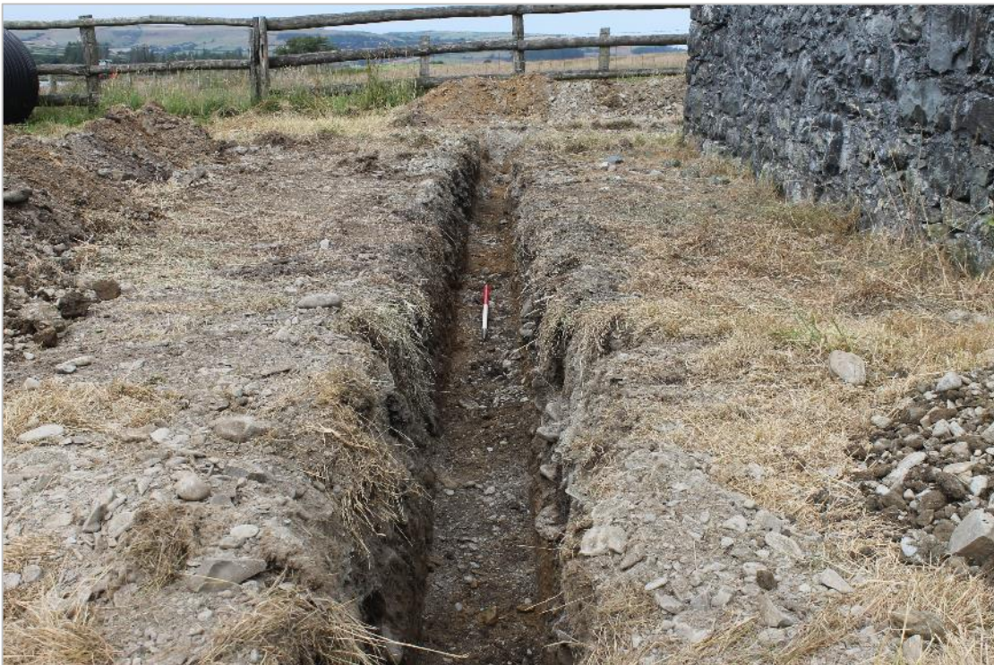
Photo 26: Showing the service trench excavated adjacent to the south-west facing gable wall of the property. Looking north-west, 1m scale.
