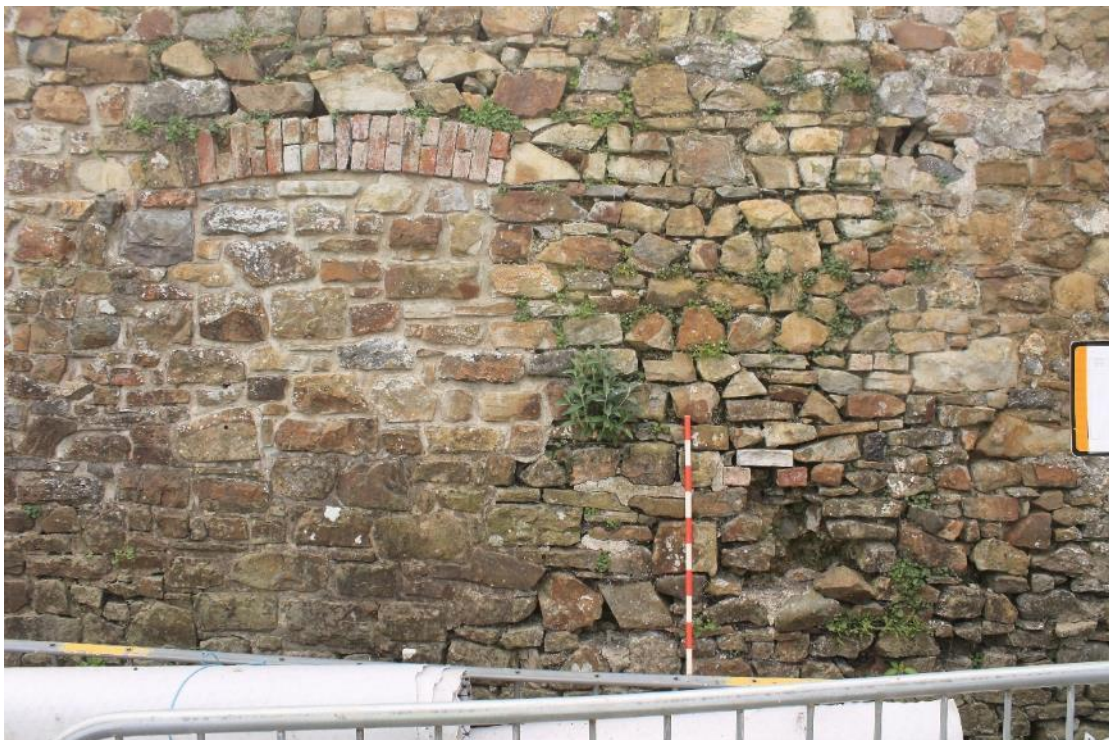
Photo 8: View SSE showing detail of the standing foundry building, including general building style and a blocked window. 1m scale.
