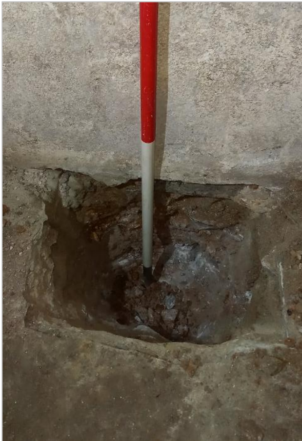
Photo 8: Exposed wall footings within TP02, No. 5 Castle Terrace. Looking east, 1m scale
