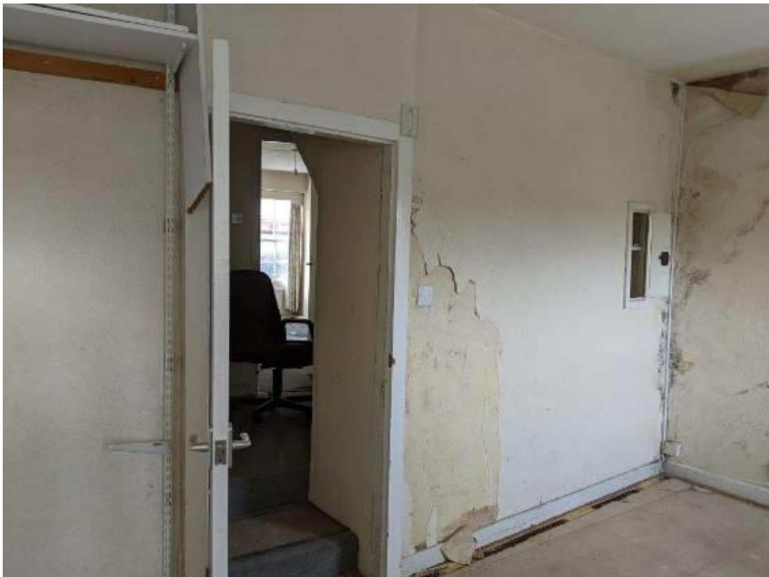
Photo 4: The medieval wall at first floor level identified in No 6 Castle Terrace, with small original opening (now a cupboard) to the right (see Photo 5).
