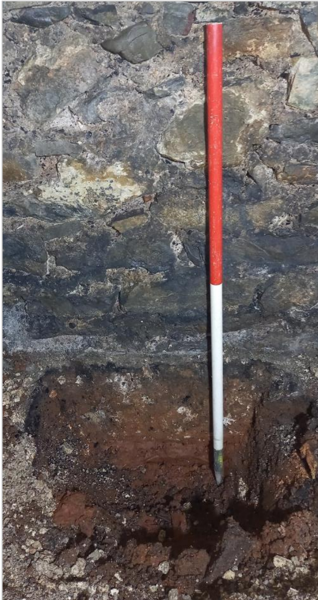
Photo 12: Wall footings exposed in TP04, below the basement in No. 7 Northgate Street. Note the visible coal 'scar' at floor level and continuing up the wall. Looking north, 1m scale
