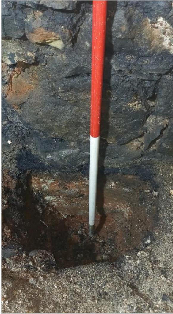
Photo 13: Wall footings exposed in TP05, below the basement in No. 7 Northgate Street. Note the visible coal 'scar' at floor level.
