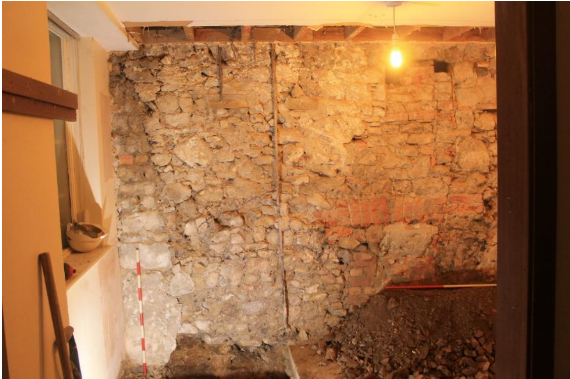
Photo 27: West facing shot showing the current wall above TP09 (visible bottom left). Note the segment of regularly coursed walling on the left and brick-headed fireplace to the right. 1m scales.
