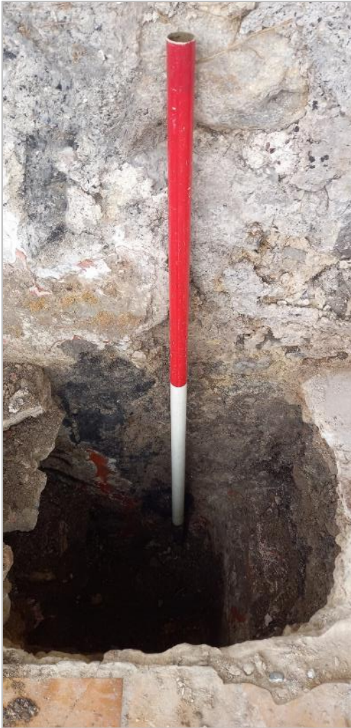
Photo 9 (left): TP03 showing below-ground, rendered footings of the rear (north facing) of No. 4 Castle Terrace (Wall {001}). Wall {002} is visible to the right. Looking south, 1m scale. Photo 10 (middle): Close-up of TP03 showing continuity of render on Walls {001} and {002}. Photo 11 (right): Modern artefacts recovered from TP03. 0.5m scale.
