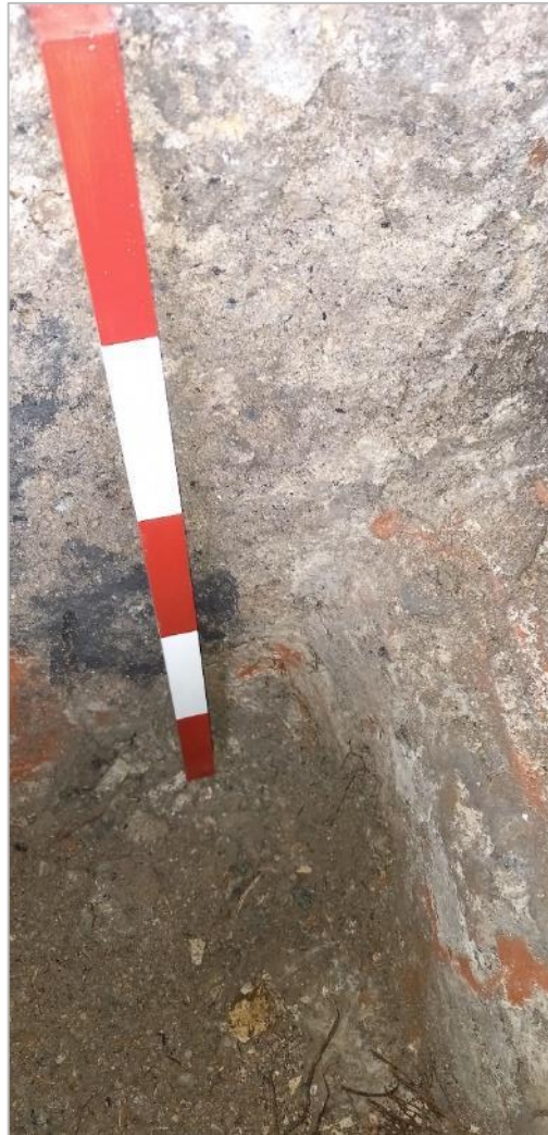
Photo 9 (left): TP03 showing below-ground, rendered footings of the rear (north facing) of No. 4 Castle Terrace (Wall {001}). Wall {002} is visible to the right. Looking south, 1m scale. Photo 10 (middle): Close-up of TP03 showing continuity of render on Walls {001} and {002}. Photo 11 (right): Modern artefacts recovered from TP03. 0.5m scale.
