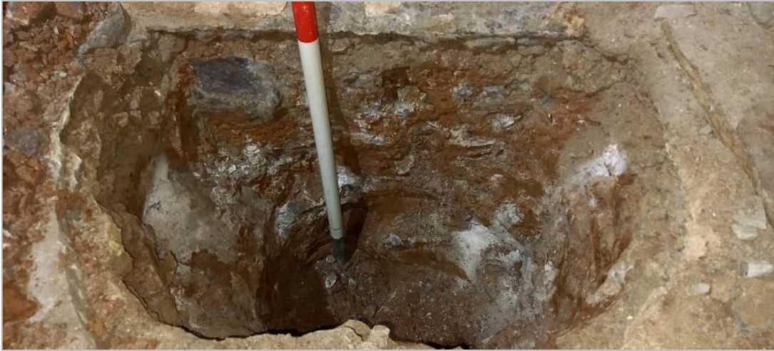
Photo 7: Exposed wall footings within TP01, inside No. 5 Castle Terrace. Looking east, 1m scale
