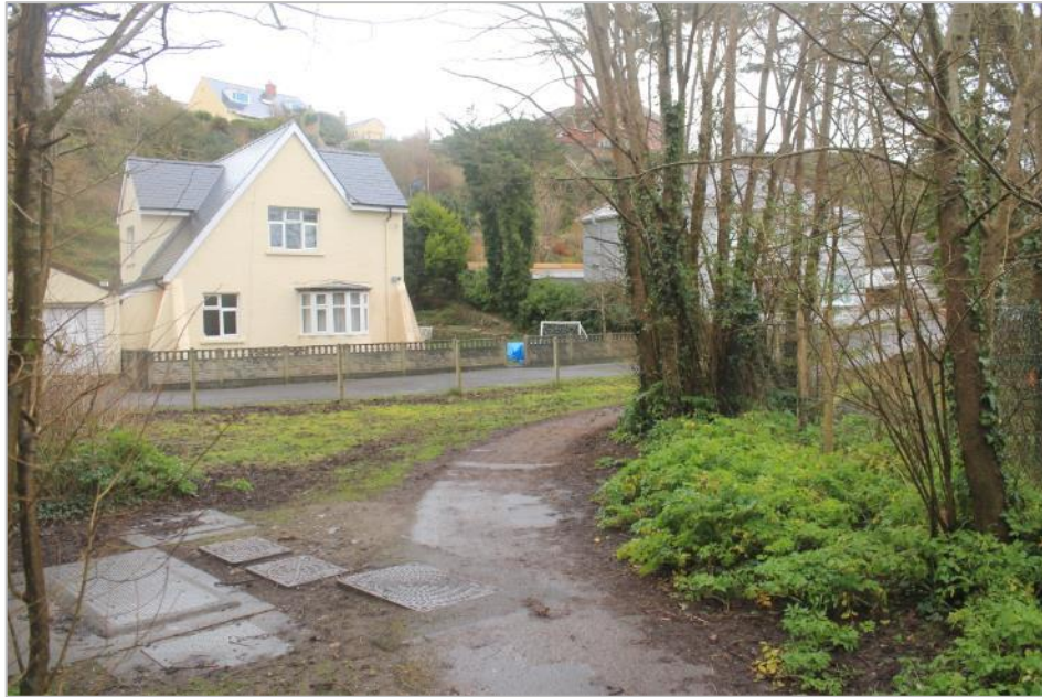
Photo 4: View east showing the access hatches to the culvert at the base of the southern side of the railway embankment.
