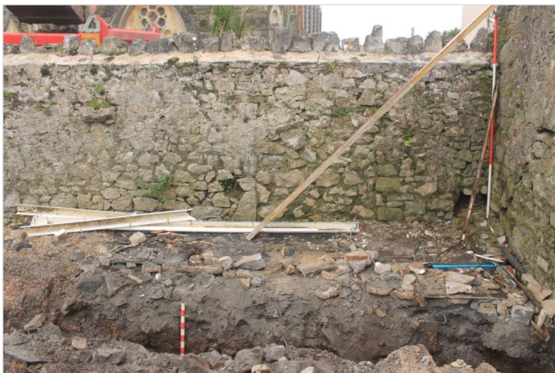
Photo 17: View southwest, showing detail of the interior of the Grade II listed wall, with blocked opening evident, including excavated foundation trench in the foreground. 2m & 0.5m scales.
