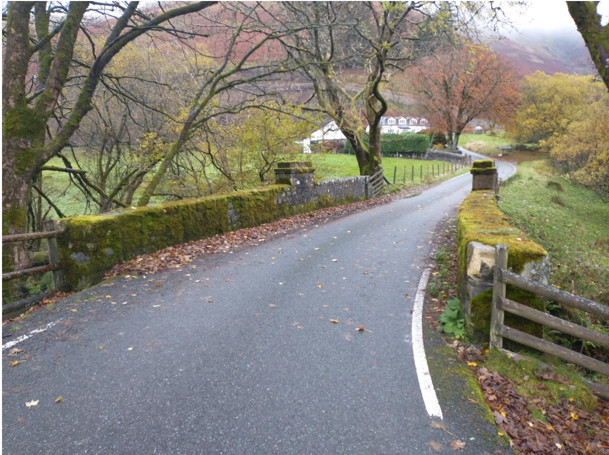
Figure 2: PRN 21759 Bont Blaen Bridge – Reported as there was some damage done to the bridge by a passing lorry. (Shown here as exposed limestone on the righthand side of the bridge – Photo courtesy of R. Kemp)
