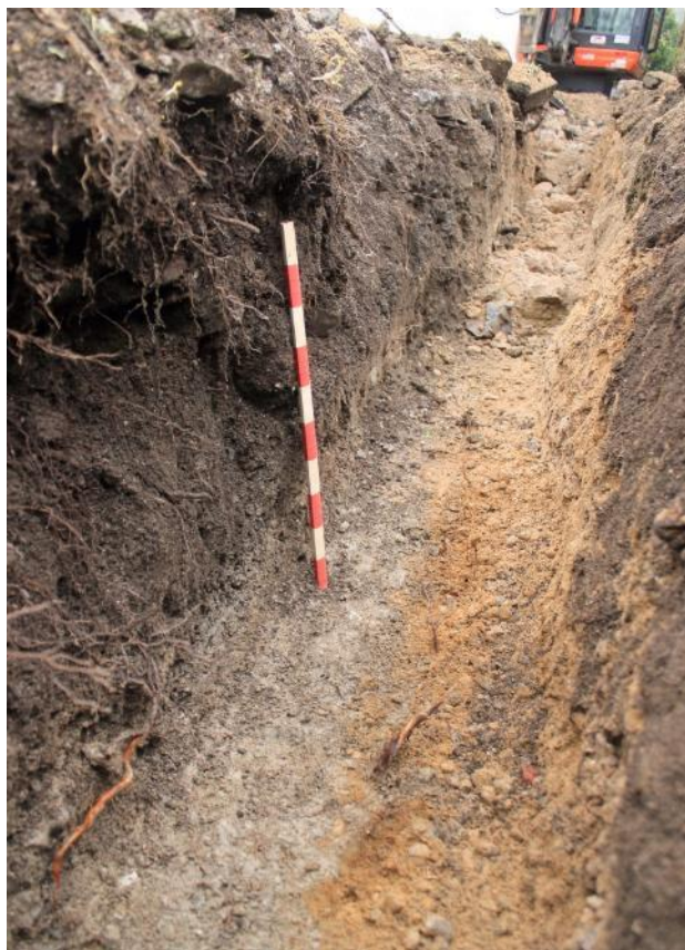
Photo 11: Potential subsoil deposit (005) on the left, cut by the sewer pipe trench [004] on the right, represented by the orange infill material. 0.5m scale.
