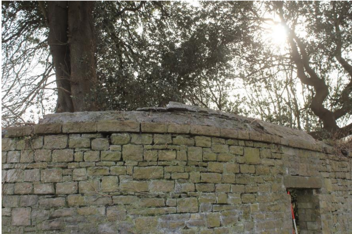
Photo 14: Southeast facing showing detail of the damaged coping on the northwest corner.
