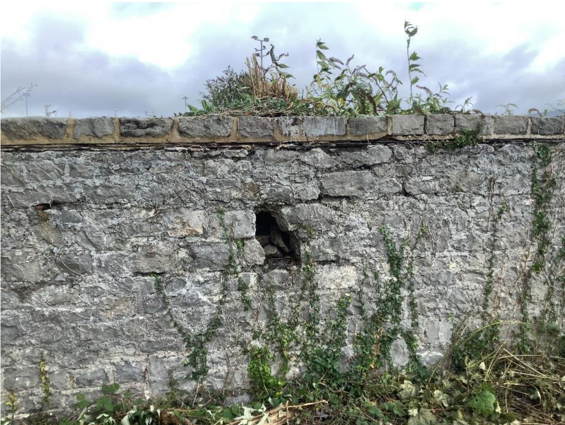
Photo 20: North facing shot showing the hole in the wall, with protruding metal bar to the left.
