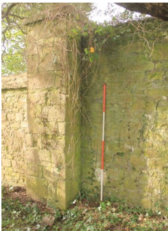
Photo 16: Southwest facing shot showing the butt joint between the corner wall and the pillar, visible to the interior. 2m scale.
