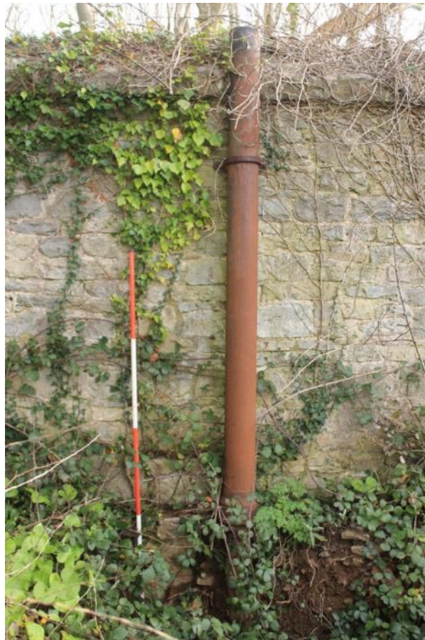
Photo 6: East facing shot of the attached iron stench pipe, with exposed foundations adjacent. 2m scale.
