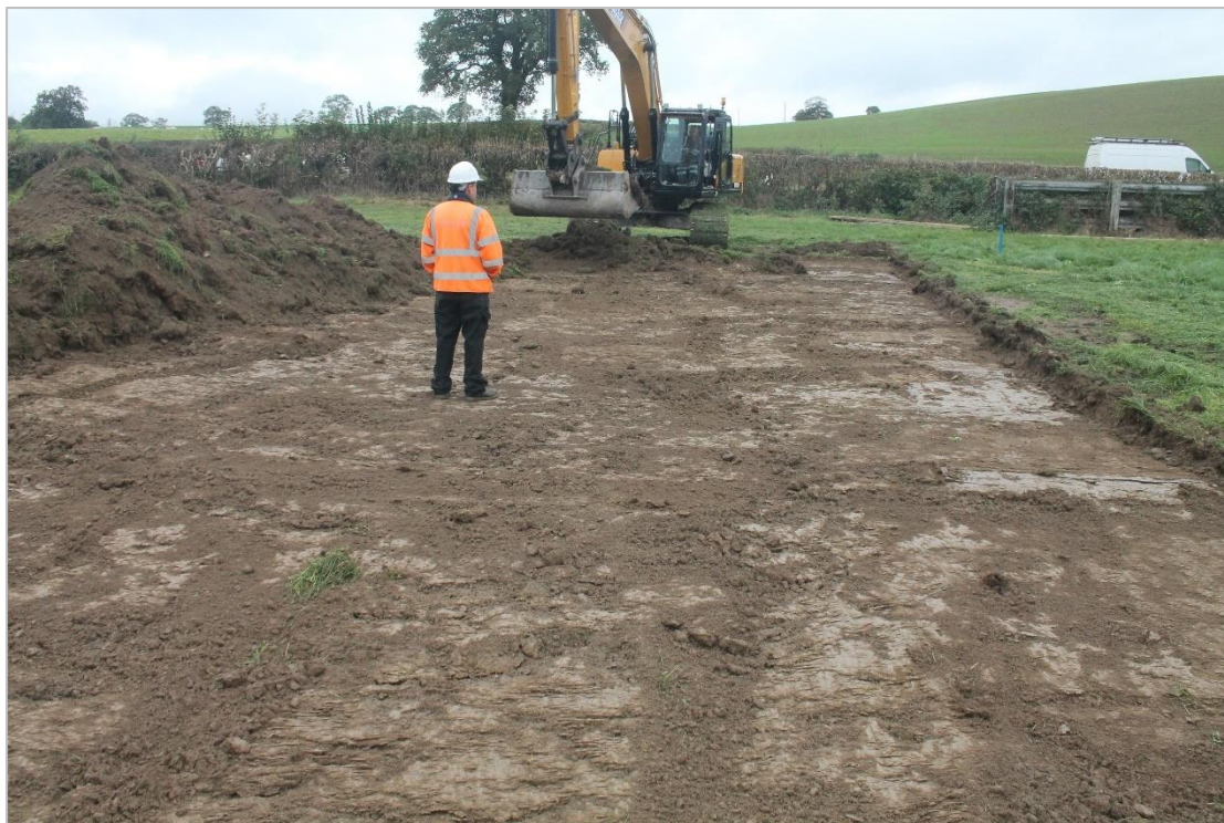
Photo 1: Topsoil stripping the compound area. View north.
