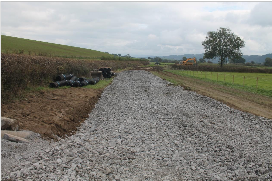
Photo 4: A section of track excavated and infilled with stone.
