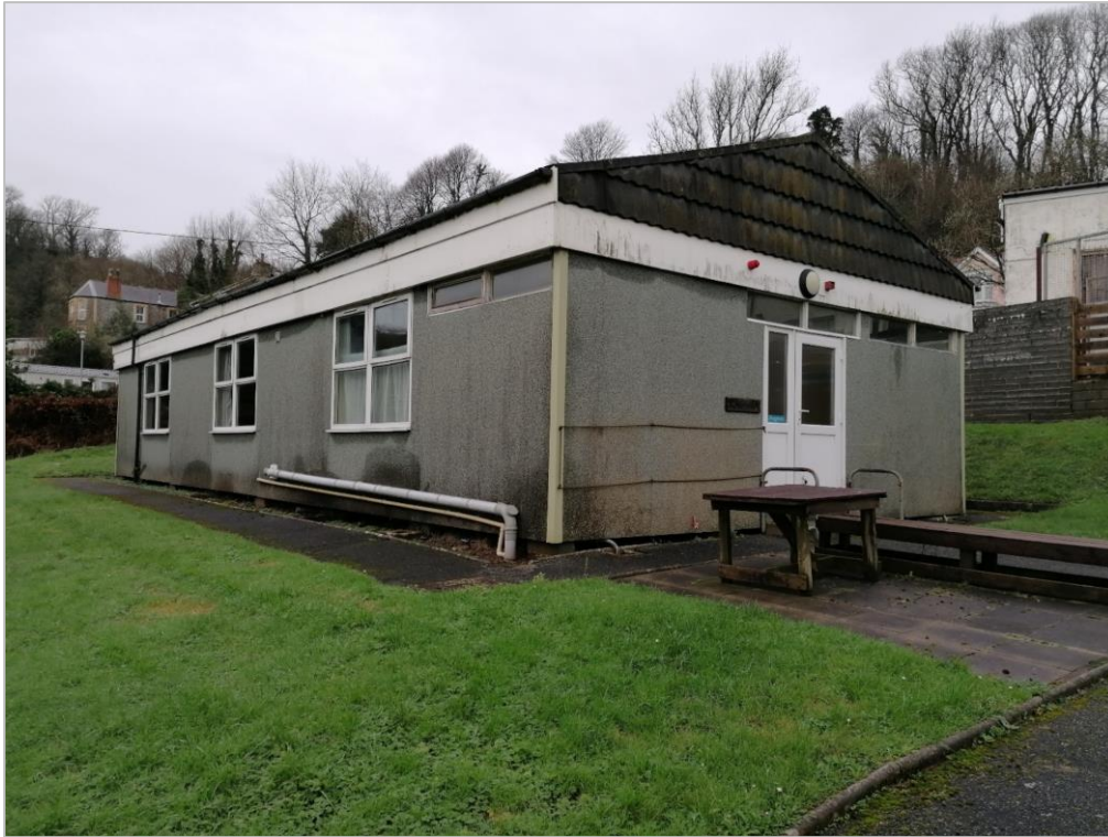
Photo 4: One of the former military blocks now being used by the Outdoor Education Centre. The dimensions and door location match the early photographs of the site, but the roof cladding, windows and external render appear to be later alterations.
