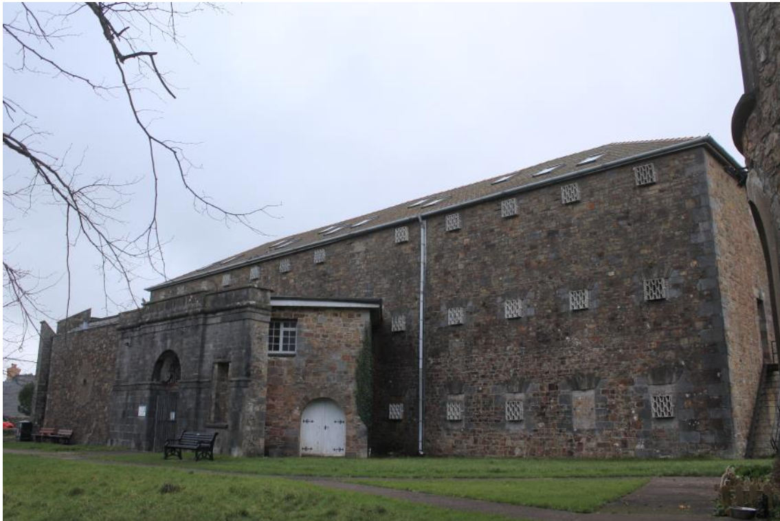
Figure 75: The current southern face of the building, showing the 1960s additions between the entrance and the main building, and the flanking walling to the west.
