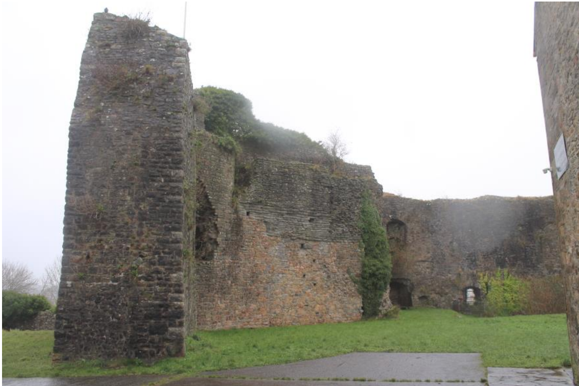
Figure 35: View east of the north curtain wall. The stonework on the end face dates to post-gaol restoration, the curtain wall east of the north tower is visible behind, showing the two phases of stonework.
