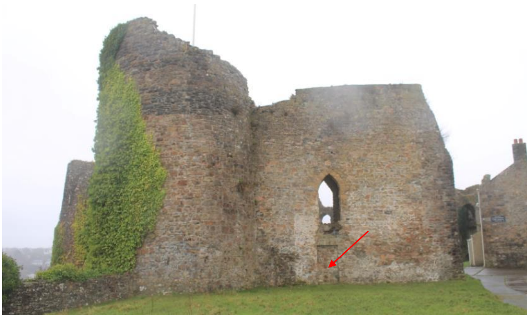
Figure 34: The external face of the north curtain wall. The blocked gaol-era door is marked in red, with the 1 st floor access above.
