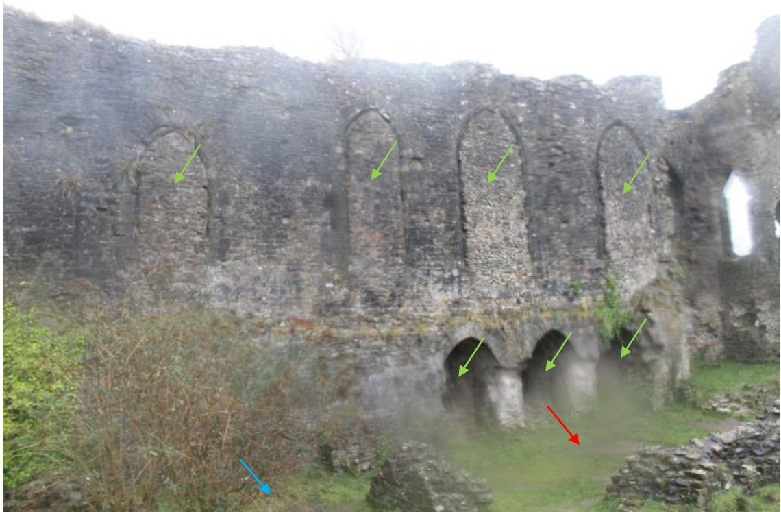
Figure 23: The East Range, interior view. The large 4 bay room with great chamber above is marked in red, a smaller room with a chamber above is in blue, with the latrine chamber (with offices above) just to the left of the small trees visible on the left. Window openings are marked in green.
