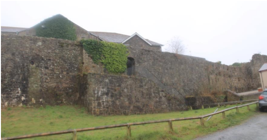
Figure 51: The inserted modern staircase in the curtain walling.
