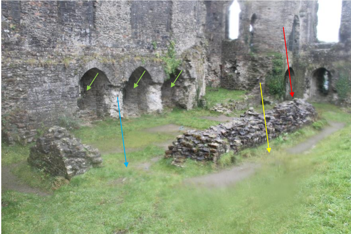
Figure 24: The East Range, interior view showing the 4-bay southern room (with Great Chamber above). The location of a possible spiral staircase is marked in red, the possible entrance in blue, windows in green and an external passage (represented by a low revetment wall to the grassed central area) in yellow.
