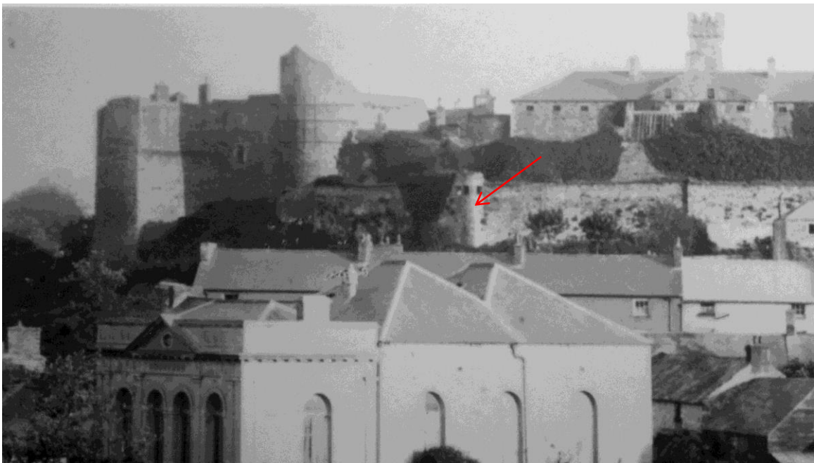
Figure 49: Photograph from 1935 (Haverfordwest Town Museum) showing the northern curtain wall and rounded turret in red, with openings visible in the upper levels.
