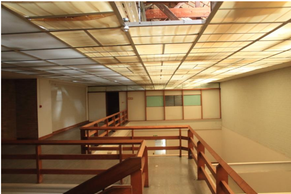
Figure 78: The interior at 1 st floor level, showing the modern mezzanine flooring and lowered ceiling.
