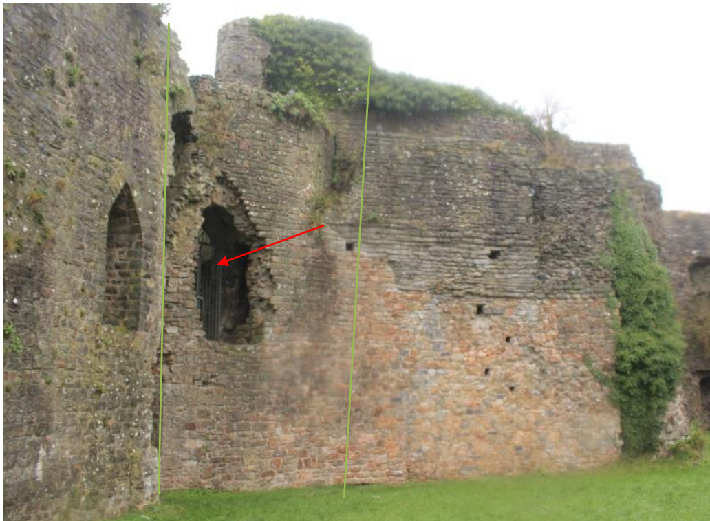
Figure 14: The internal face of the North tower, between the green lines. The original entrance to the first floor level is shown in red.
