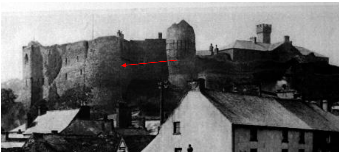
Figure 9: Photo of circa 1900 showing the keep as a more solid projecting bastion, with a upper line in keeping with the surrounding walling. (Haverfordwest Town Museum).
