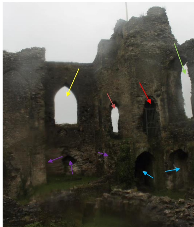
Figure 30: A view of the chapel from the west, unfortunately taken in poor weather conditions. Ground floor open windows are marked in blue, the left one being within an enclosed room, blocked windows are marked in purple. Chapel chancel east window is marked in yellow, the chancel south window in brown, nave south window in green. The Chapel spiral stair is marked in red.
