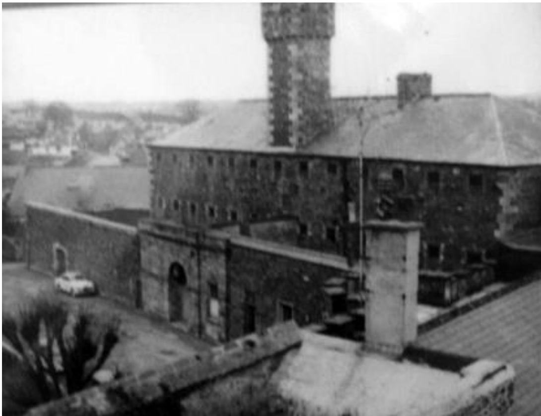
Figure 74: View from the roof of the Governor's House of the south face of the gaol building, also showing now-removed features such as the flanking walling to either side of the entrance, and the tall watchtower projecting from the roof. (Haverfordwest Town Museum).
