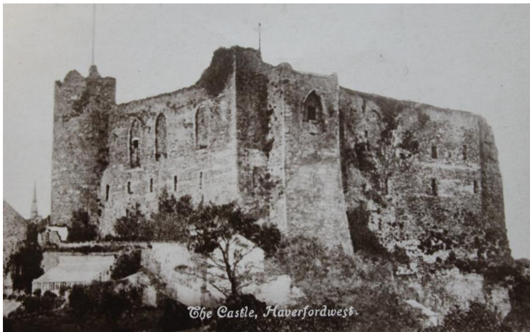
Figure 26: Undated photograph, showing the projecting chapel in the central square turret, with the South Range to the left. At this point the upper windows were blocked. (Haverfordwest Town Museum).
