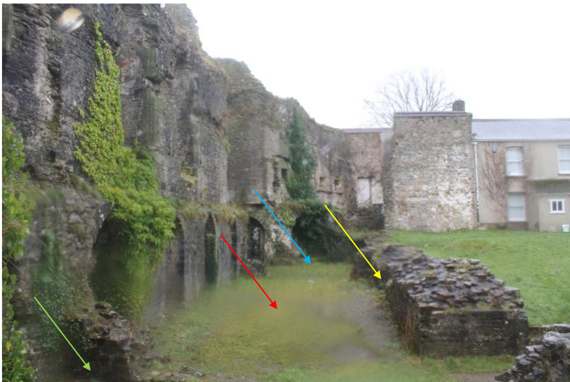
Figure 28: The South Range viewed from the east. The central 4-bay room is marked in red (hall at 1 st floor) with the fireplace set in a curve in the wall in yellow, the west room in blue, the east room in green.
