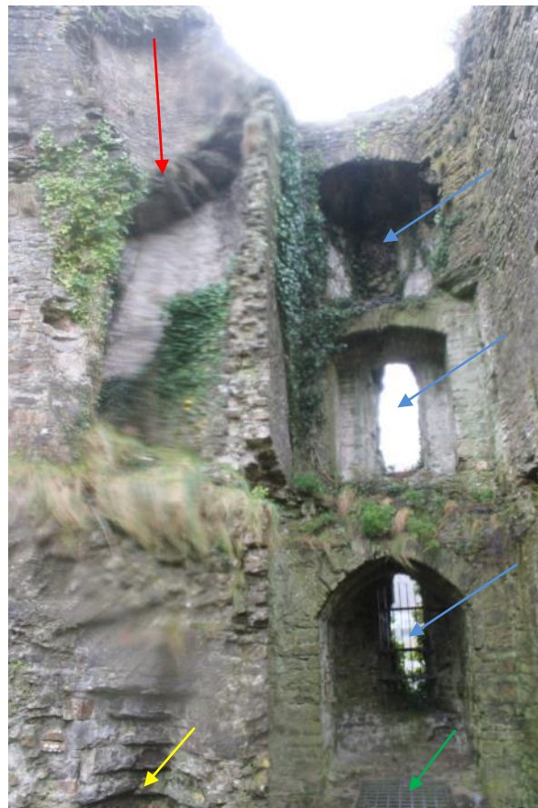
Figure 19: Interior of the Southwest tower, looking south. Features of note include the spiral stair in red, windows in blue, basement shaft in green and the stair to garden/queens arbour in yellow.
