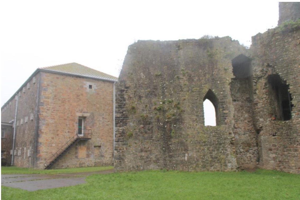
Figure 36: The internal face of the north curtain wall, with the gaol building to the left. The 1 st floor opening is visible, with the internal recess visible on the right. The opening on the right is part of the North Tower.
