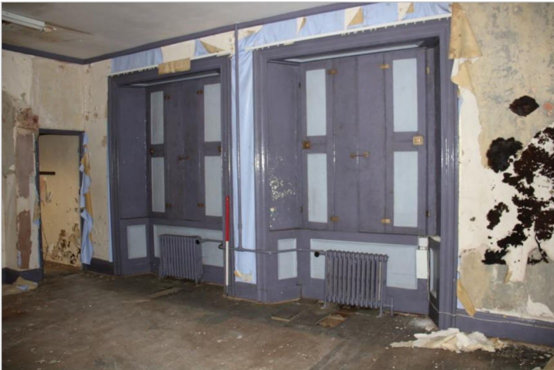
Photo 30: Recessed shuttered windows in north wall of Common Room.
