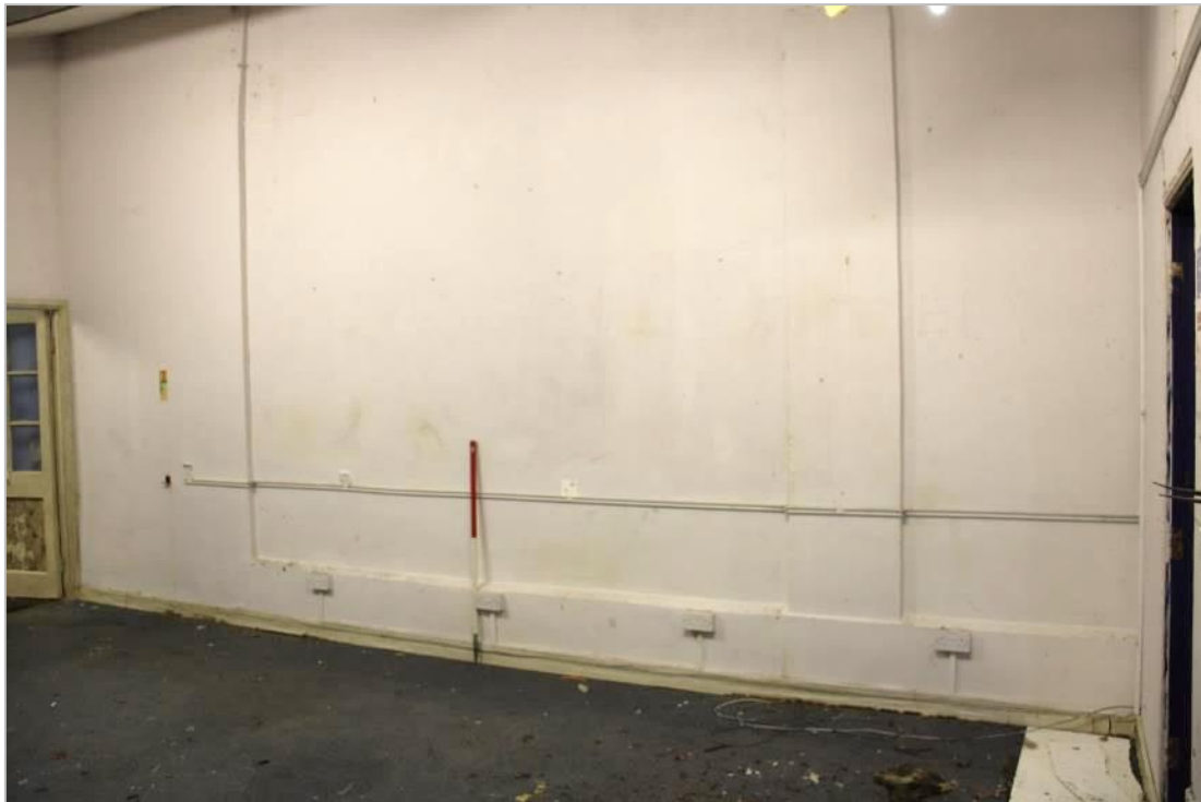
Photo 32: North wall of IT Room, once an outside wall. Pilaster on the right possibly marks the boundary between Phase 1 and Phase 2.
