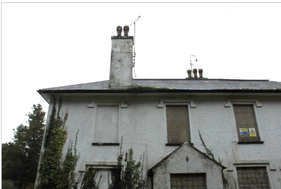
Photo 3: North elevation showing tall chimney stack with blind window below.
