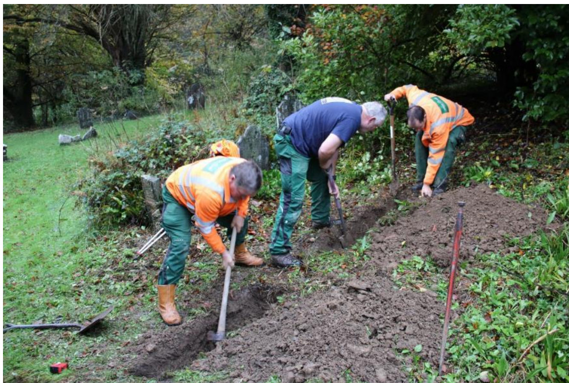
Photograph 1: Hand excavation of new pipe trench. View roughly north.
