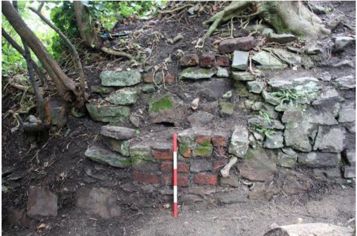
Photo 7: Bricked-up opening in north wall of building B (1m scale)
