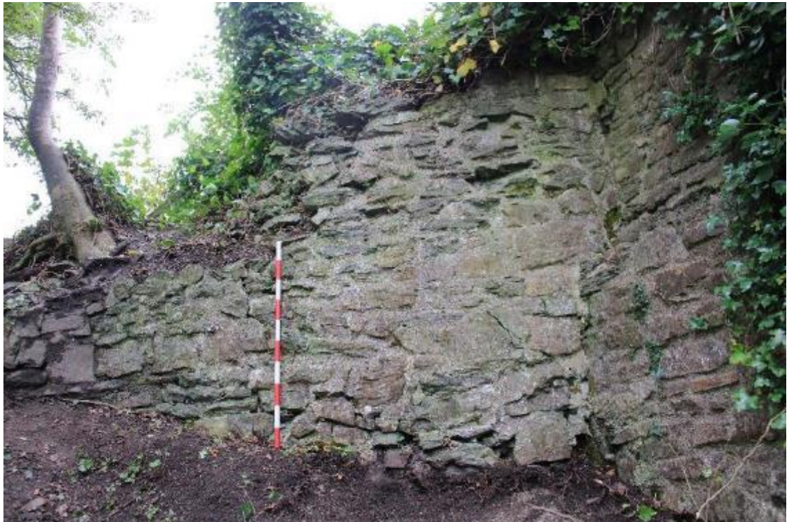
Photo 6: East end of north wall of building B butting up against Castle wall (1m scale)
