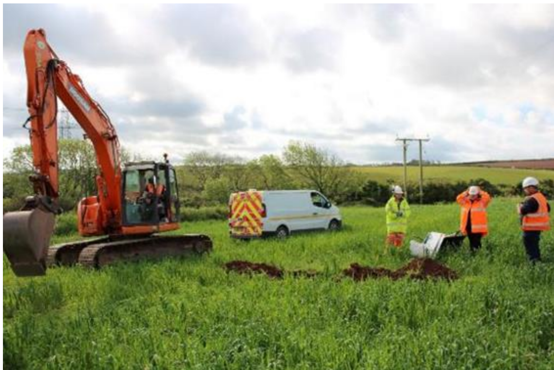
Photograph 1: Excavation of geotechnical trial pits at location of proposed substation
