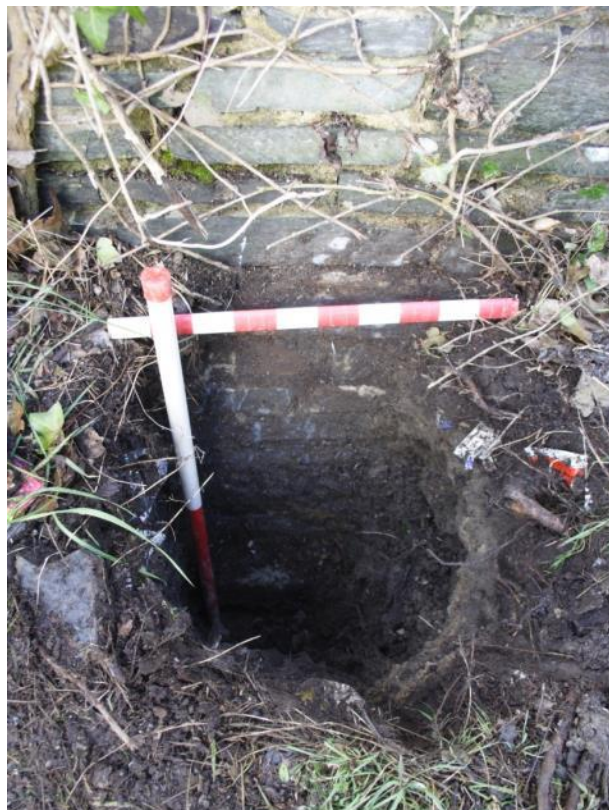
Photo 5: Test pit (Meek 2015) excavated adjacent to wall on south side of The Strand, showing foundations of 1970s built wall viewing north
