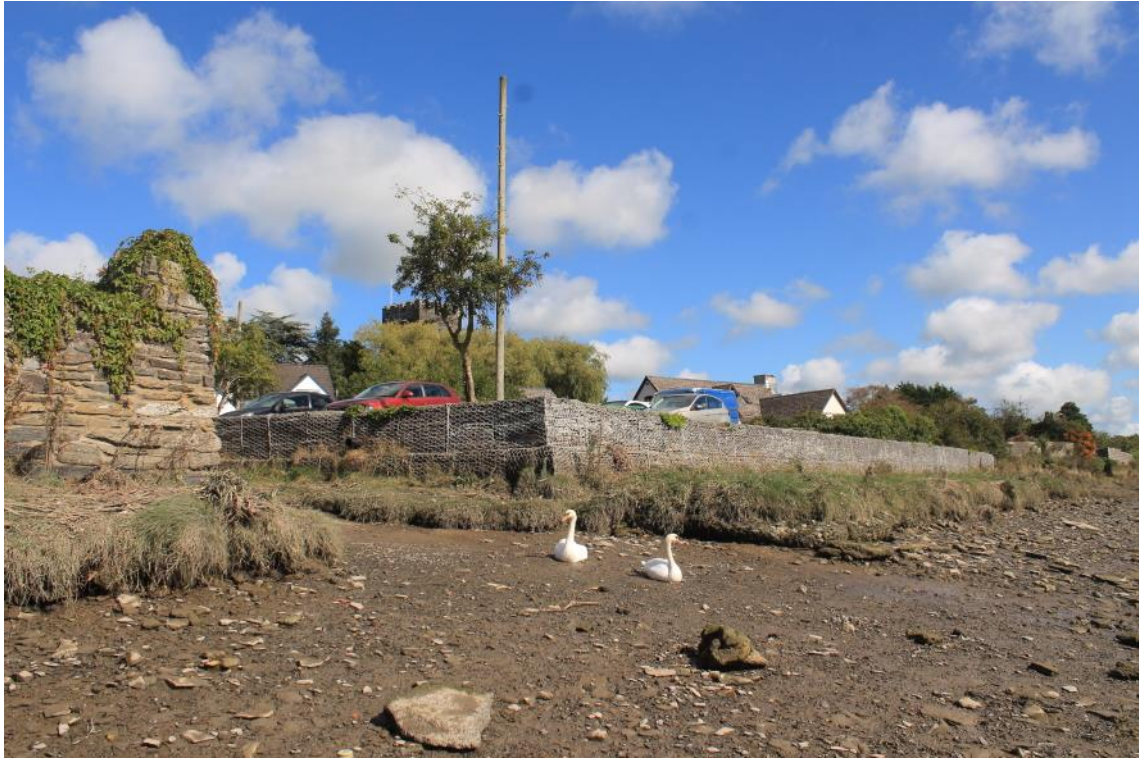
Photo 22: The stone-filled gabions around the Gloster Row car park.
