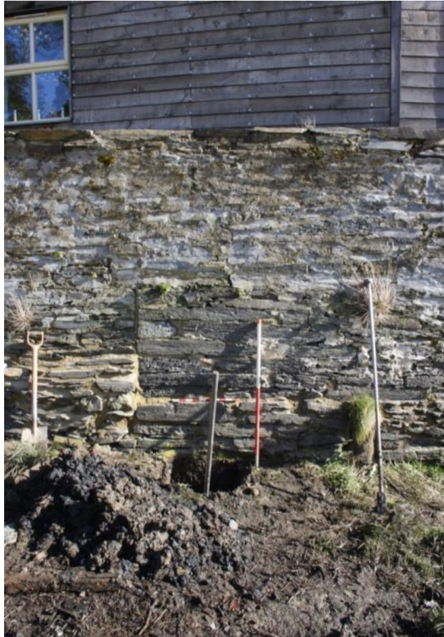
Photo 6: Test pit (Meek 2015) excavated adjacent to Cardigan Bathroom Centre wharf, showing different phases in construction
