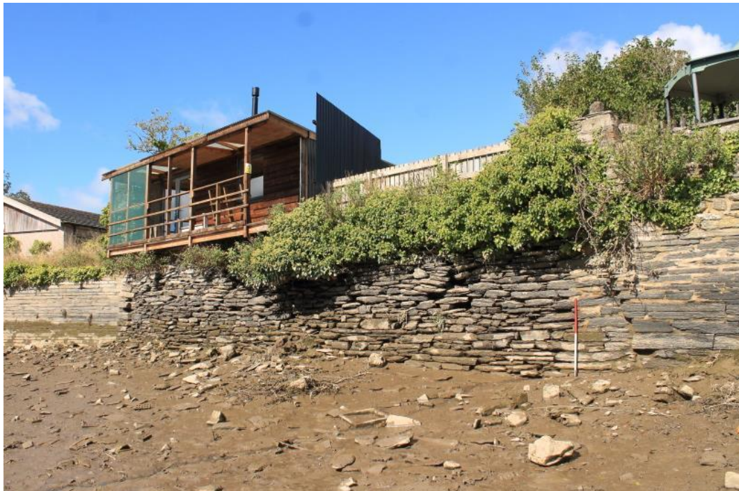
Photo 19: Closer view of the mixed rough stone walling fronting the riverside to the west of the slipway. 1m scale.
