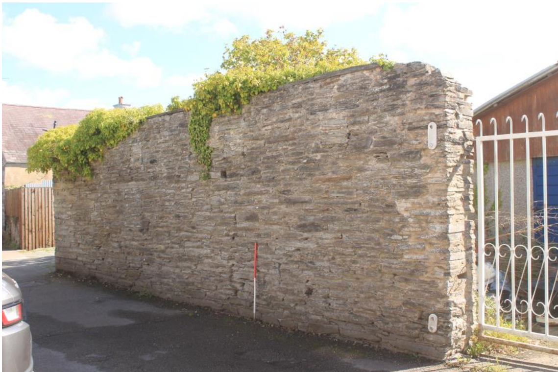
Photo 15: The northern wall of the Scout enclosure, to the east of the gateway, showing blocked openings. 1m scale.
