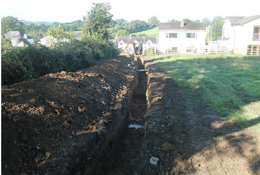
Photograph 8: View west after completion of cable-trench.
