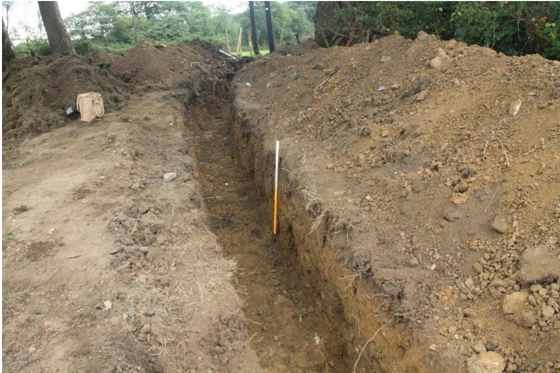
Photograph 5: View east showing 0.5m wide trench excavated along the centre of proposed trackway.
