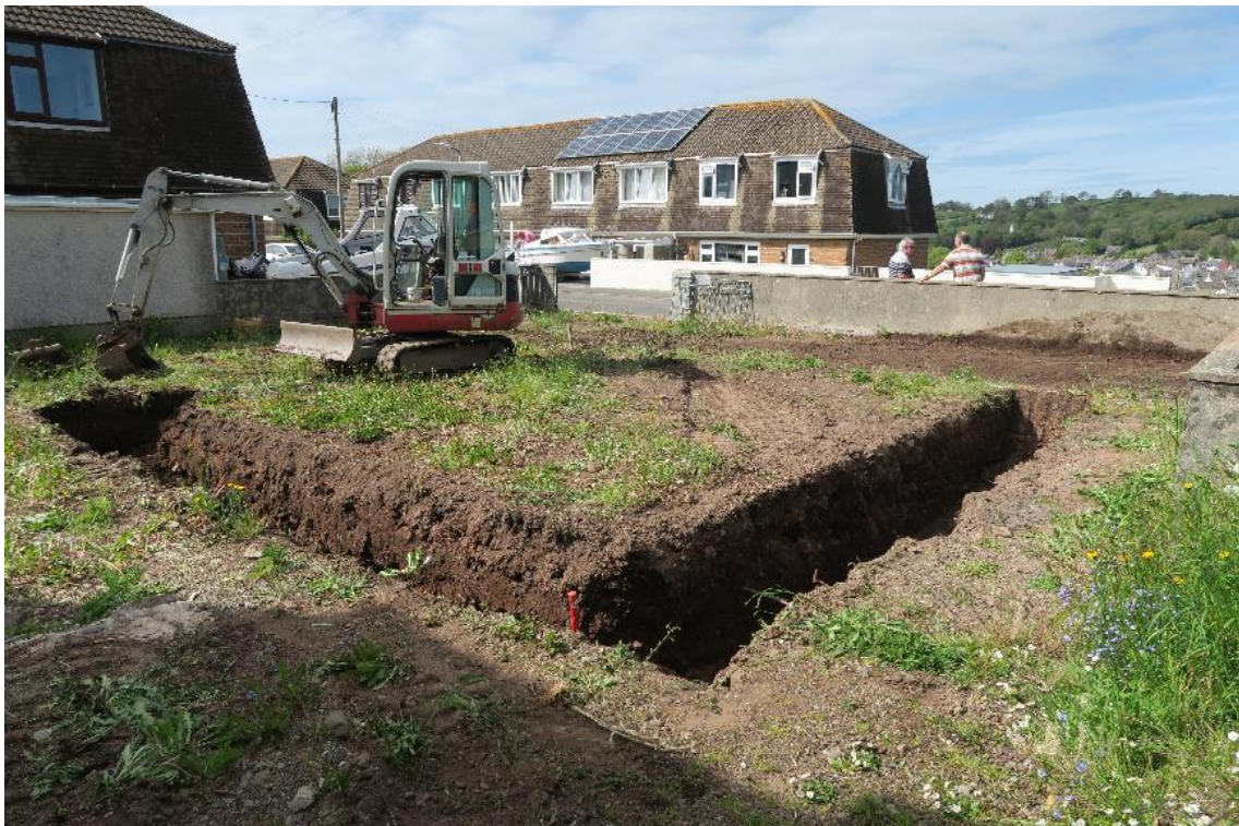
Photo 4: Looking north across site – showing excavated foundation trenches.
