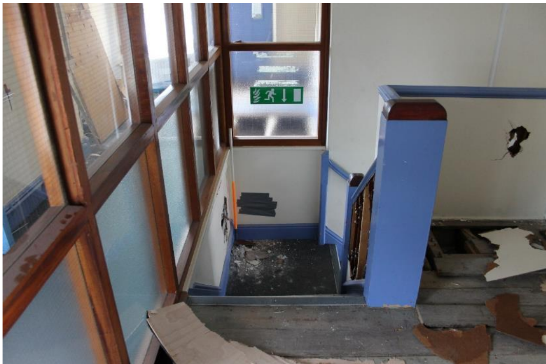
Photo 39: Reinforced glass and timber framed wall beside landing (blocked stairway right of 1m scale)
