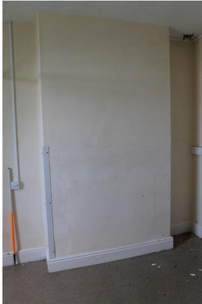
Photo 27: Chimney breast and probable blocked fireplace in a room at the southern end of the N-S corridor (1m scale)
