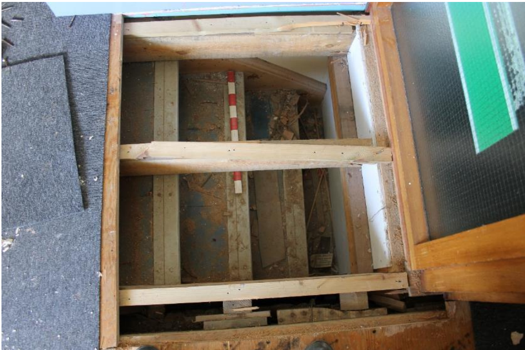
Photo 43: Lifted floorboards reveal blocked stairs leading to mid-landing (see photo 39)
