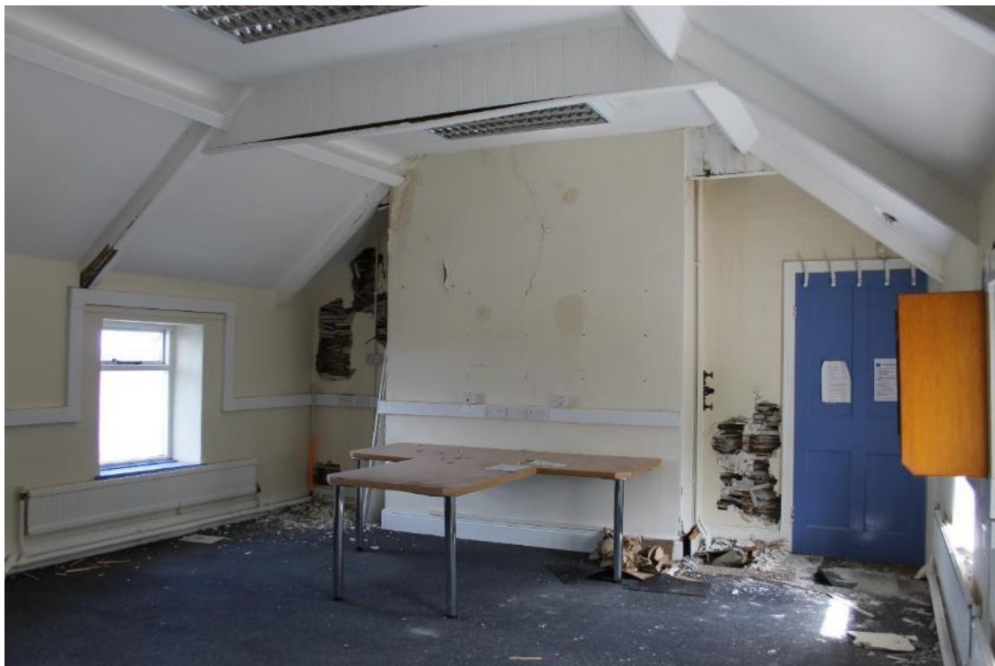
Photo 49: Chimney breast and blocked fireplace in large office at south end of building (1m scale)
