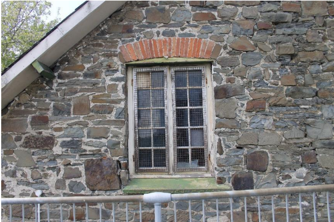
Photo 17: East facing elevation of rubble stone wall and window possibly associated with workhouse.
