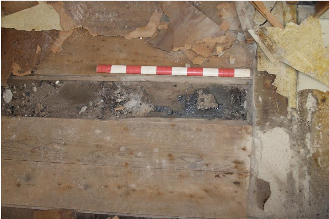
Photo 30: Lifted floorboard showing thin layer of bitumen beneath (0.5m scale).
