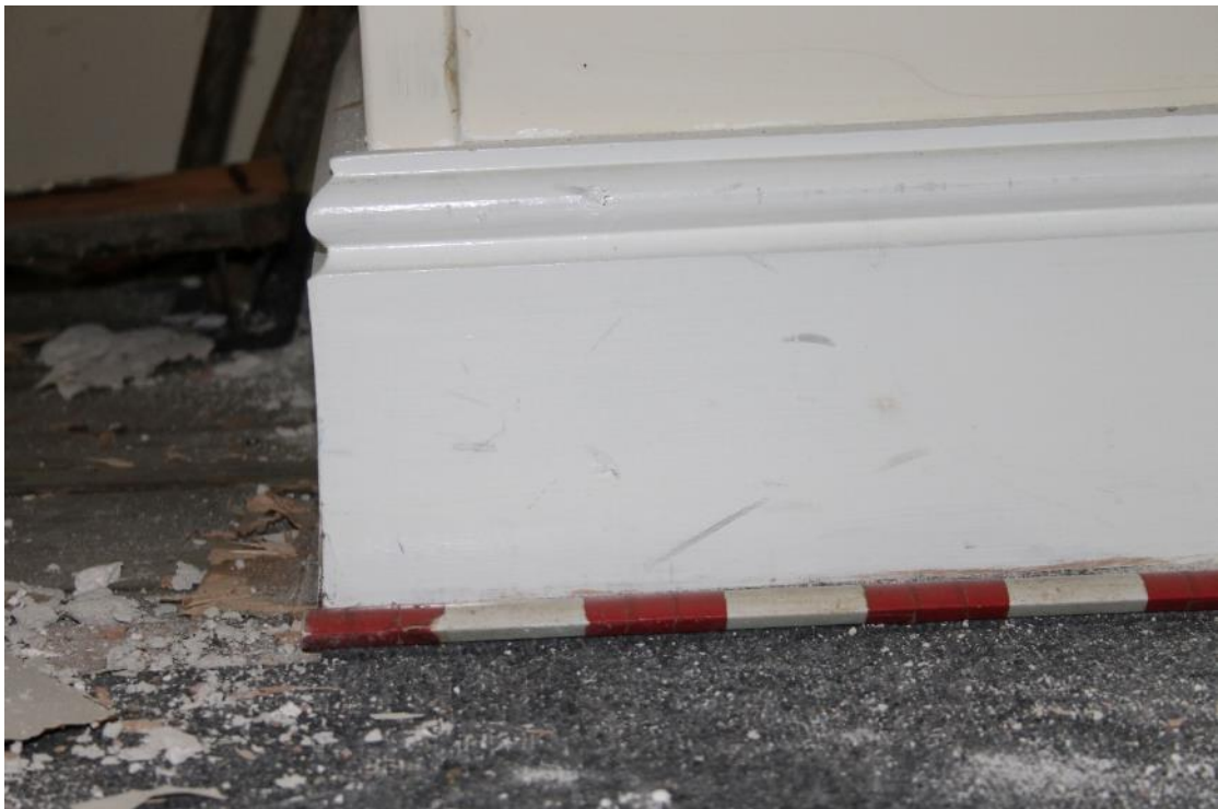
Photo 41: Typical (original) skirting board profile seen throughout building (0.5 scale)
