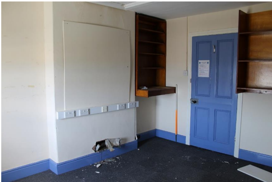
Photo 51: Blocked fireplace and four panelled door in office at north end of building (1m scale).
