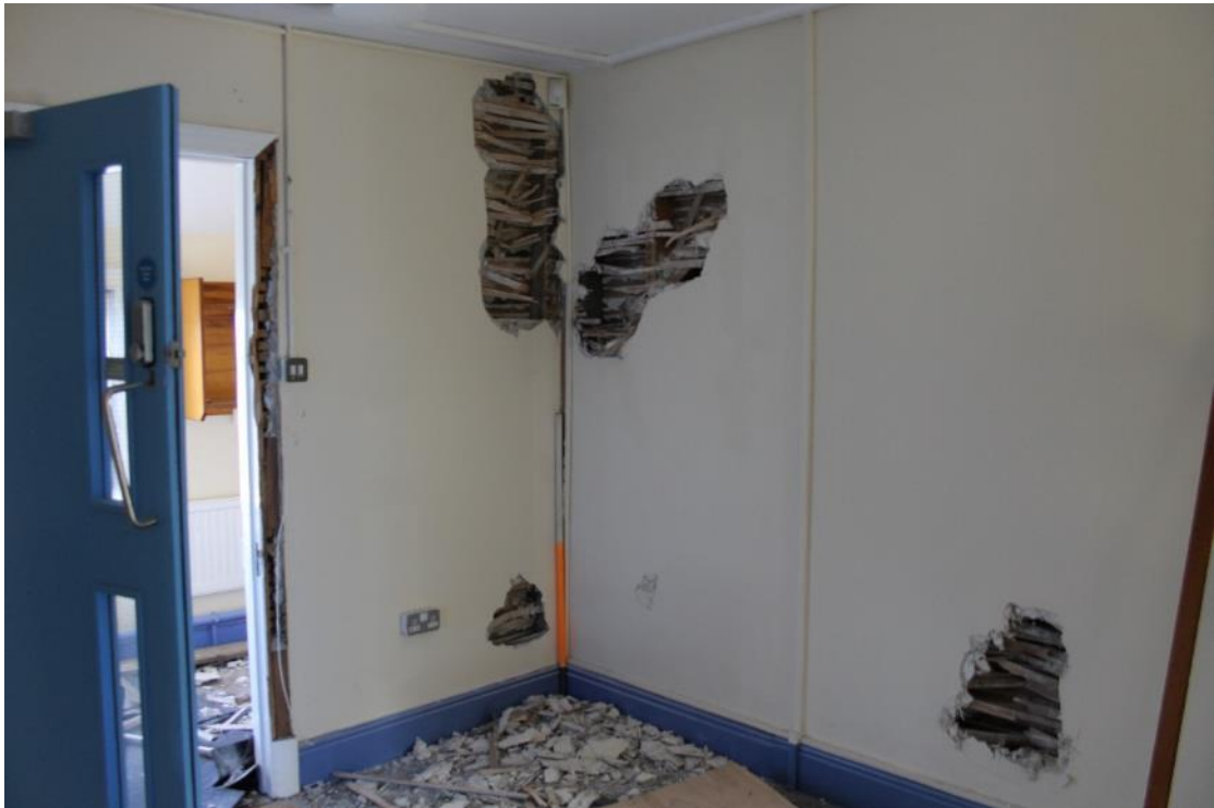
Photo 40: Lathe and plaster walls in landing (1m scale)
