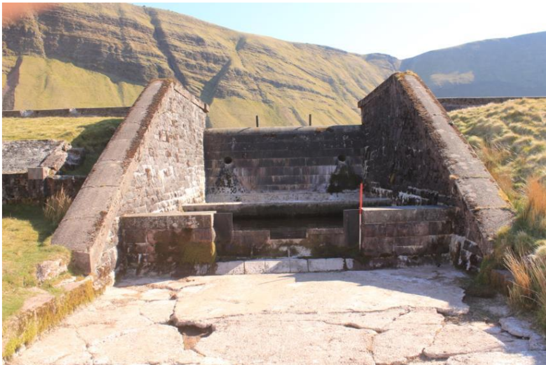
Photo 19: View looking SSW at the spillway, placed centrally along the reservoir dam wall.
