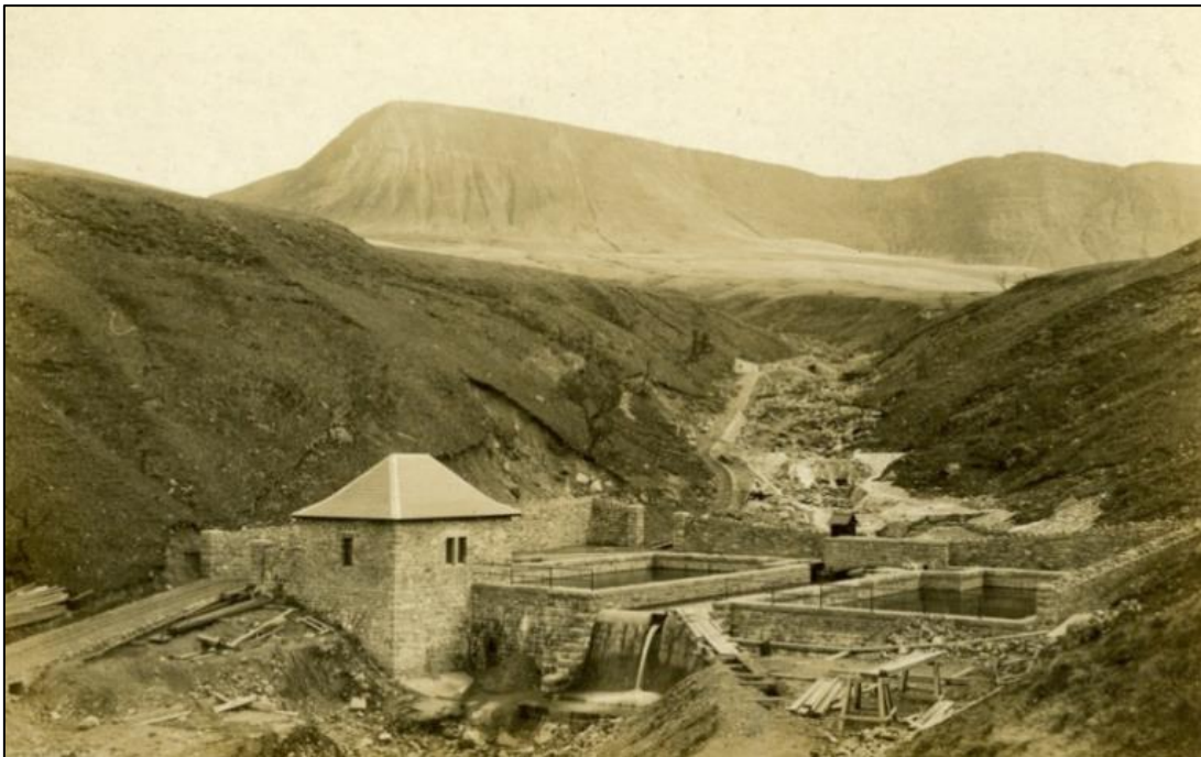
Photo 1: The Valve House and Filter Beds under construction. (Peter Davies Collection).
