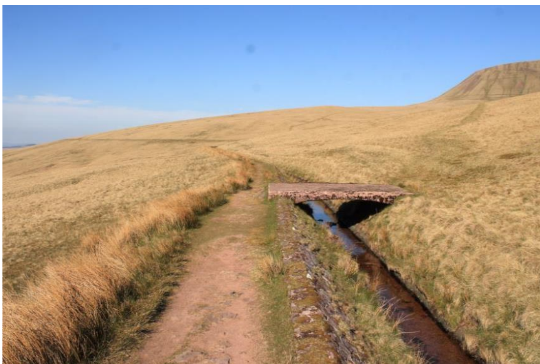
Photo 23: View north showing the catchwater (PRN 111185) feeding the reservoir from the northeast.
