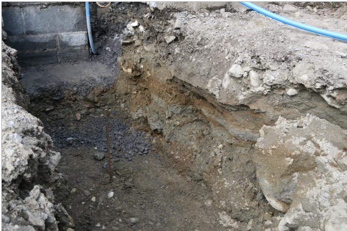
Photograph 6: Undisturbed river gravels, silts and pebbles on north side of site
