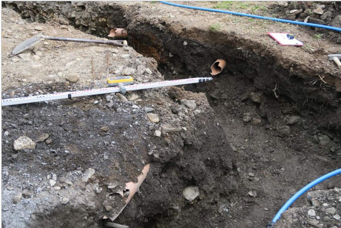
Photo 7: Plastic drainpipes unearthed during the trench excavation
