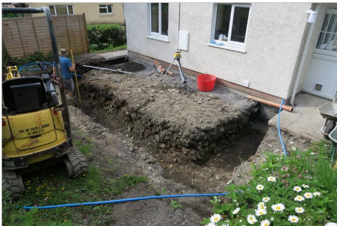
Photograph 3: Looking south at completed foundation trenches
