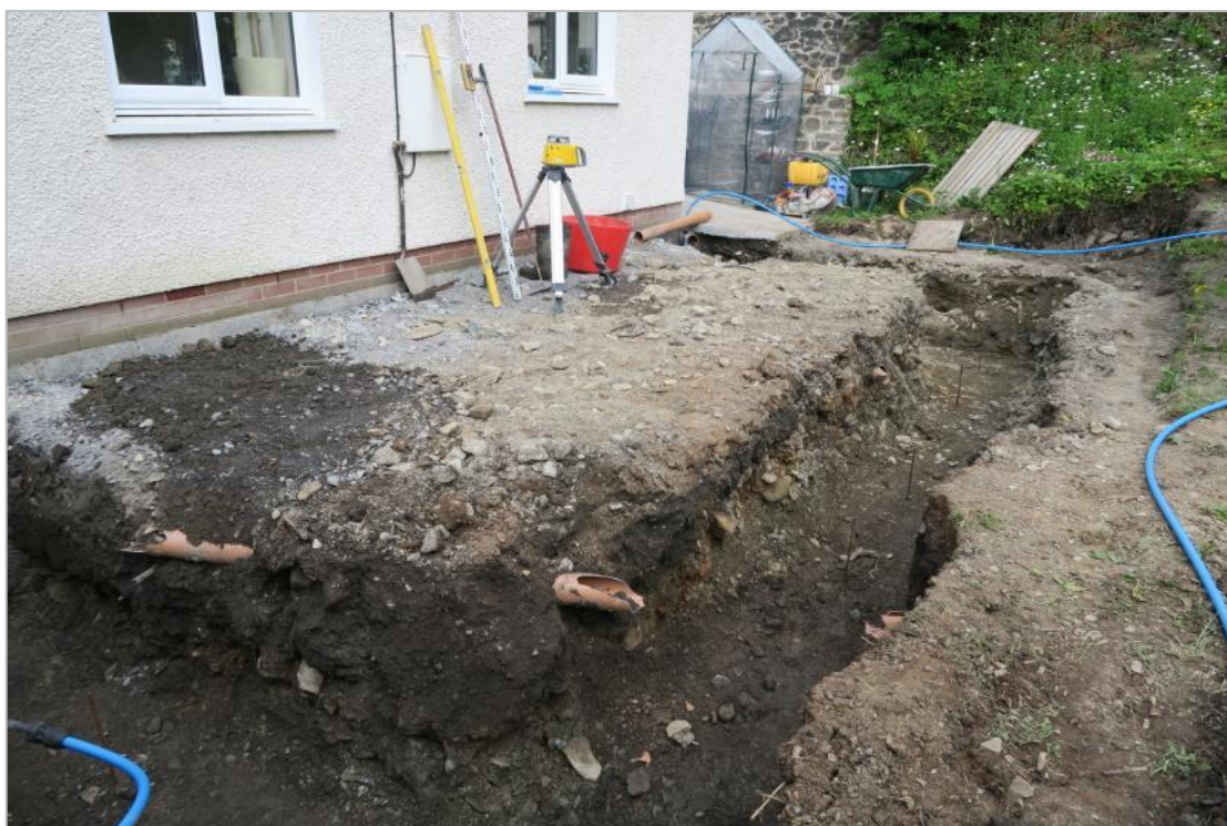
Photograph 4: Looking NW at completed foundation trenches
