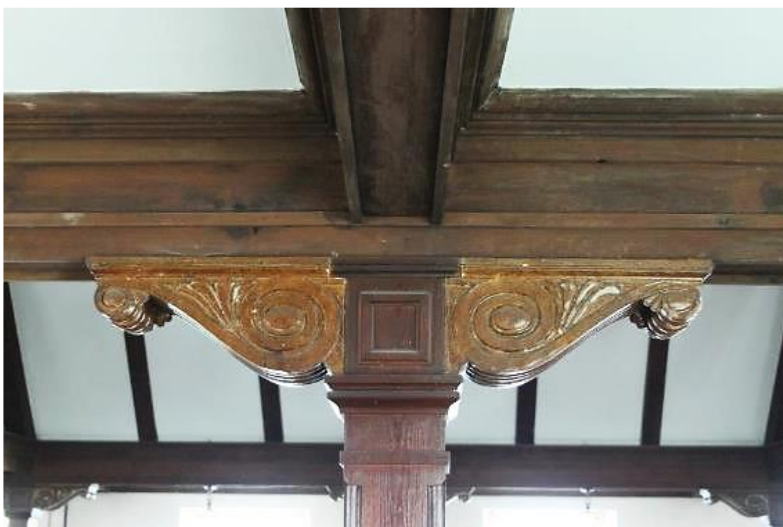
Photo 64: Detail of ornate console bracket under longitudinal beam
