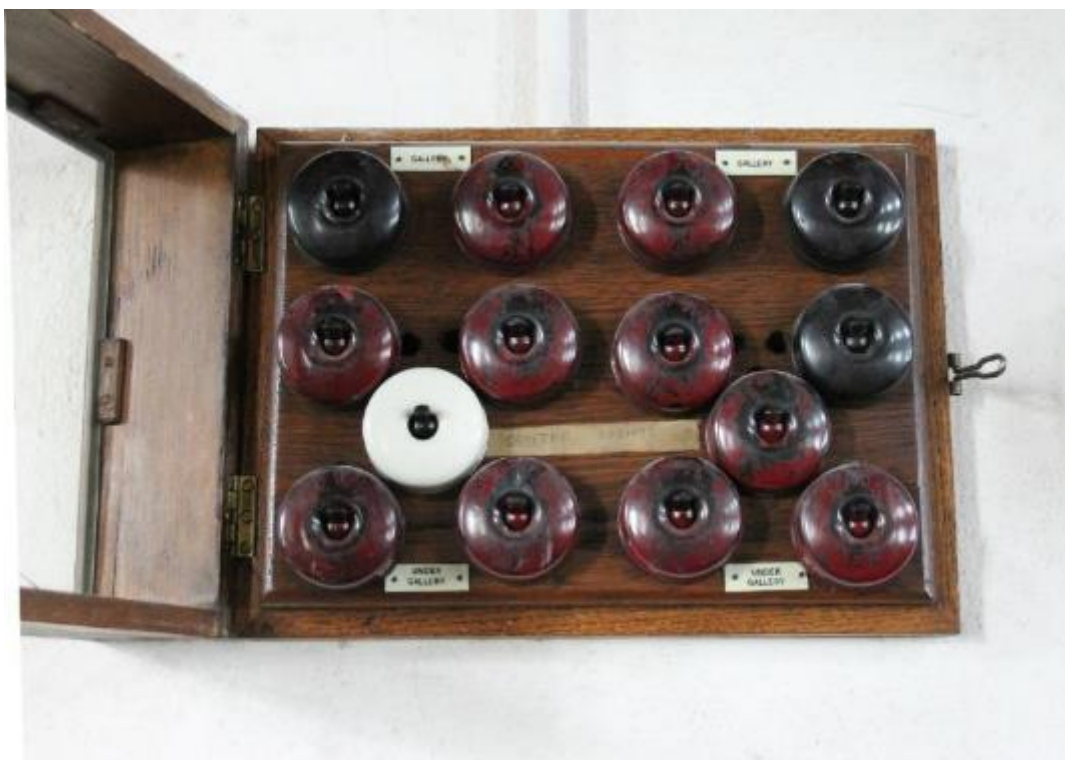
Photo 51: Set of bakelite swithes in north wall of chapel
