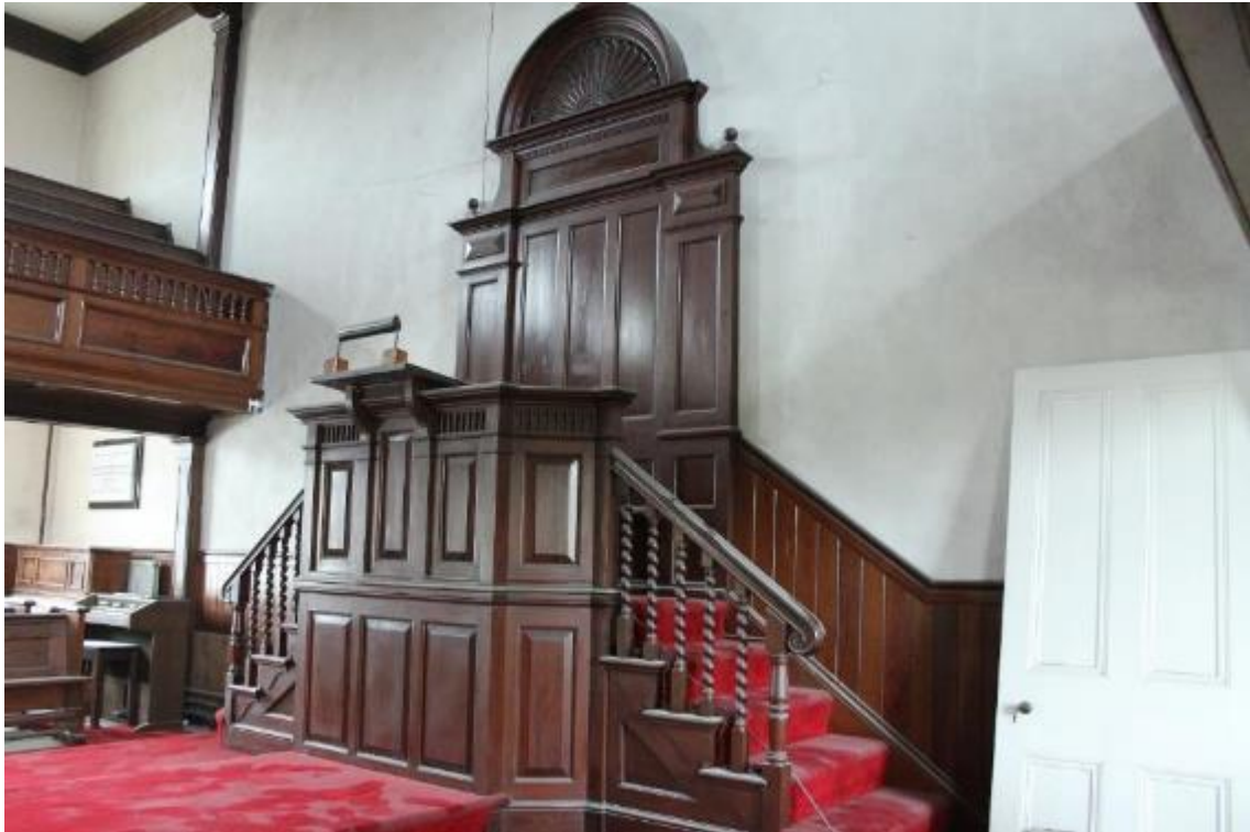
Photo 41: Oblique view of pulpit with twisted-baluster steps each side, panelled front with canted sides and ornate pulpit-back in mannered C17 classical style, with semi-circular top panel, carved in radiating shell pattern.
