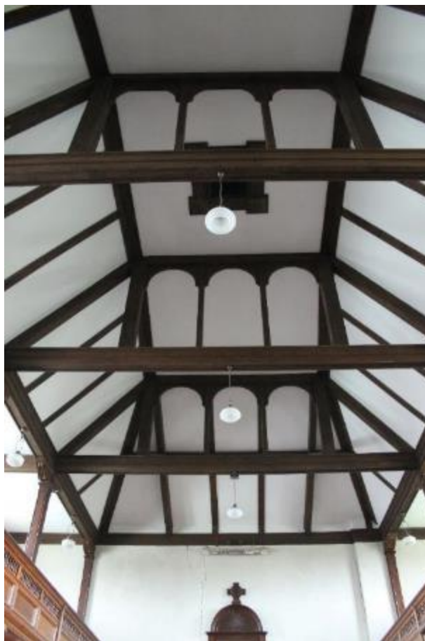
Photo 67: View south; tall, triple arcade above tie-beams.
