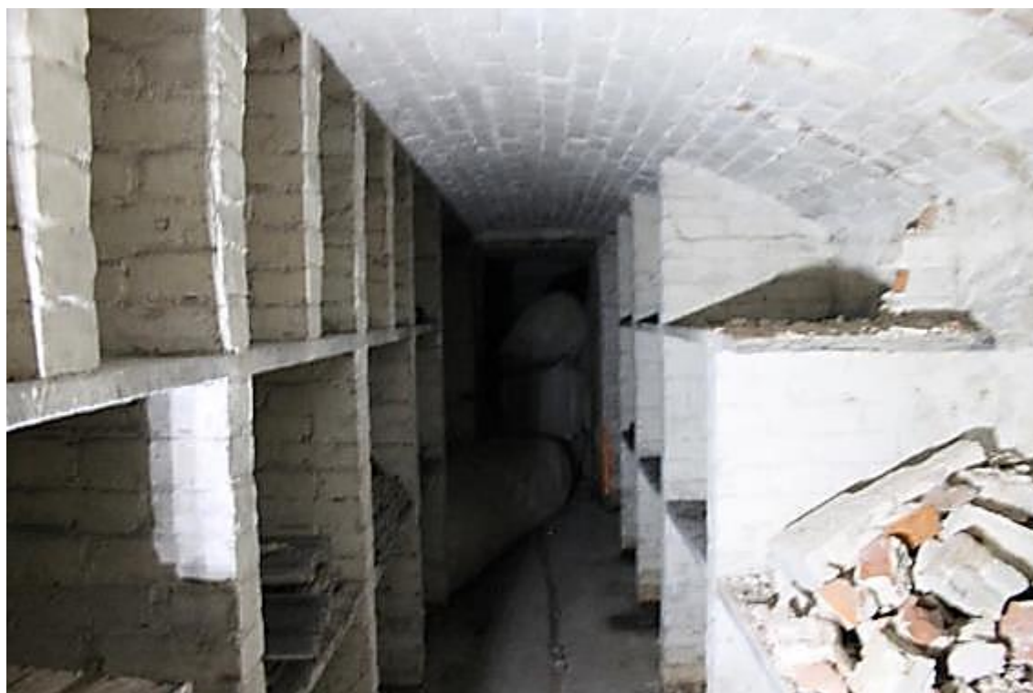
Photo 12: View south along wine cellar showing wine bins and brick vault.
