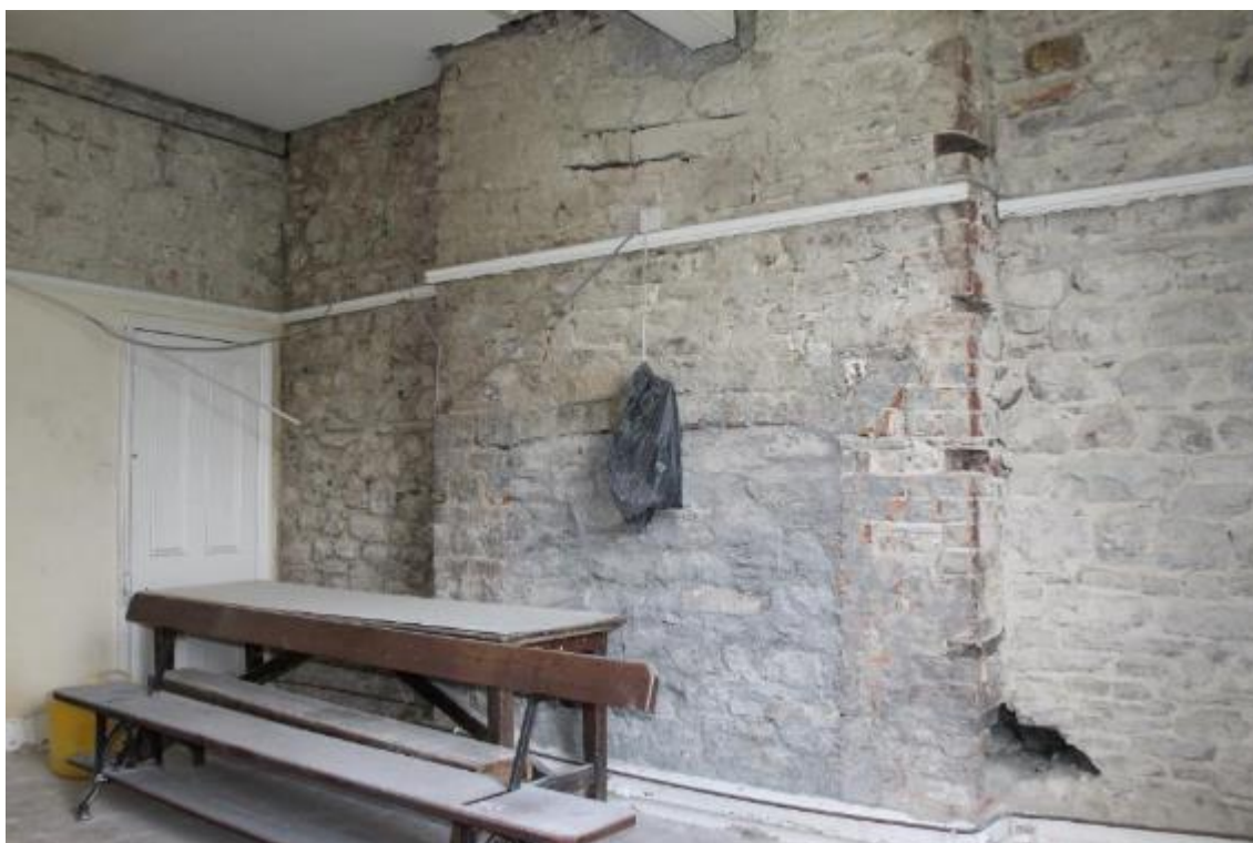
Photo 27: Blocked fireplace in south wall of kitchen.
