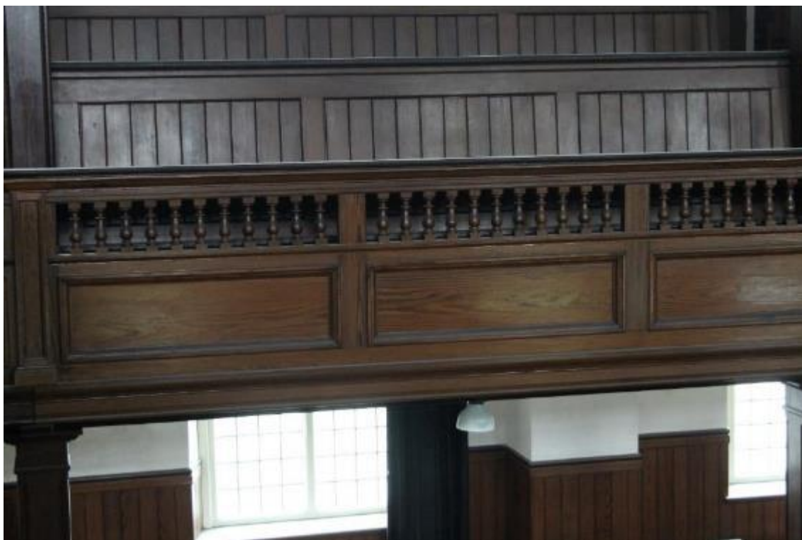
Photo 62: Detail of front of gallery; long panels with open balustrading under top-rail.
