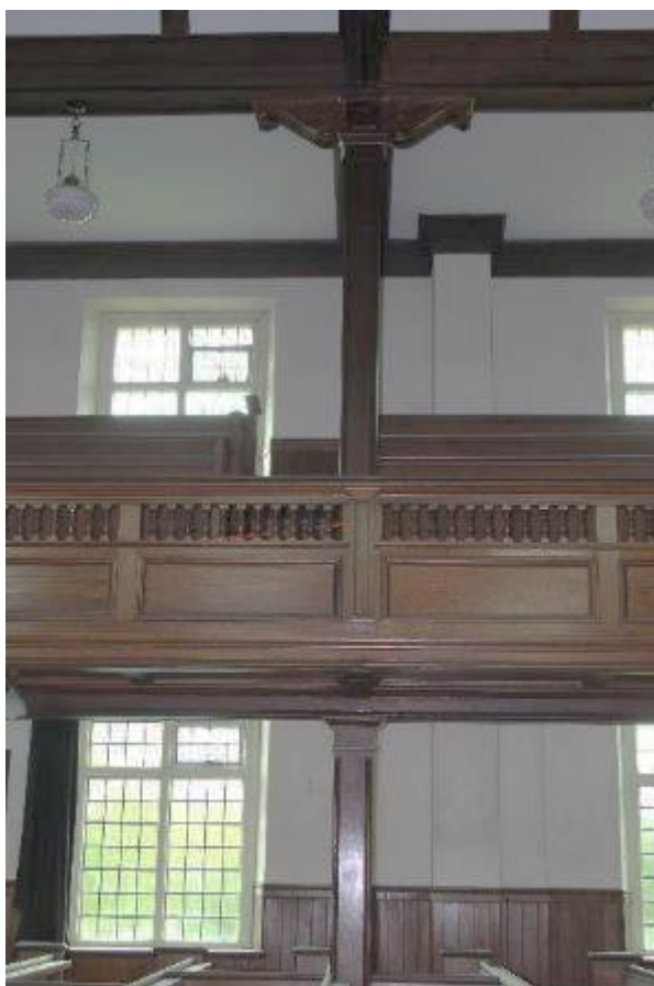
Photo 49: View west at one of eight piers supporting the hipped roof.
