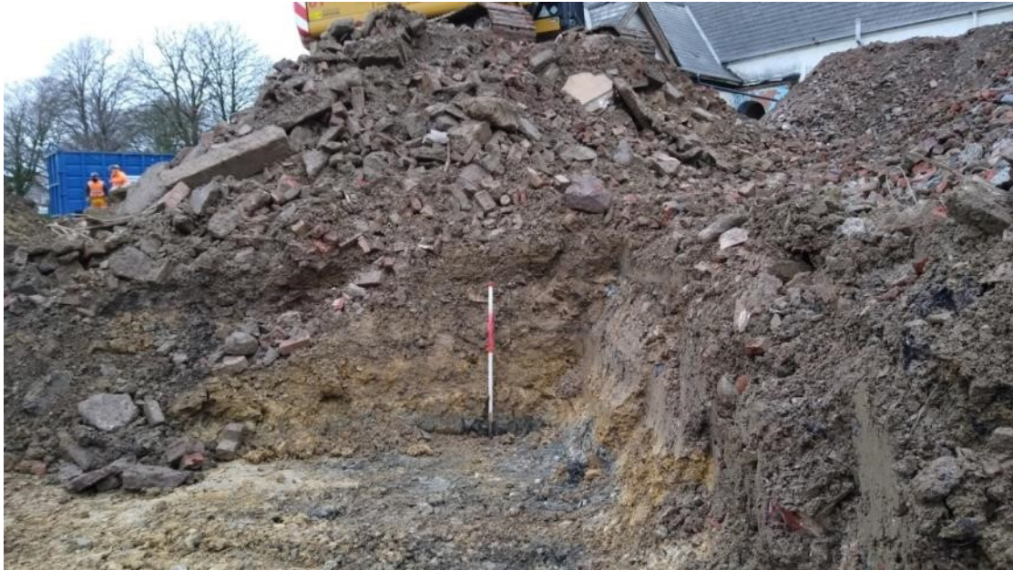
Photo 5: Exposed section in north edge of Area 1 showing layers of imported material (1m scale).
