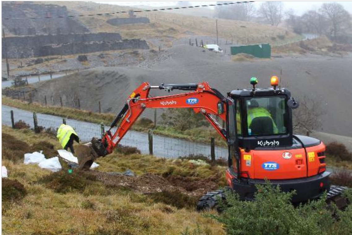
Photograph 2: Machine excavation of trial trenches.
