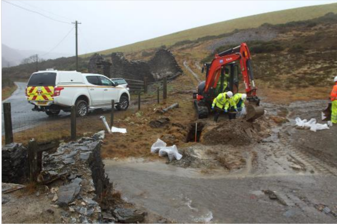
Photograph 3: Machine excavation of trial trenches.
