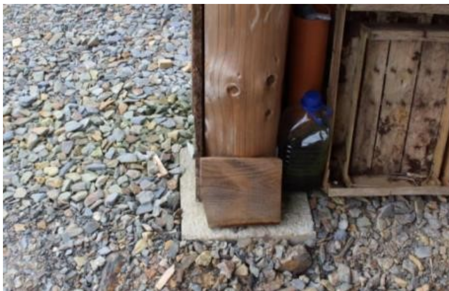
Photo 17: Example of the structural posts and foundation pads.
