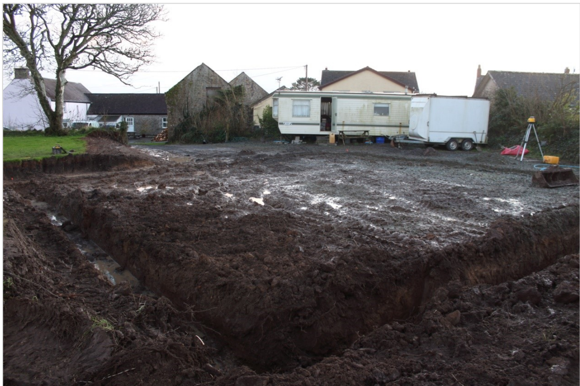
Photo10: View southwest of the completed foundation trenches for the new manager's dwelling.
