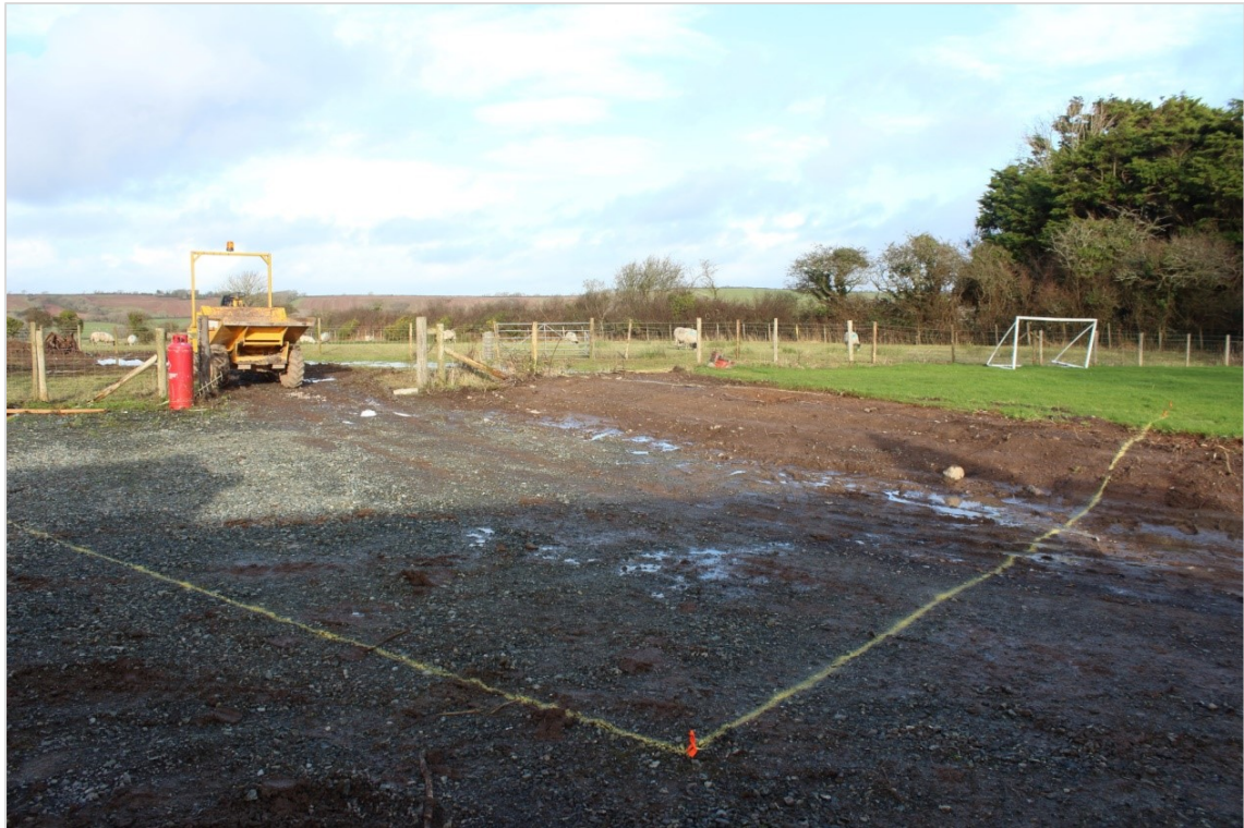
Photo 1: View northeast of foundation trenches marked out prior to excavation.
