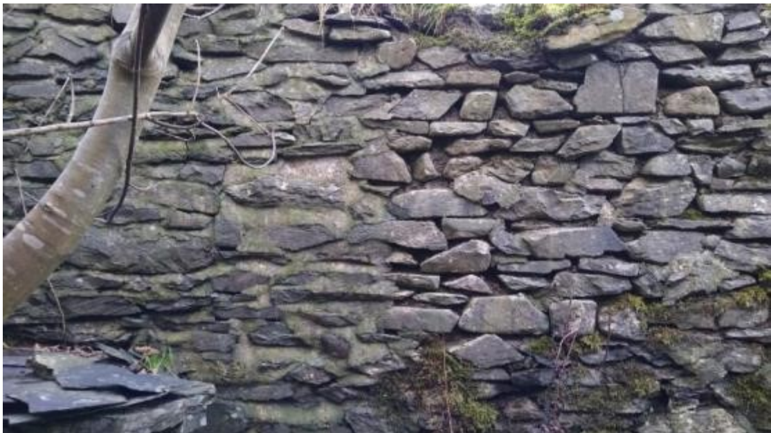
Photo 26 Interior view of north wall of annex showing pointed and unpointed stonework
