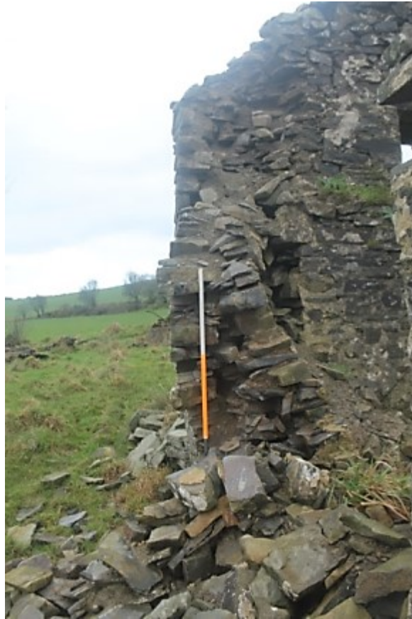
Photo 3: Exposed corework at west side of frontage – 1m scale
