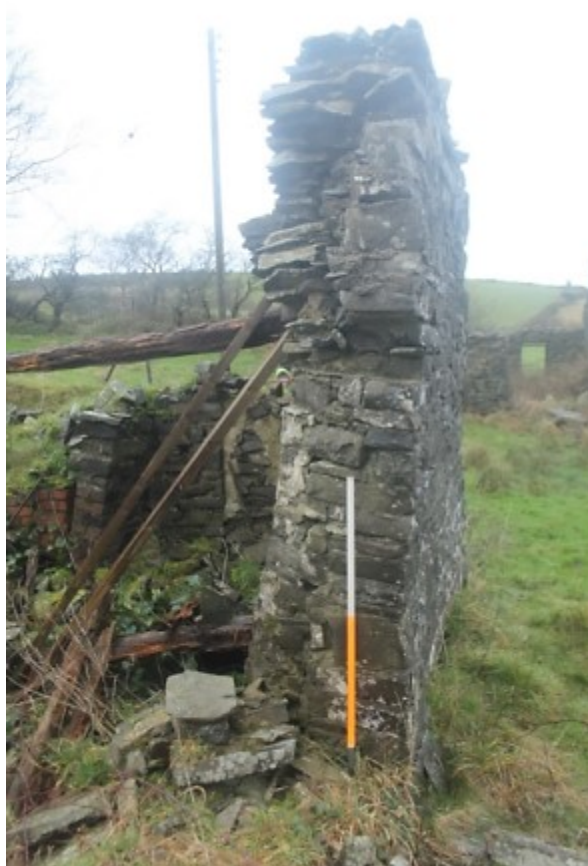
Photo 6: Remains of splayed window in east side of frontage – 1m scale
