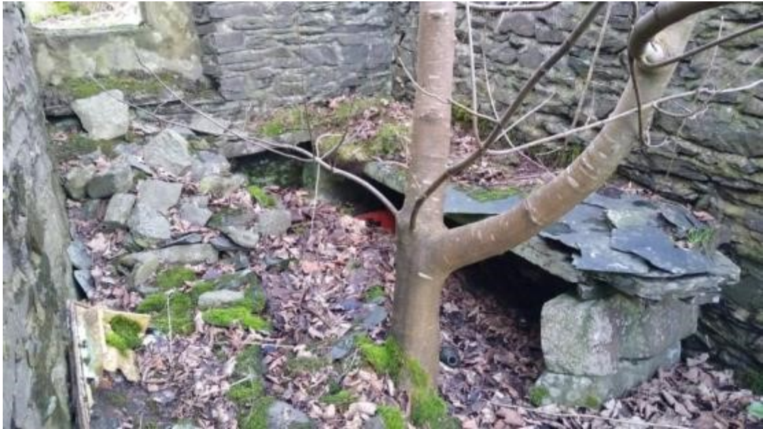
Photo 25 Northwest corner of dairy with slate-slab benches
