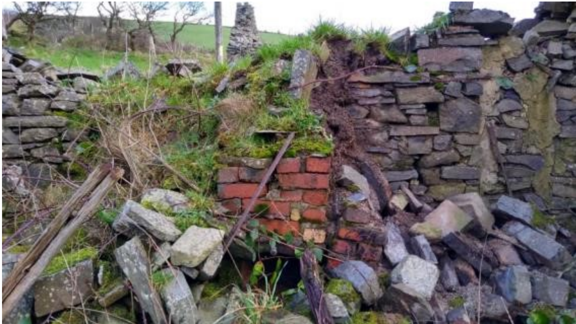
Photo 20: Interior east wall of kitchen (brick oven can be partially seen -1m scale
