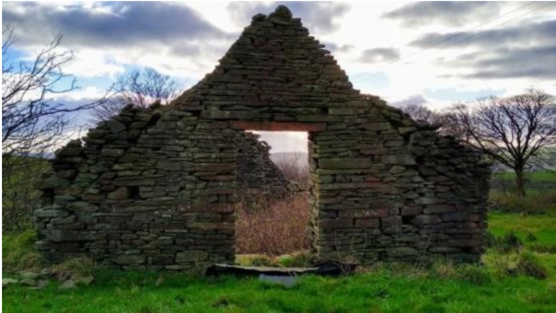
Photo 37: North elevation of granary. Note roofline has been modified
