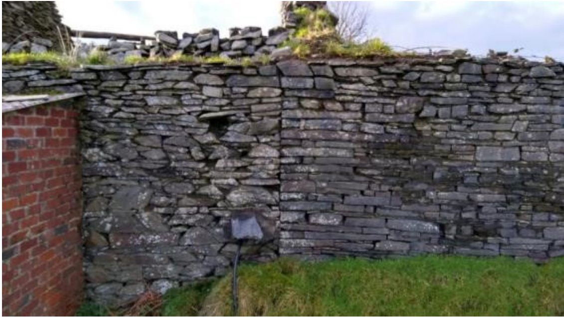
Photo 31: Vertical joint between cowshed and barn in east elevation
