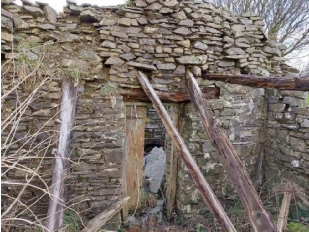
Photo 19: Northeast interior corner of kitchen with door leading to scullery with later stonework above doorway
