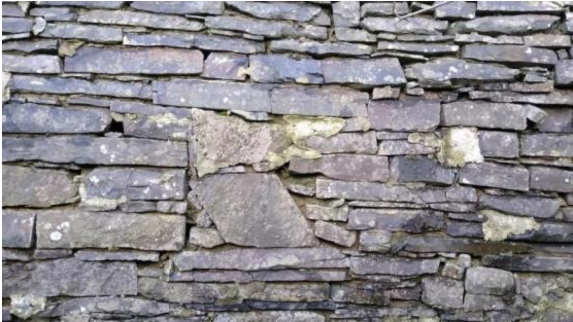
Photo 27: Blocked window in north wall of house
