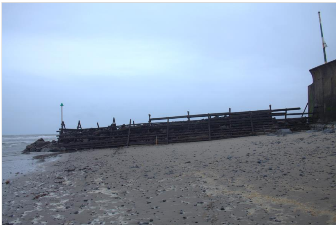
Photograph 14: Showing south-western breakwater extension constructed of railway track and stone. Looking north, 1m scale.
