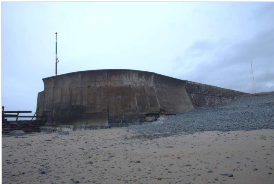
Photograph 13: Showing stone phase of south-western breakwater at the lower level, rebuilt in concrete. Looking north-east.
