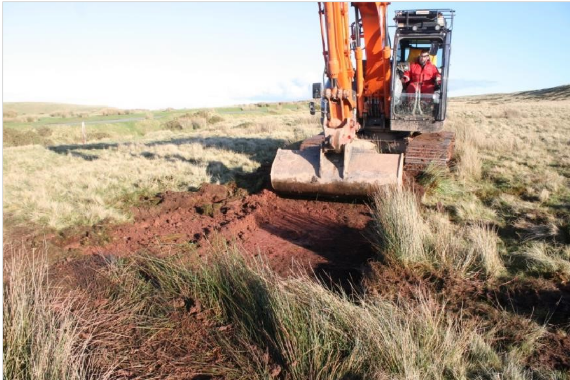
Photo 5: View north east of initial removal of topsoil within footprint of the workers compound area
