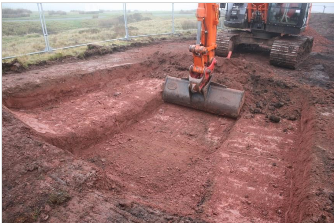
Photo 8: View north east of excavation of pipe trench and benching of both sides
