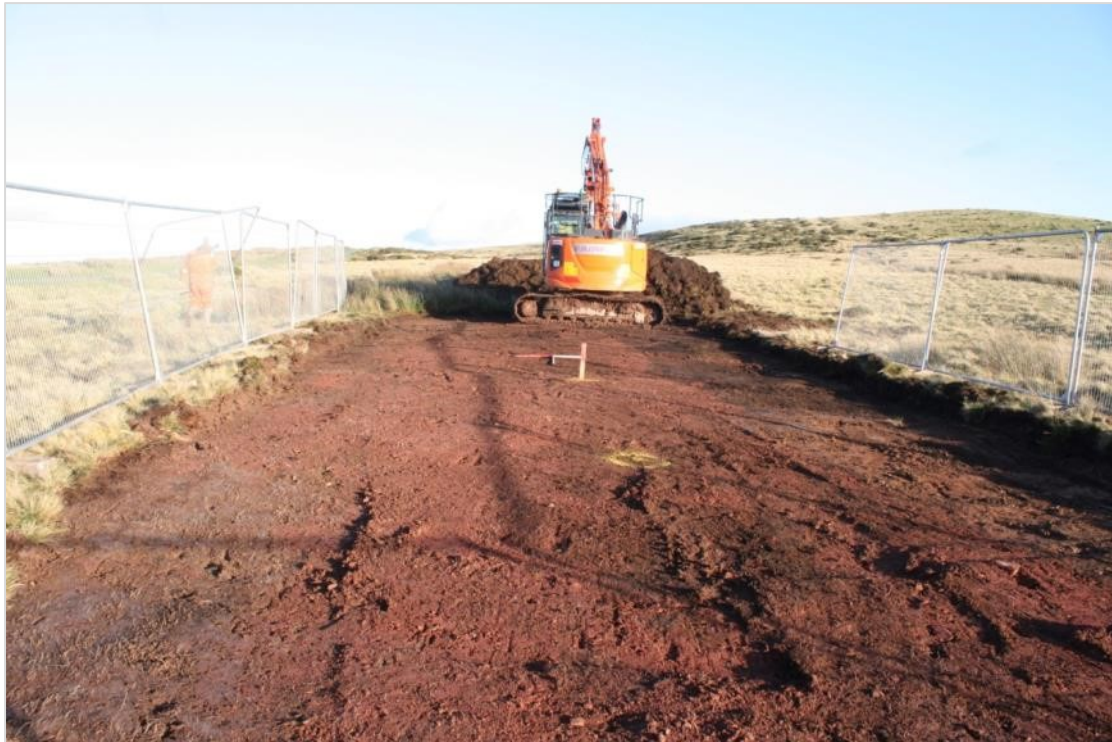
Photo 7: View of completed workers compound with backfilled pipe trench visible as a central red corridor of soil [1001], flanked either side by subsoil [1002]. 2 x 1m scales
