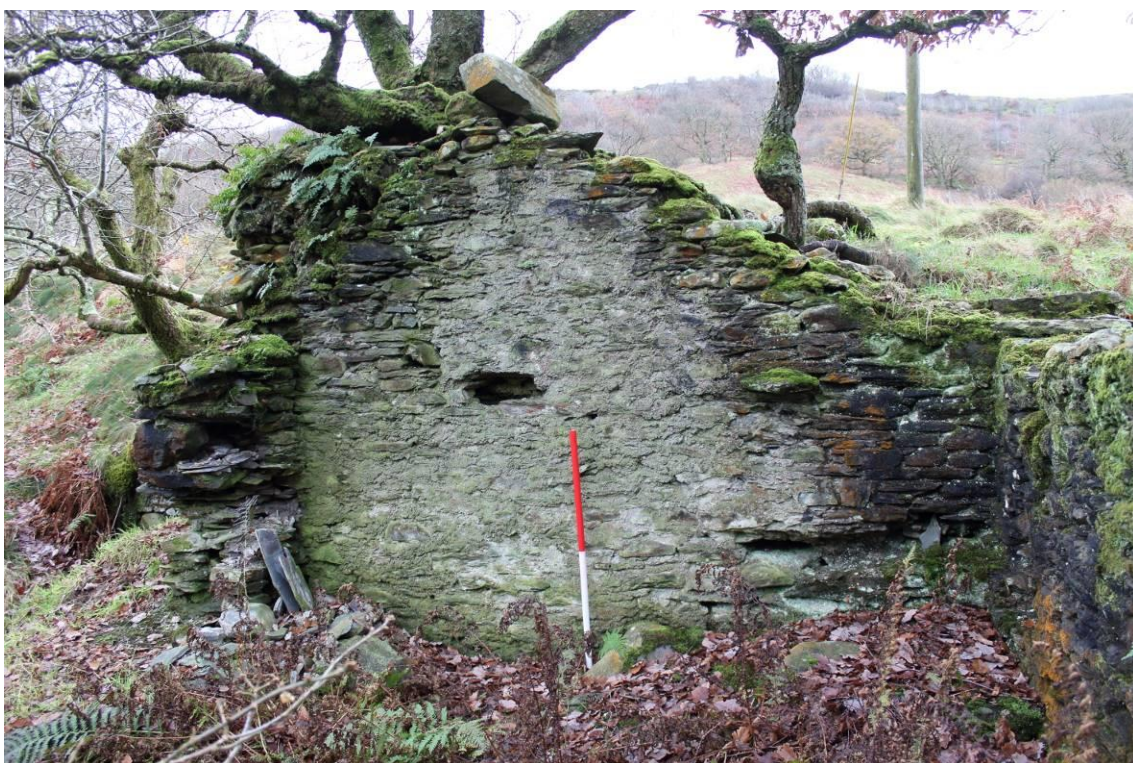
Photo 11: The internal elevation of the southern gable end of winding house PRN125585, with the possible remnants of a thin limewash. 1m scale (DAT Photo 125592_3450).
