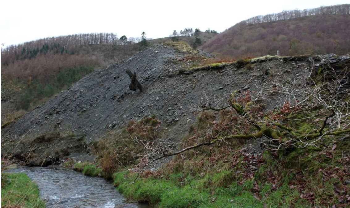
Photo 20: A wooden post is seen protruding out from the actively eroding, steep southern slope of development tip PRN96393 (DAT Photo 125592_3469)
