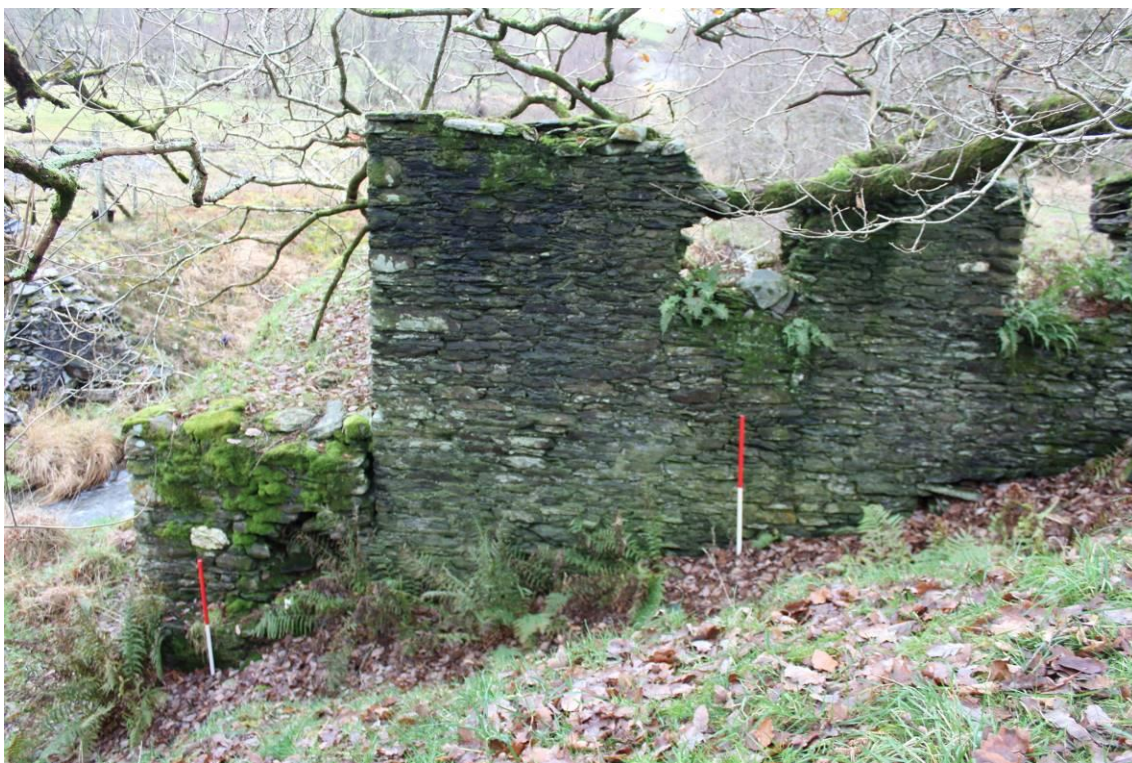
Photo 13: The northern end of the western elevation of winding house PRN 125585 and the abutting platform or revetement at its northern end. 1m scale (DAT Photo 125592_3454)
