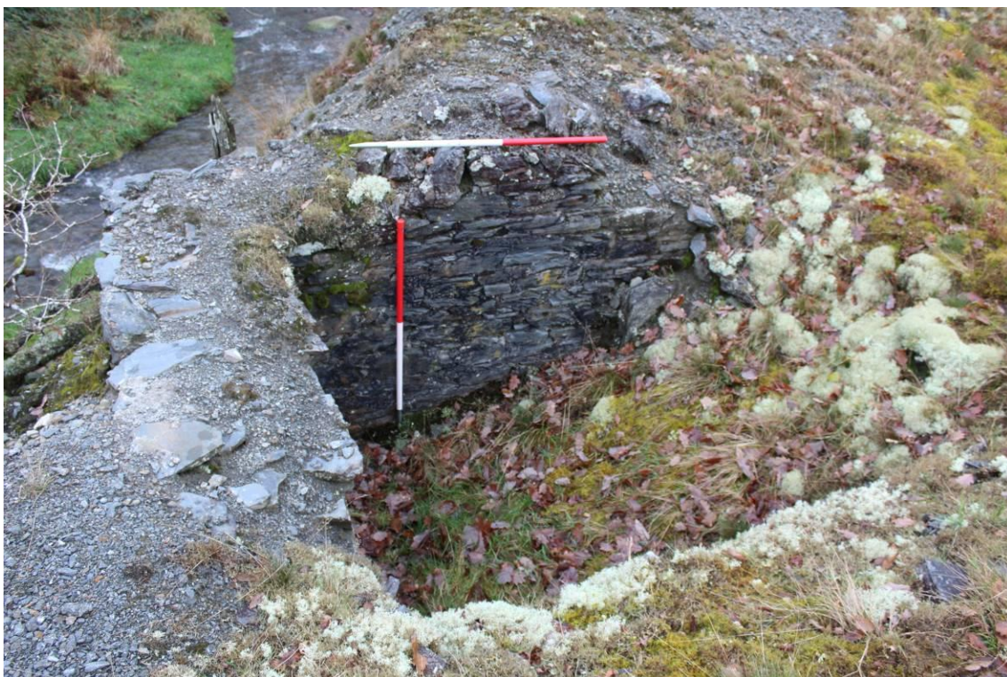
Photo 15: The square masonry collar for shaft PRN69390. Facing west. 1m scale (DAT Photo 125592_3460)
