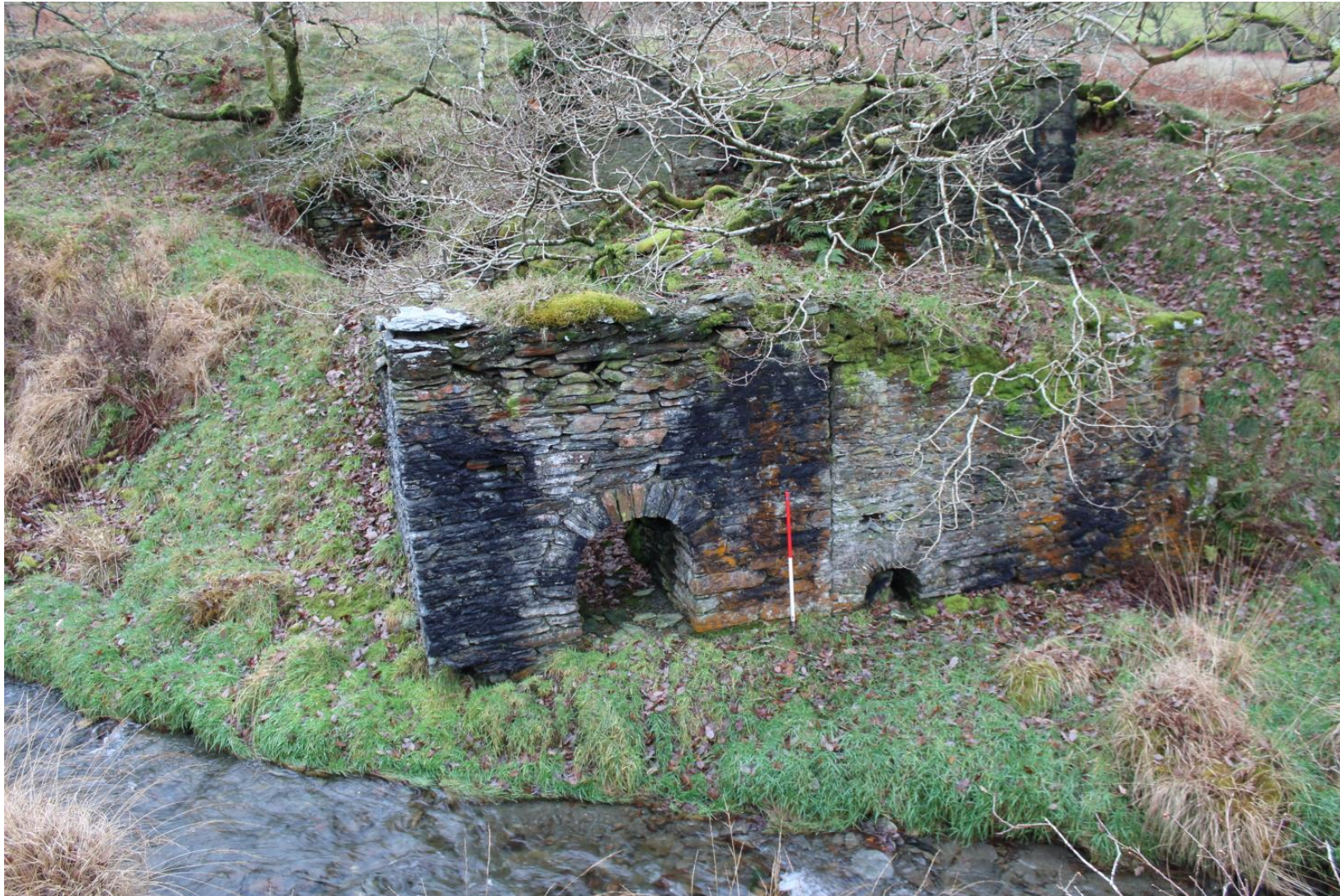
Photo 8: The north facing elevation of wheelpit PRN96394. 1m scale (DAT Photo 125592_3458)
