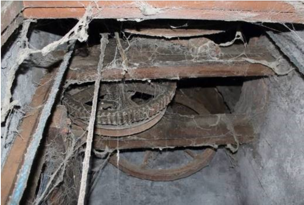
Photo 58: Detail of the dumbwaiter pulleys.
