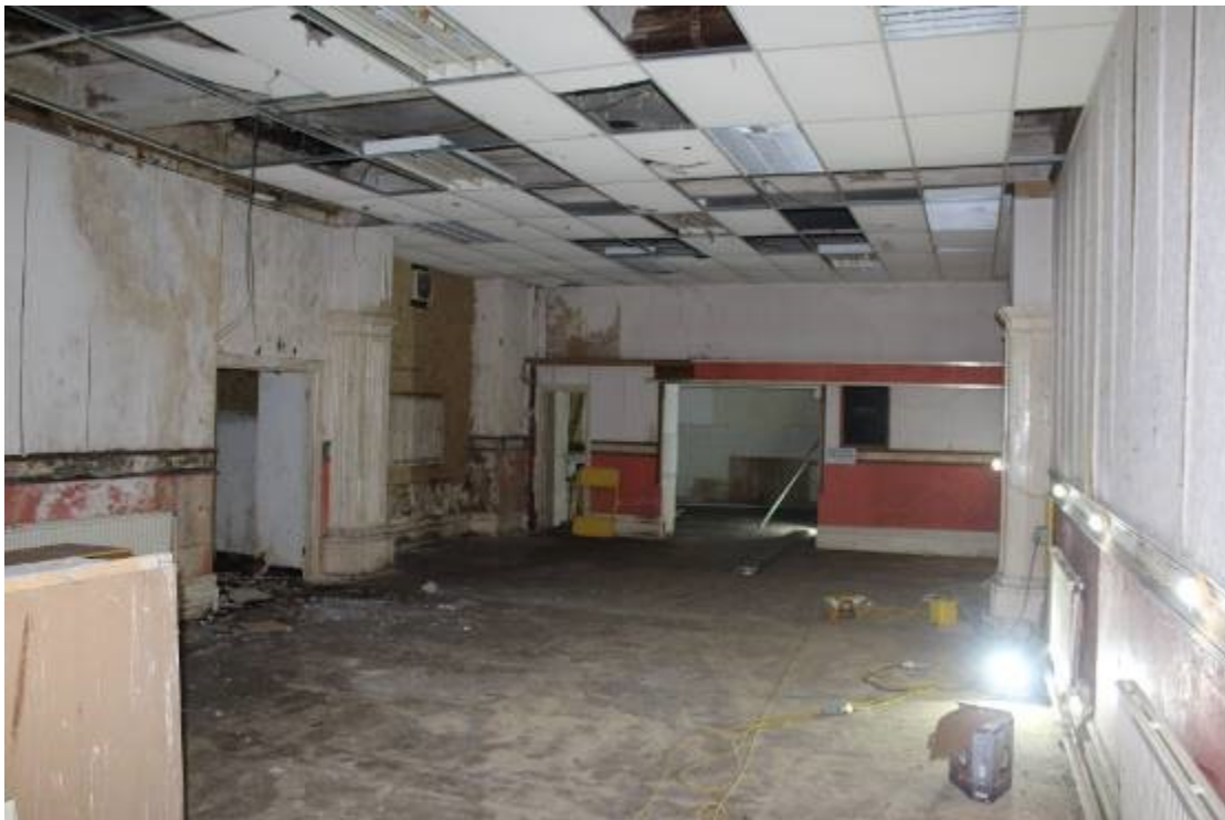
Photo 16: Southwest facing of the main hall room, with kitchen opening to the rear, potentially inserted through a former fireplace. 2m scale.
