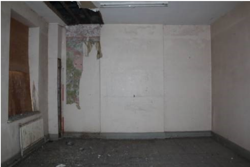
Photo 51: Southwest facing shot of the 2 nd floor rear room, showing the blocked fireplace in the gable wall. 2m scale.
