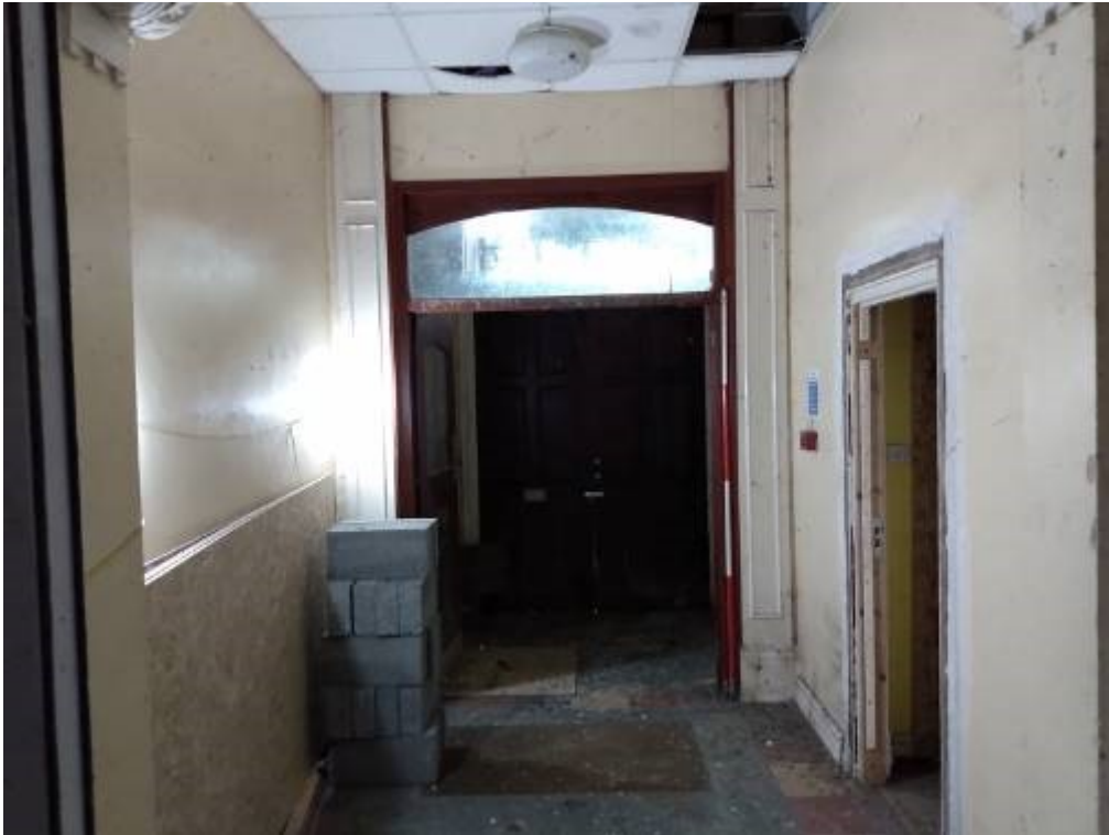
Photo 10: Northwest facing shot of the current main entrance. The left wall and decorated pillars may be original, the remaining features are later inserts 2m scale.
