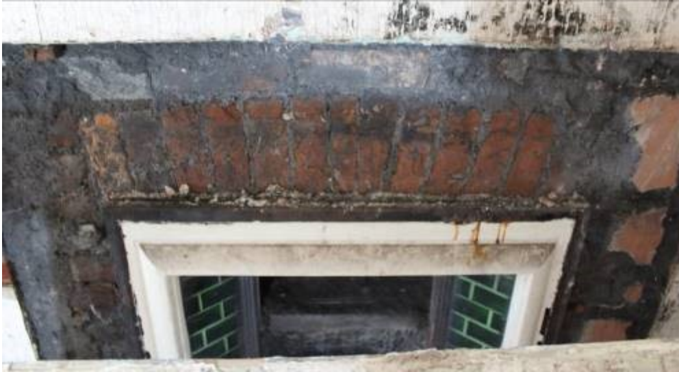
Photo 54: Detail of the brick lintel behind the fire surround.
