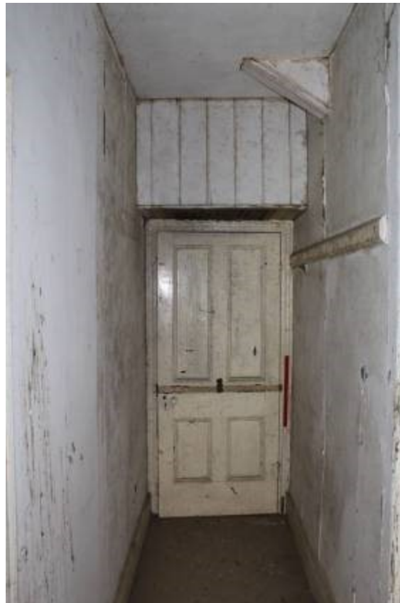
Photo 57: Northeast facing shot along the central 3 rd floor corridor, showing the door enclosing the otherwise open dumbwaiter shaft. 2m scale.
