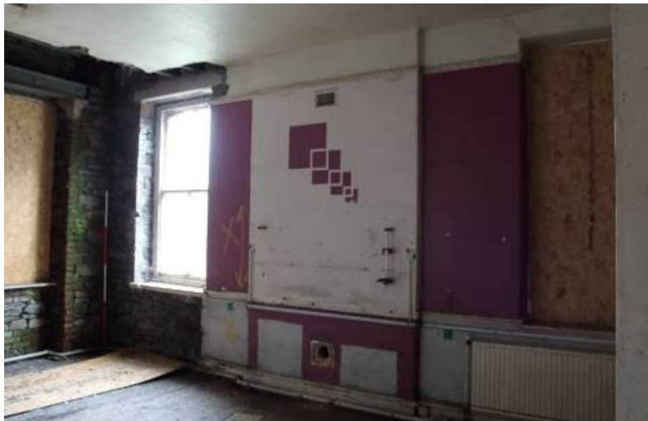
Photo 45: Northeast facing shot of initial 2 nd floor frontage room, showing blocked fireplace in gable wall. 2m scale.
