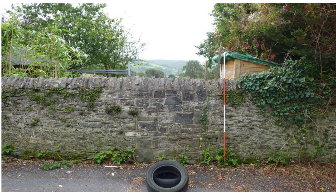
Photo 43: Southeast facing shot of the boundary wall to the adjacent property. The change of masonry potentially indicating an infilled gateway. 2m scale.
