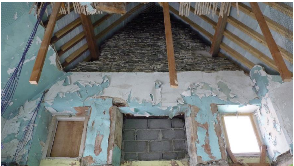
Photo 18: Southwest facing shot showing the replaced roof structure, exposed walling and partly blocked openings.
