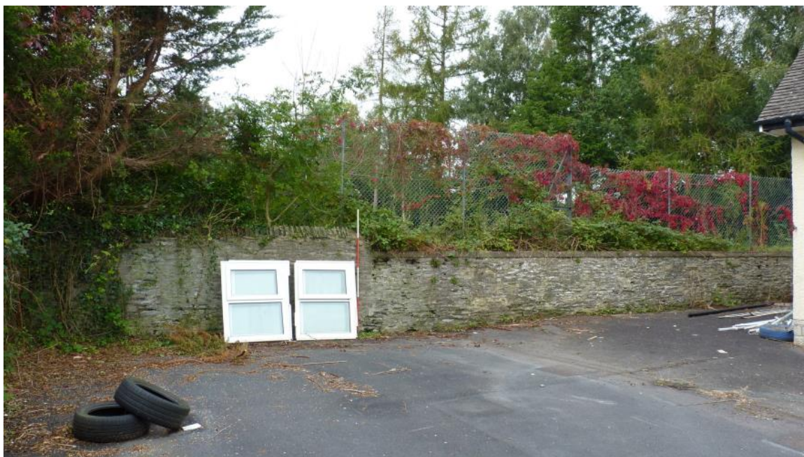
Photo 42: Southwest facing shot showing the boundary wall to rising ground, the change of height signifying a potential area of later rebuild to the right. 2m scale.
