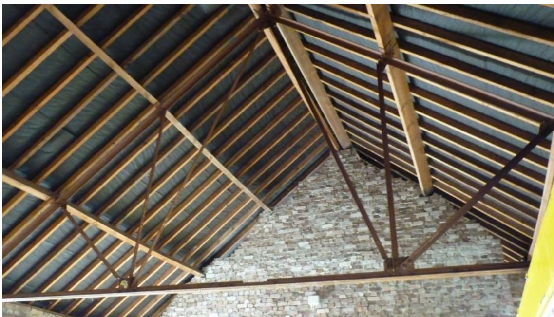
Photo 38: Detail of the roof structure in the later extension.
