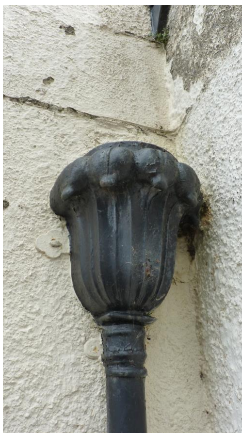
Photo 11: Detail of drain pipe hood on the easternmost entrance block.
