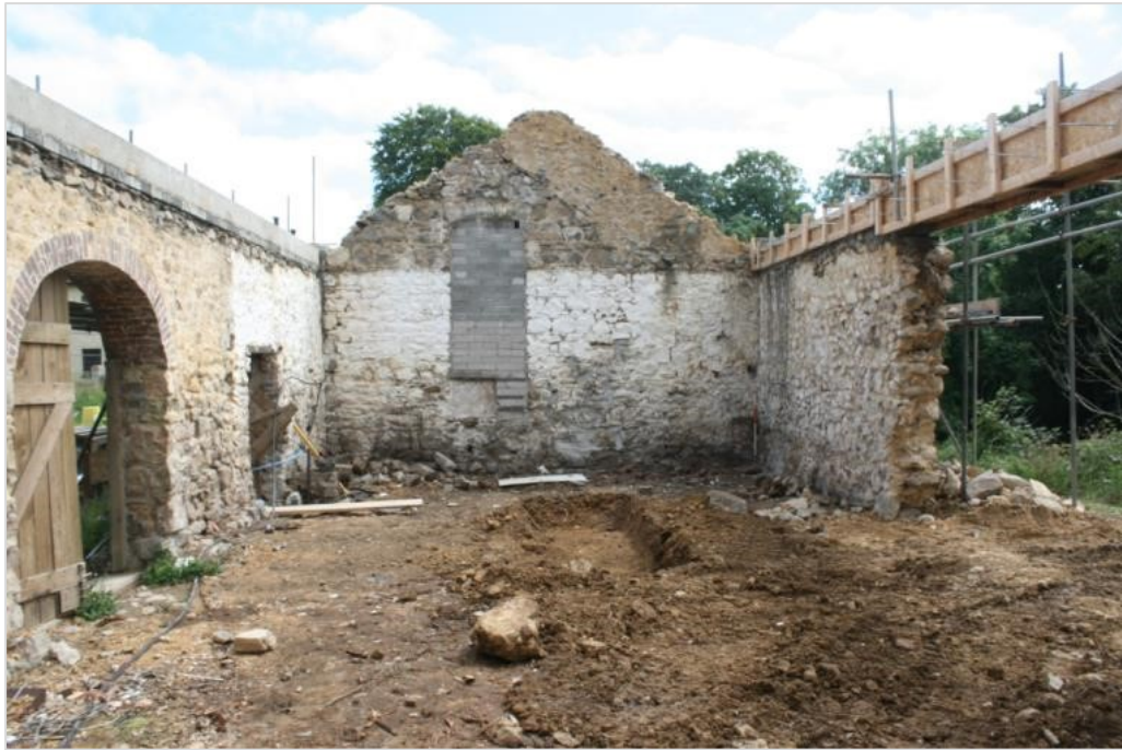
Photo 12: The location of the test pit in Building 3 and infilled opening in the southern gable of Building 3 (DAT Photo).
