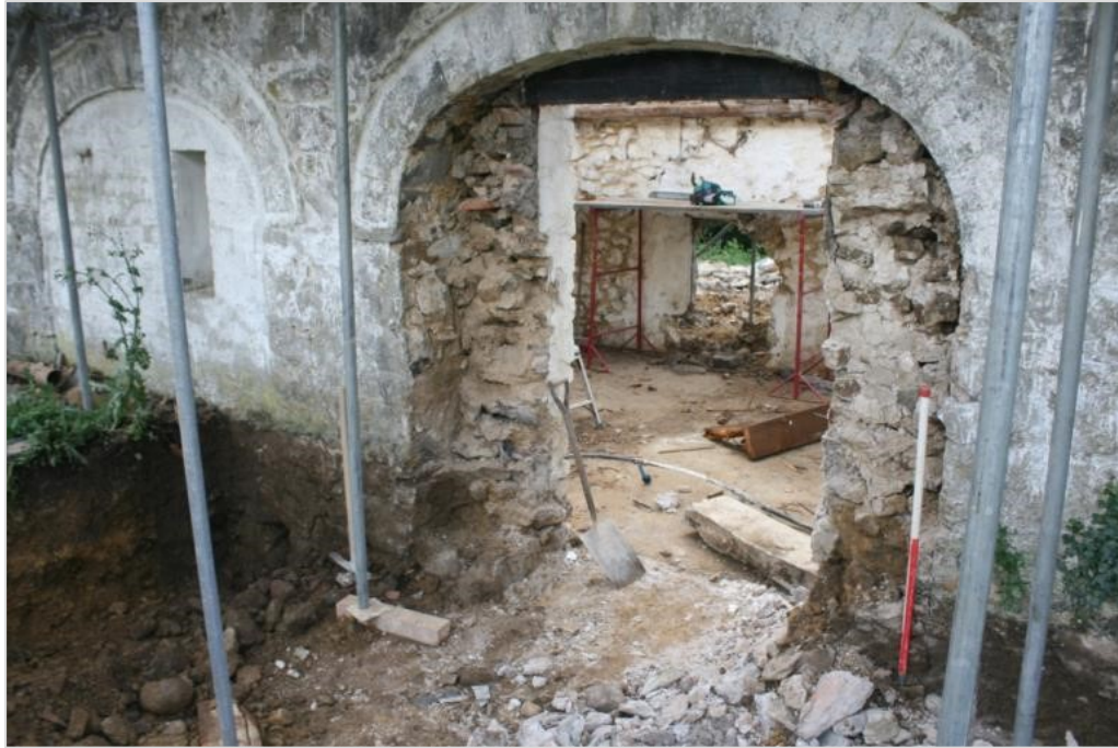
Photo 17: The partially widened central opening in the east facing elevation of Building 2 (DAT Photo)
