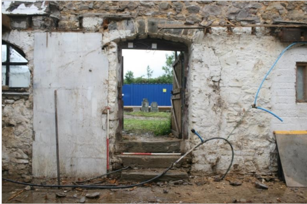
Photo 15: The internal elevation of the central, infilled opening in the east facing elevation of Building 2 showing the inserted steps and difference between the internal and external ground levels (DAT Photo)
