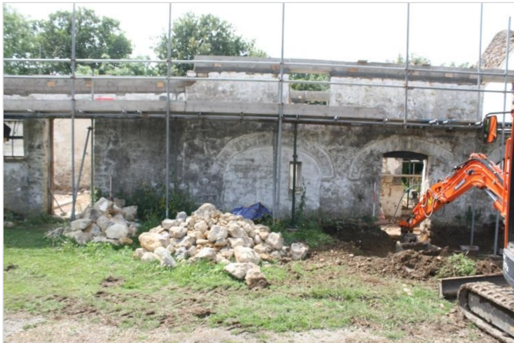
Photo 14: The southern and central infilled openings in the east facing elevation of Building 2 (DAT Photo)
