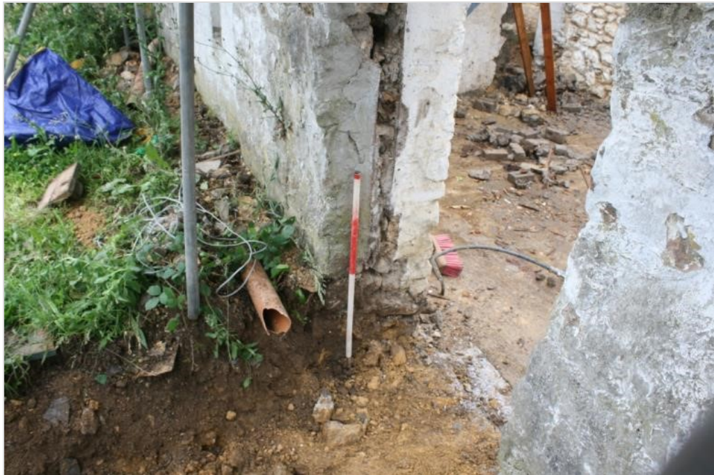
Photo 16: The reduced ground level and truncated water pipe of the central infilled doorway in the east facing elevation of Building 2 (DAT Photo)
