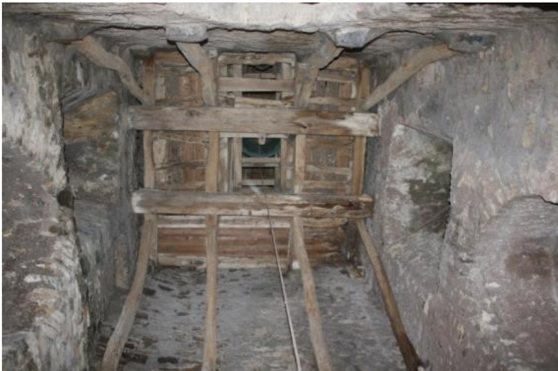
Photo 29: View of wooden belfry underfloor from the first floor of the tower.
