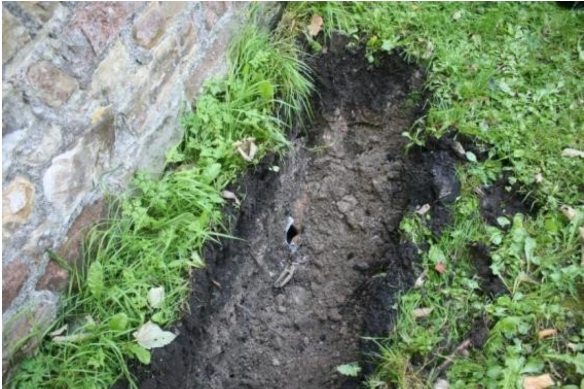
Photo 2: View southwest of Victorian French drain exposed north of vestry.
