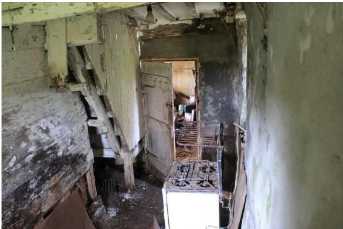
Photo 61: Doorway from dairy to hall (horizontal-boarded partition and rear of stairwell to left).
