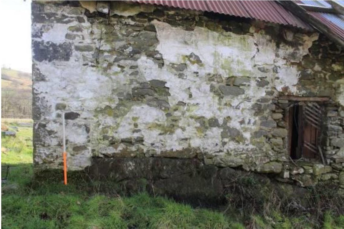
Photo 32: North end of west wall of house (note rising bedrock in wall). 1m scale
