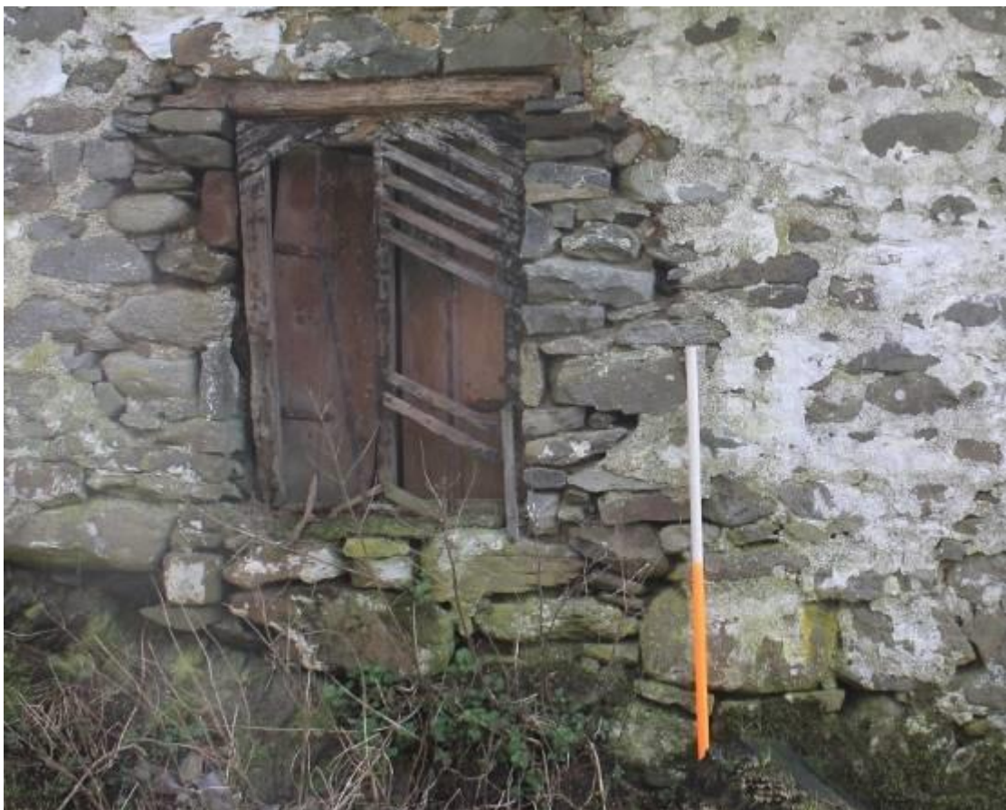
Photo 29: Shuttered window (located in dairy) in west wall of house. 1m scale
