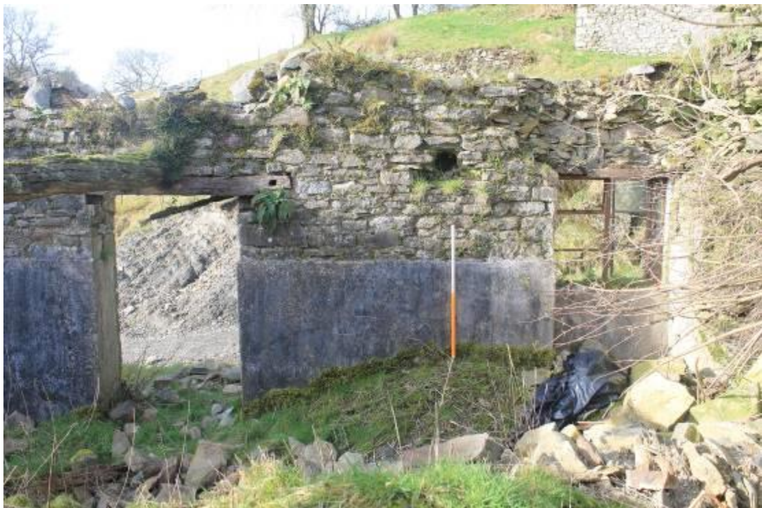
Photo 82: Two openings in west wall of byre (blocked opening originally rear entrance to cross passage) (north end)
