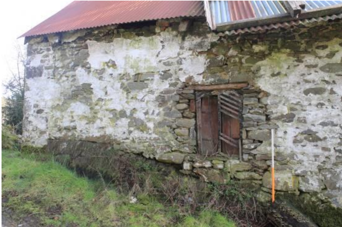
Photo 28: West wall of house (note rising bedrock). 1m scale
