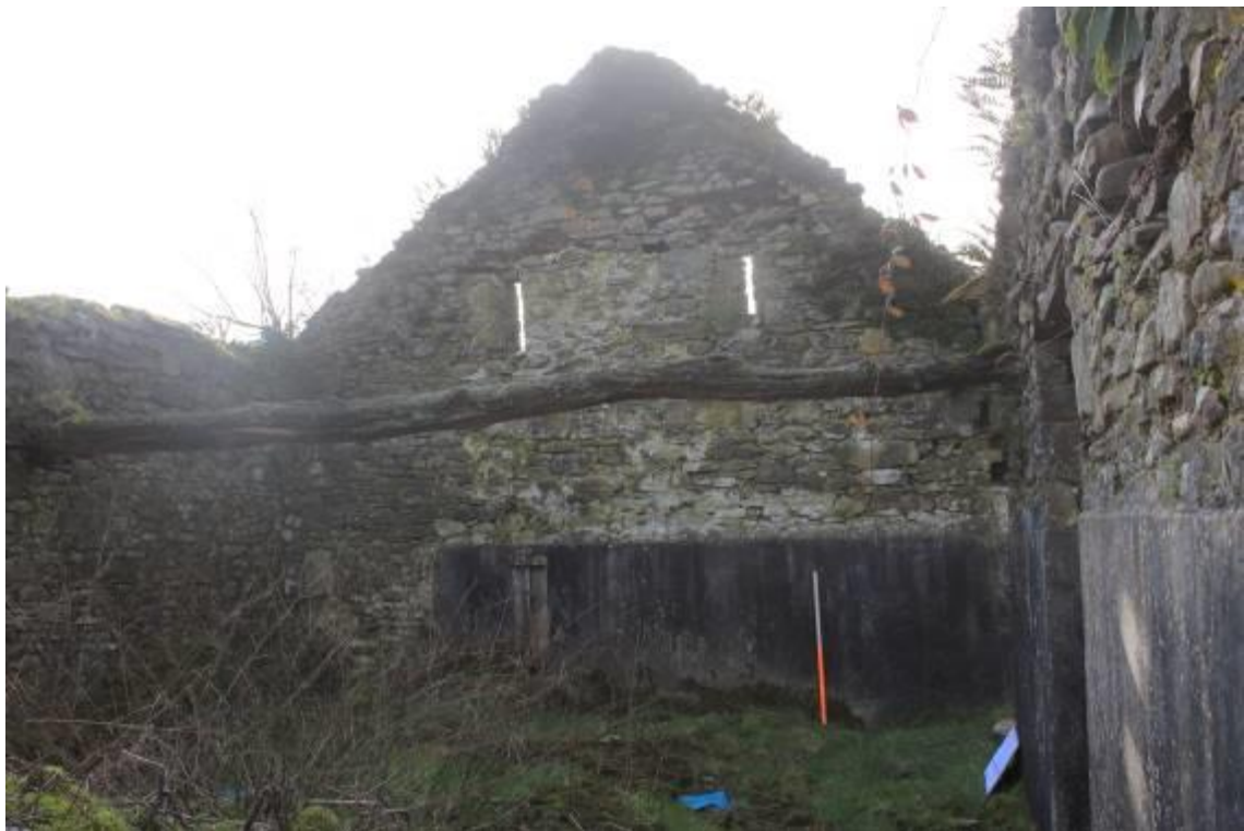
Photo 78: South gable of byre showing loops and crossbeam
