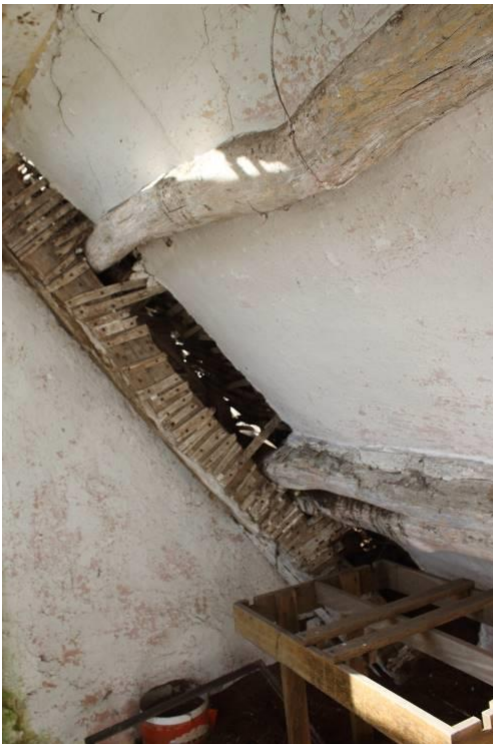
Photo 75: Purlins visible above stair landing
