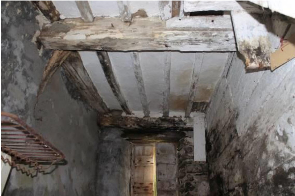
Photo 63: Looking north at dairy ceiling showing cross beam and ceiling joists; part of scarfed cruck can be seen on left (west) wall.
