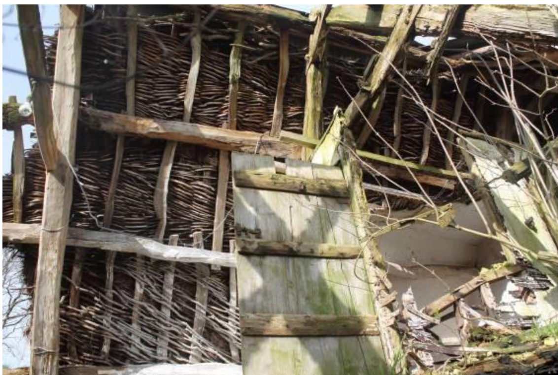
Photo 73: Exposed roof in south end of house showing part of yoked apex, purlins, split ash rafters and underthatch of hazel
