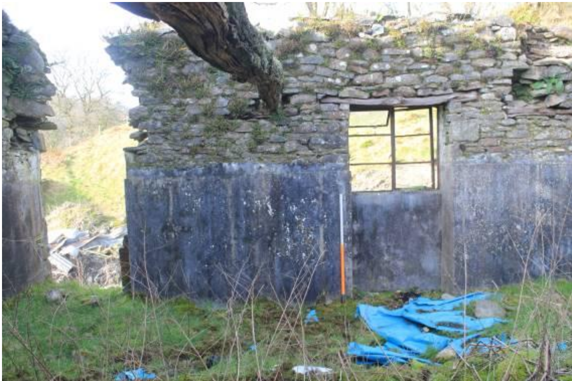
Photo 80: Southern end of west wall of byre showing two doorways (one blocked and window inserted)
