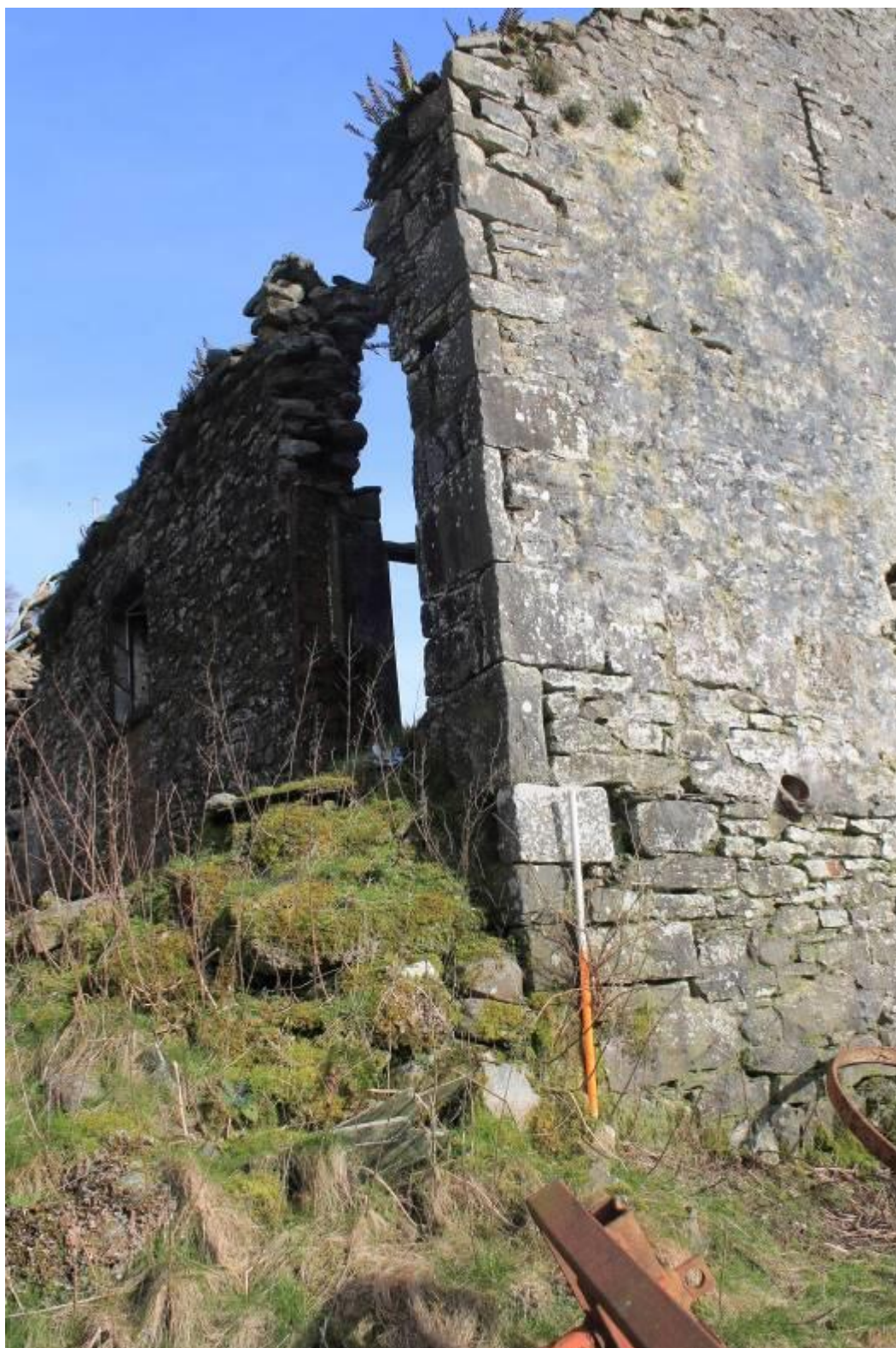
Photo 22: Quoins at southwest corner of byre. 1m scale
