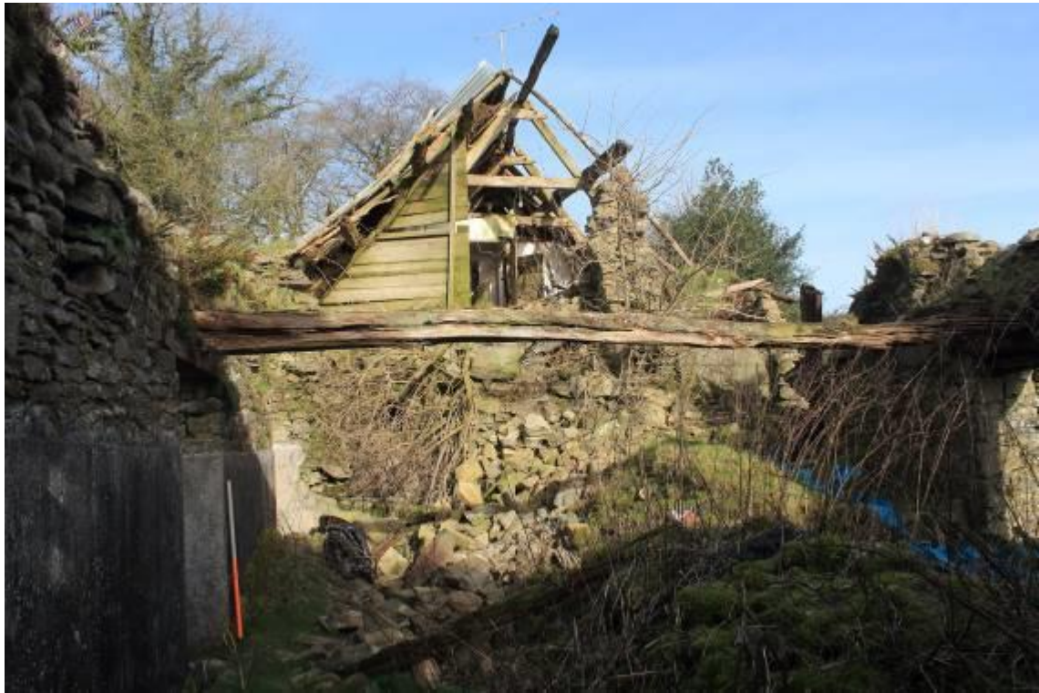
Photo 77: North end of byre (wall is obscured by collapse of south gable end); one of a pair of cross-beams shown.
