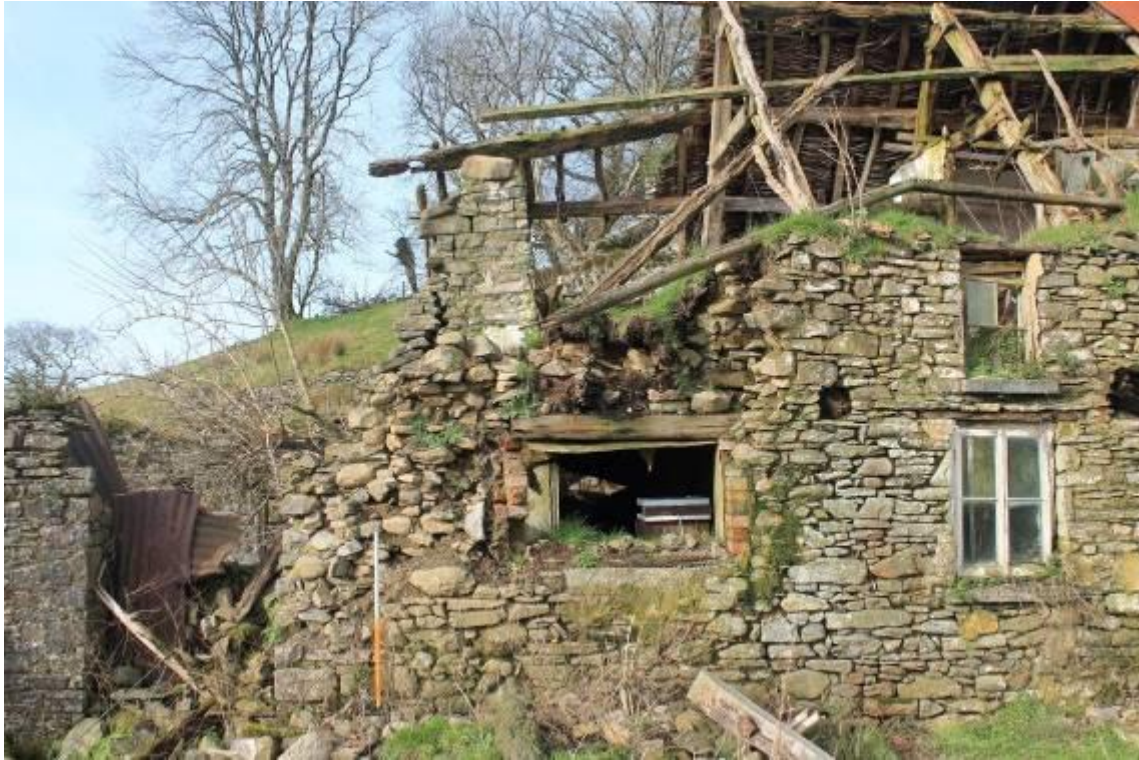
Photo 13: Detail of southern end of house showing modern window (right of 1m scale) and entrance to former cross-passage (left of 1m scale)
