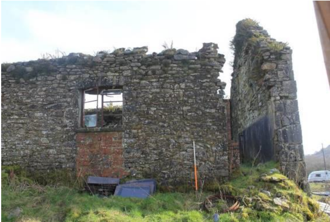
Photo 23: Blocked entrance with stone voussoirs (left of 1m scale) and corner entrance in west wall of byre. 1m scale
