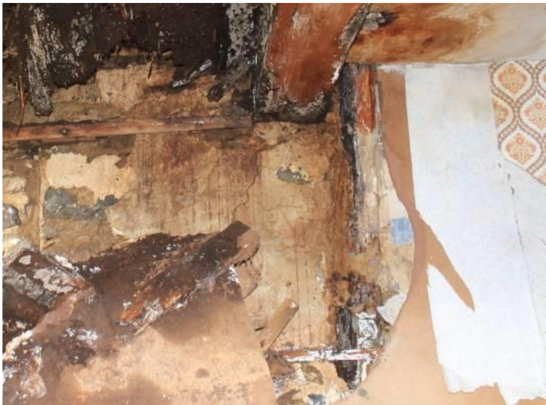
Photo 52 Close-up of foot of scarfed cruck in west wall of hall
