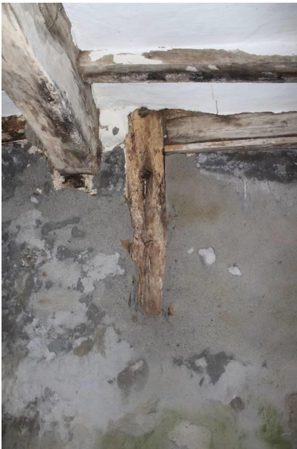
Photo 62: Scarfed cruck in west wall of dairy (north of window)
