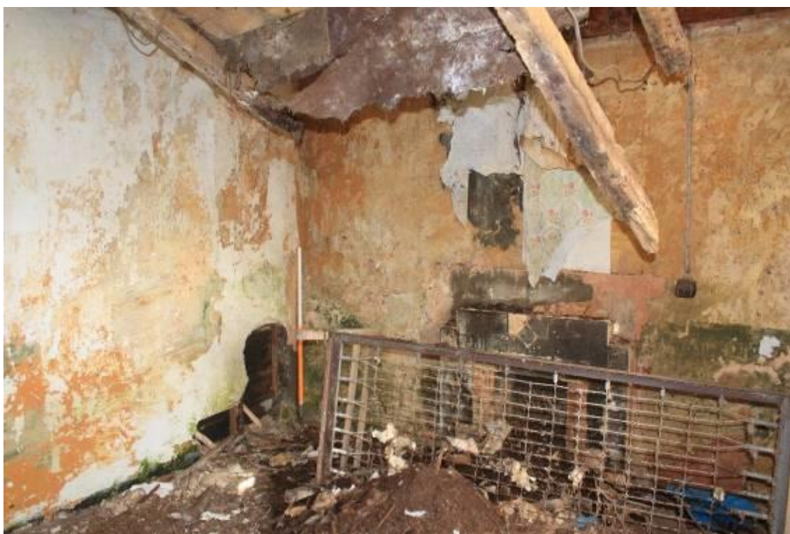
Photo 46: Northwest corner of parlour. Dairy partition (horizontal boards) can be seen in hole next to 1m scale.
