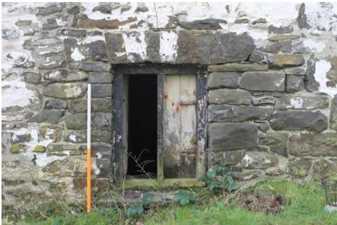
Photo 33: Shuttered window with stone voussoirs (located in dairy) in north wall of house. 1m scale
