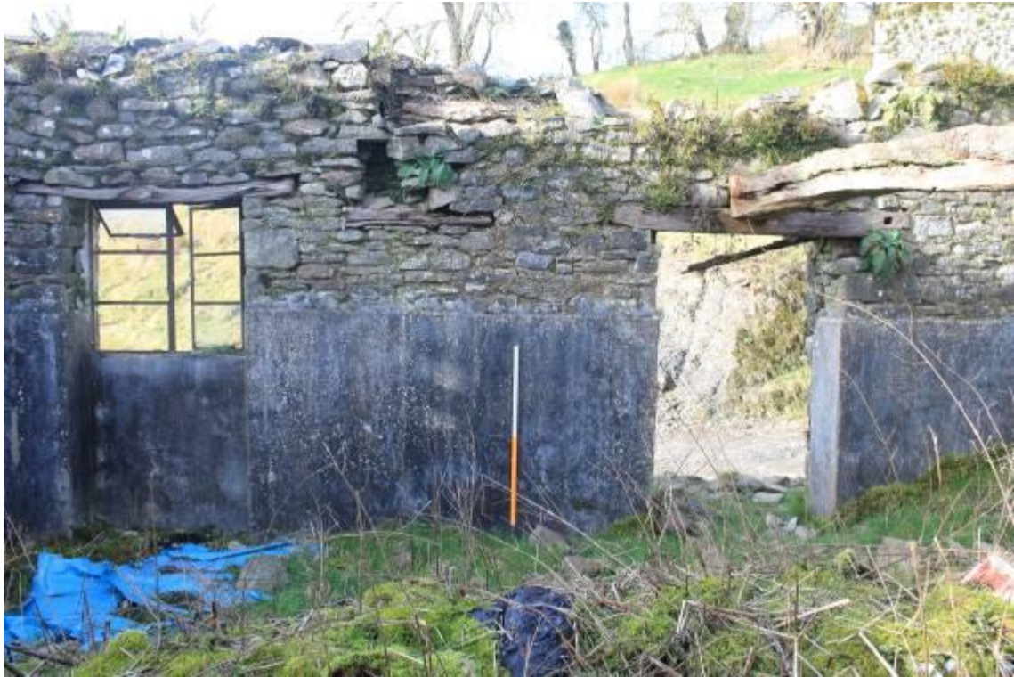
Photo 81: Two openings in west wall of byre (one blocked and window inserted) (south end)
