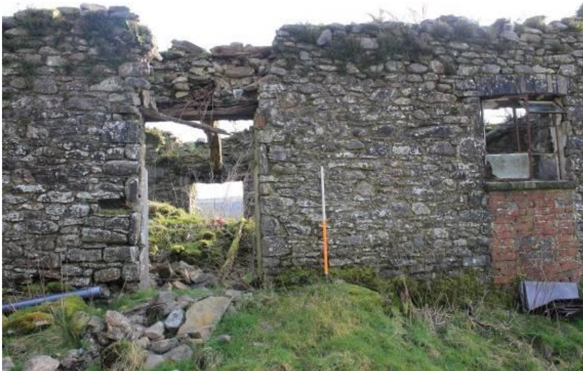
Photo 24: Entrance (with timber lintel) in west wall of byre. 1m scale
