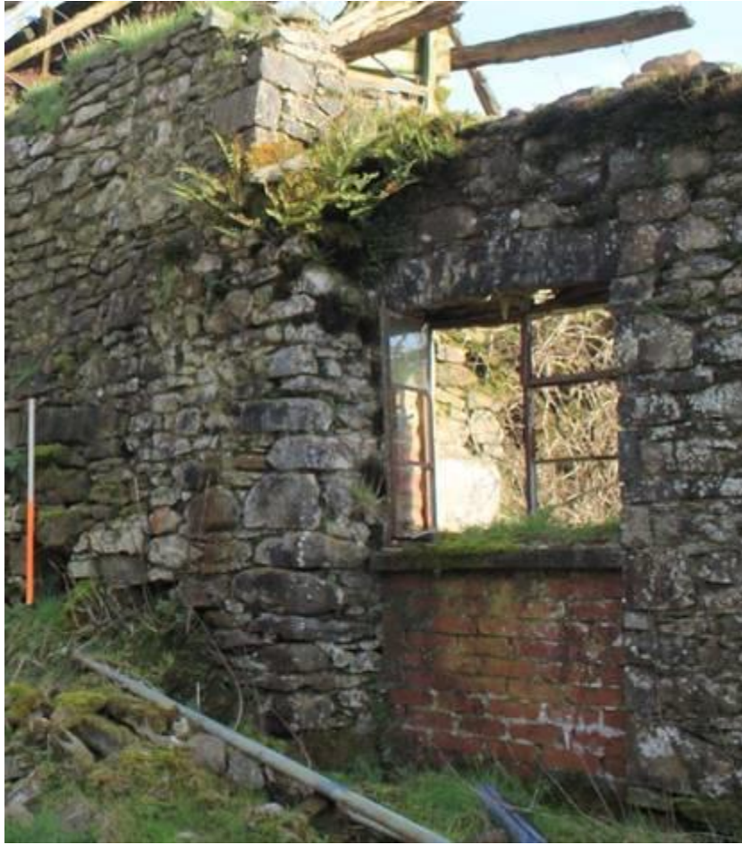
Photo 25: Detail of blocked entrance to former cross-passageway in west wall of byre. 1m scale
