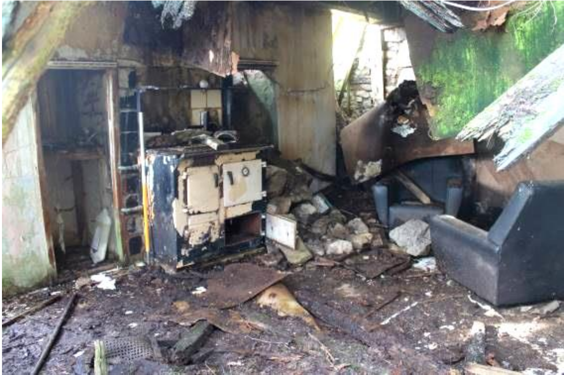
Photo 53: Fireplace in south wall of hall – recesses on either side of Aga represents original width of fireplace. Entrance to stone staircase on the far left.
