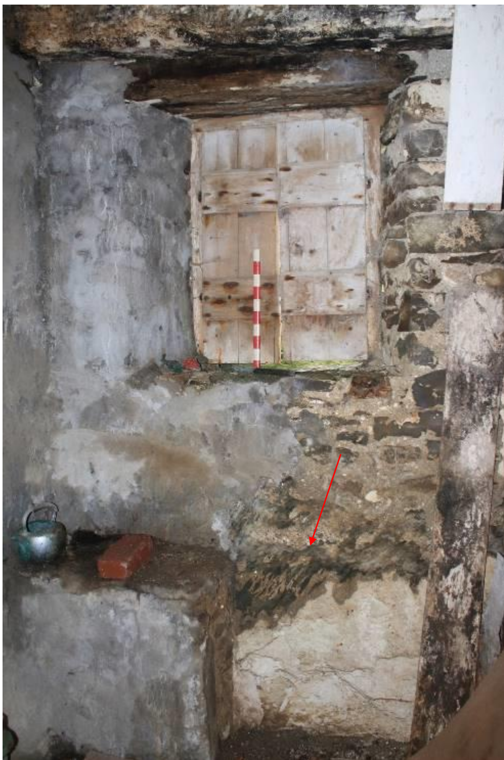
Photo 60: Shuttered window in north wall of dairy (top of bedrock arrowed)
