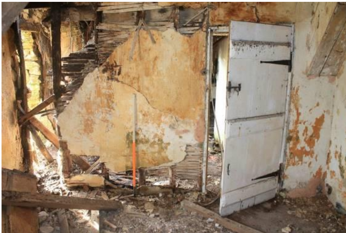
Photo 43: South (lathe and plaster) wall of parlour; door leads to lobby.
