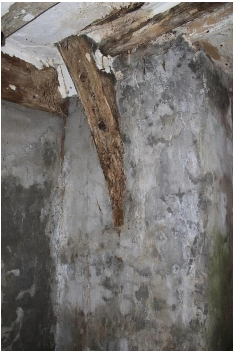
Photo 65: Scarfed cruck in west wall of dairy (south of window)
