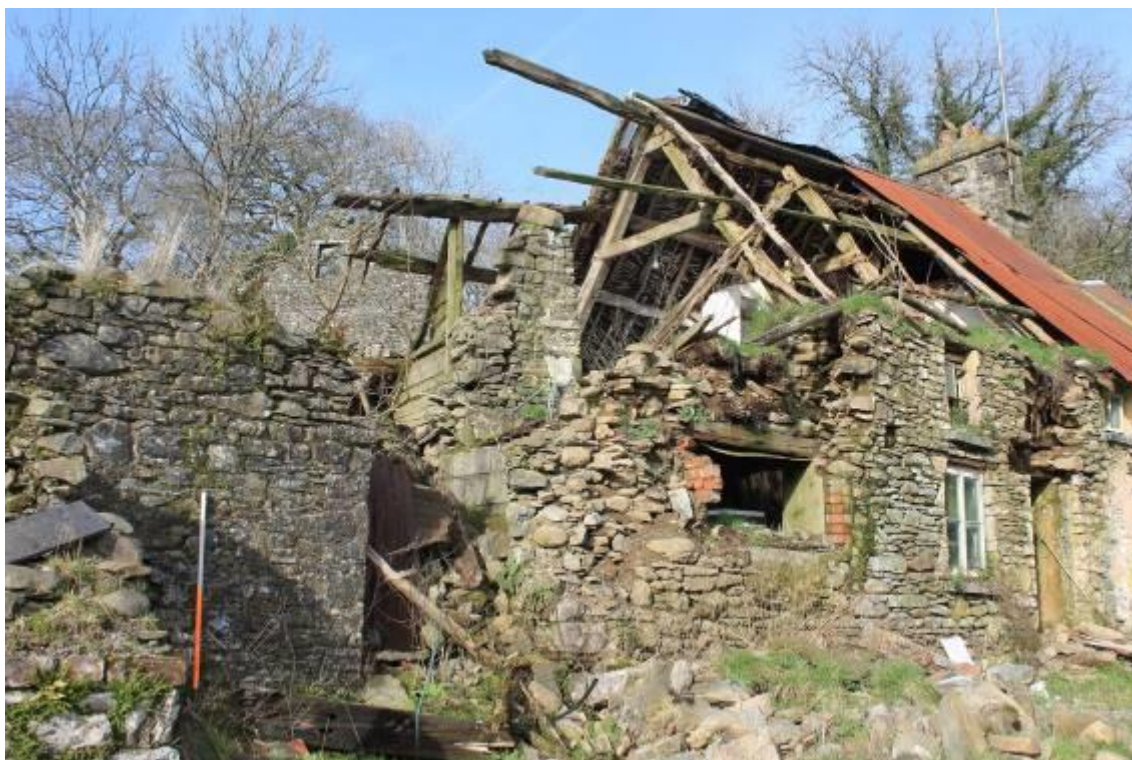
Photo 17: View north towards collapsed south end of house and exposed roof timbers. 1m scale
