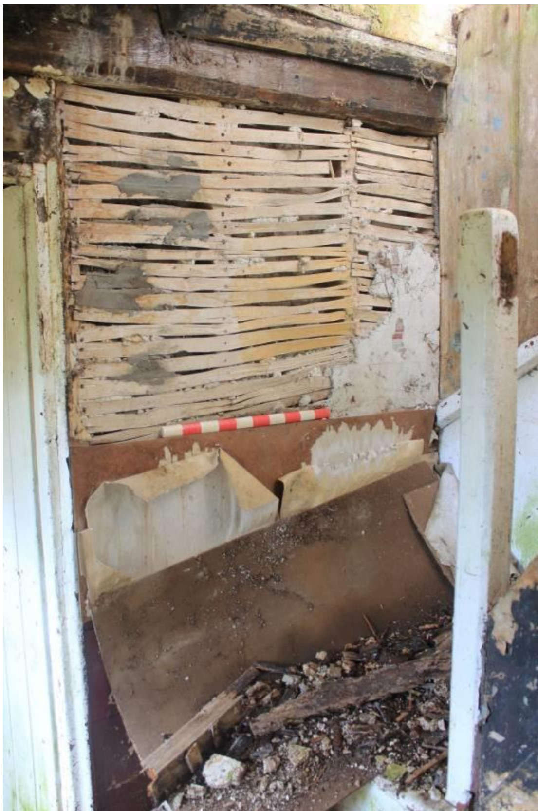
Photo 41: Lathe and plaster partition in stairwell (hall behind)
