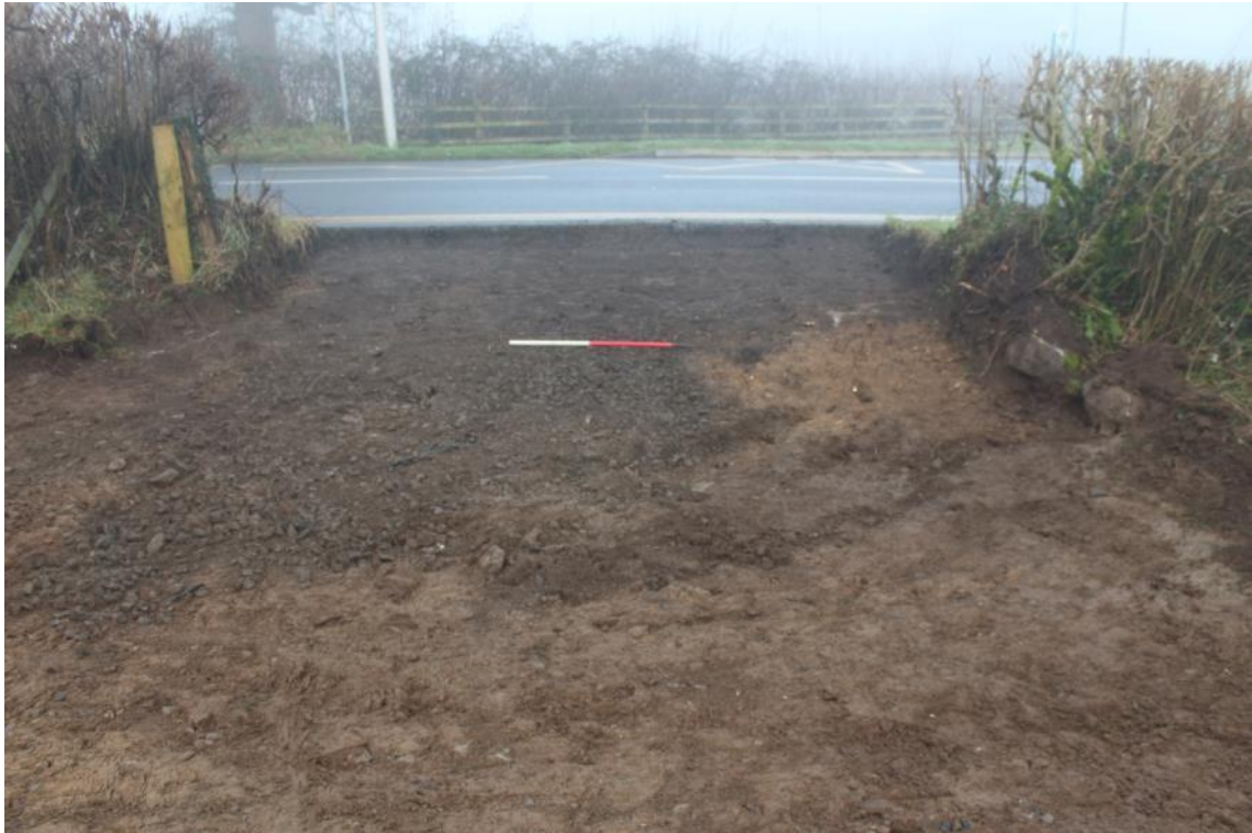
Photo 1: View north: topsoil strip for access road beside existing gateway (1m scale)
