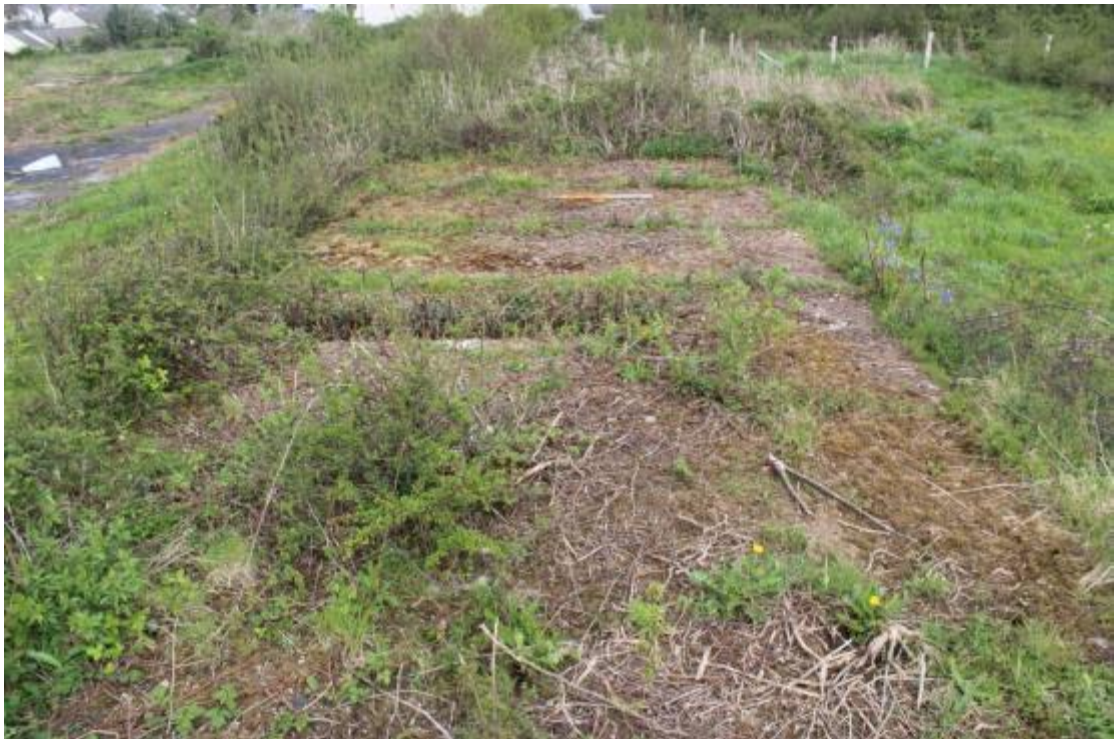
Photo 30: View east: Building 181 (Post Office); well preserved concrete raft measuring c. 10.9m by 4.7m; rectangular slot measuring 2.7m by 0.5 and 0.5m deep at roughly midway point.
