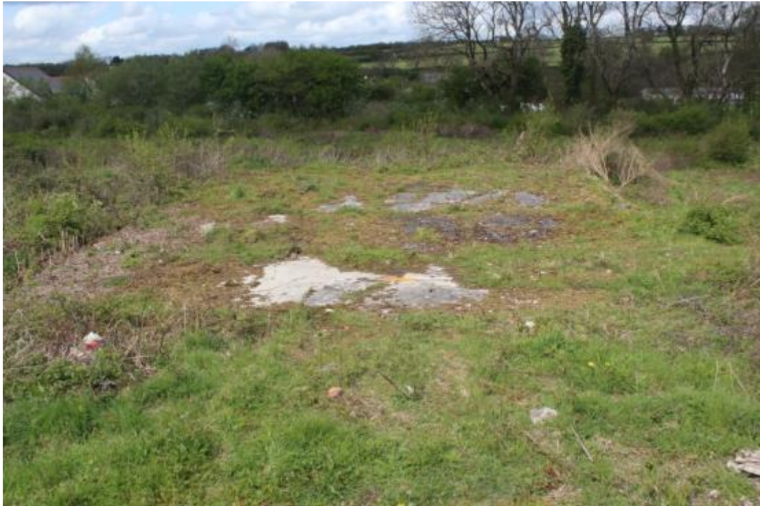
Photo 15: View west: Building 2 (Decontamination Annexe); concrete raft measuring 12.6m by 9.8m; east corner is roughly 1m high; two small extensions, at the north and south ends, shown in the 1946 plan are not visible.
