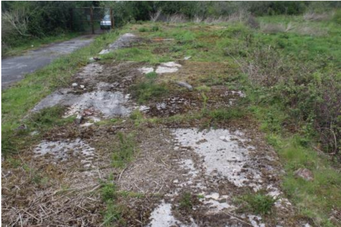
Photo 9: View north: Buildings 29 and 47 (Guards sleeping Quarters/Picket Post and Prophylactic Room) ;concrete raft is approximately 29m long and 5.8m wide; north end is c. 0.9m high from the ground. Brick pilasters/butresses are spaced around the outside of the plinth. A scar is visible halfway along the plinth, dividing 29 and 47; steps lead up from the west side.
