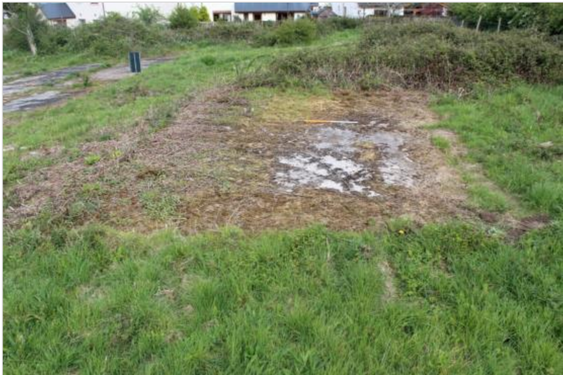
Photo 28: View east Building 63 (MT Office and WAAF Rest Room); intact, well-preserved concrete raft with good edges; measures c. 7.5m by 5.5m.
