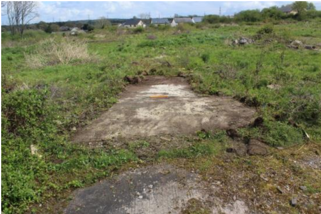
Photo 12: View east: Building 21; concrete floor - edges of floor are grassed over. The visible area is approximately 11.8m long and 3m wide.
