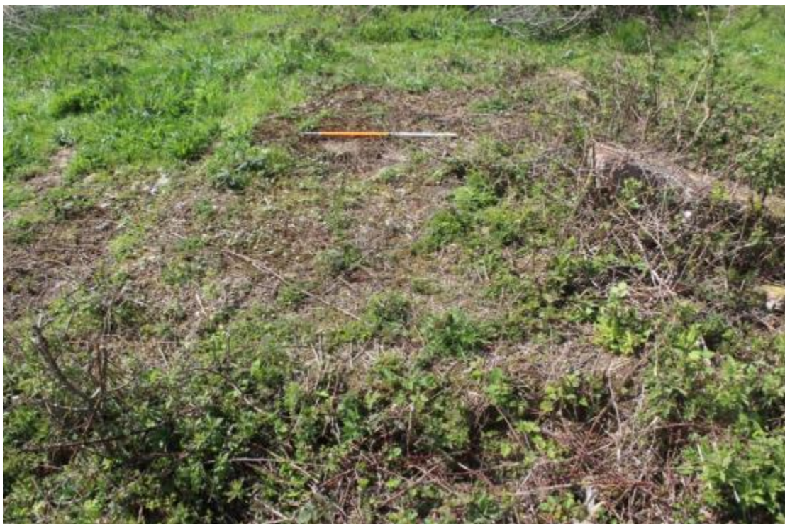
Photo 14: View east: Building 183; small concrete raft measuring approximately 4m by 4m; apart from southwest corner, edges of plinth are well delineated.
