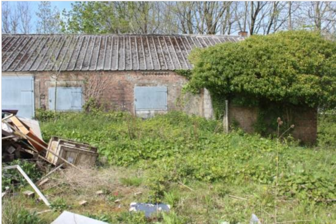
Photo 56: North end of east elevation showing various blocked openings associated with demolished wing (shown in the 1946 Air Ministry Plan).
