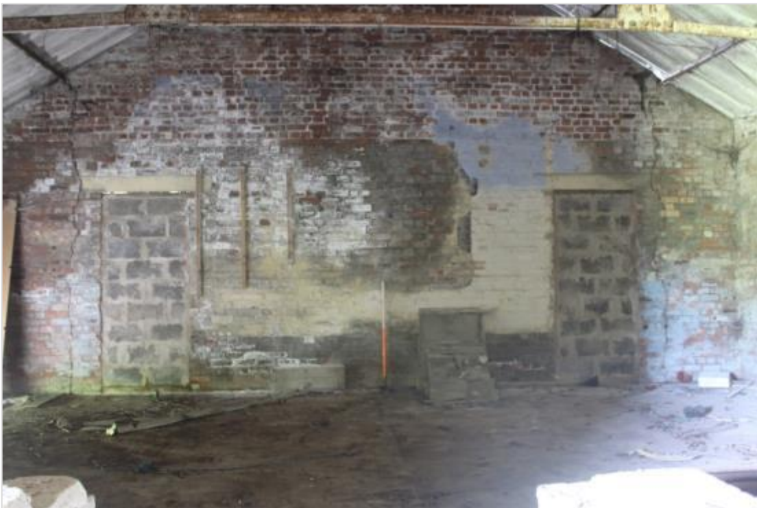
Photo 68: South wall of main room showing two blocked doors that opened onto garage on south side of building.
