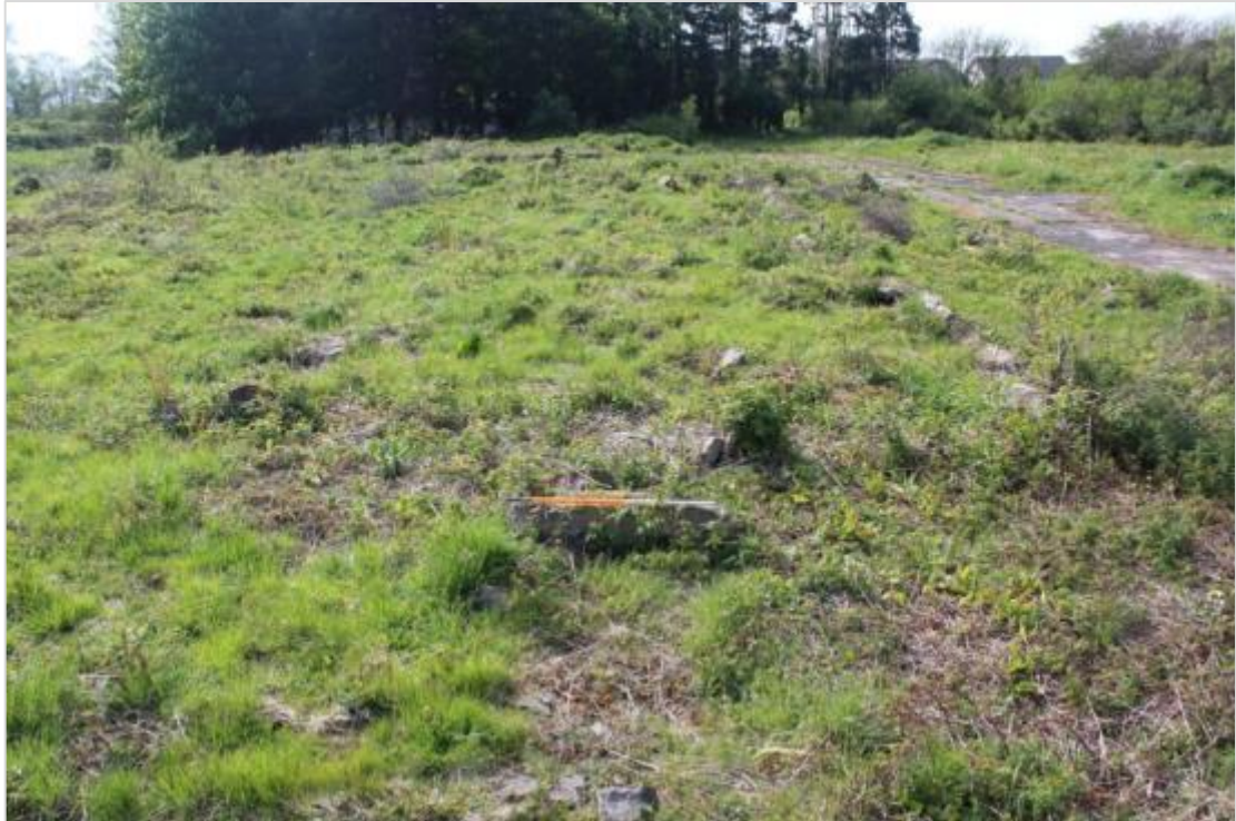
Photo 45: View west: Building 39 (Aircrew Intelligence – Barber and Shoemaker); well-defined north and west edges, rest is rubble strewn and grassed over; area roughly measures 29m by 7m.
