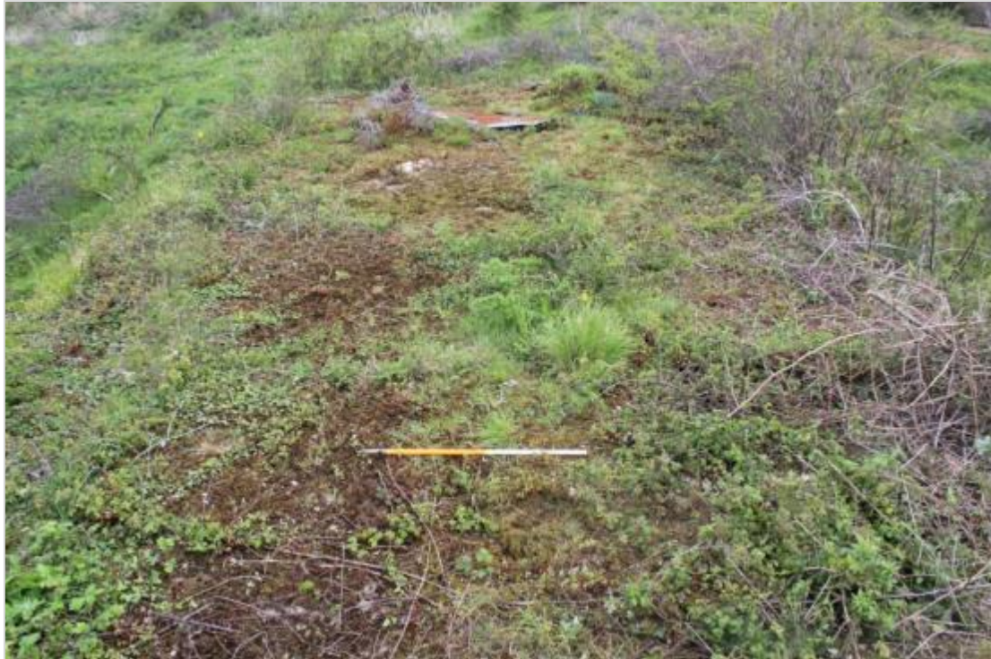
Photo 17: View east: Building 37 (Medical Inspection Block); concrete raft measuring c. 13.6m by 5.8m; vegetation covered with well delineated edges; has survived fairly intact; north face is c. 1m high with pilasters/butresses.
