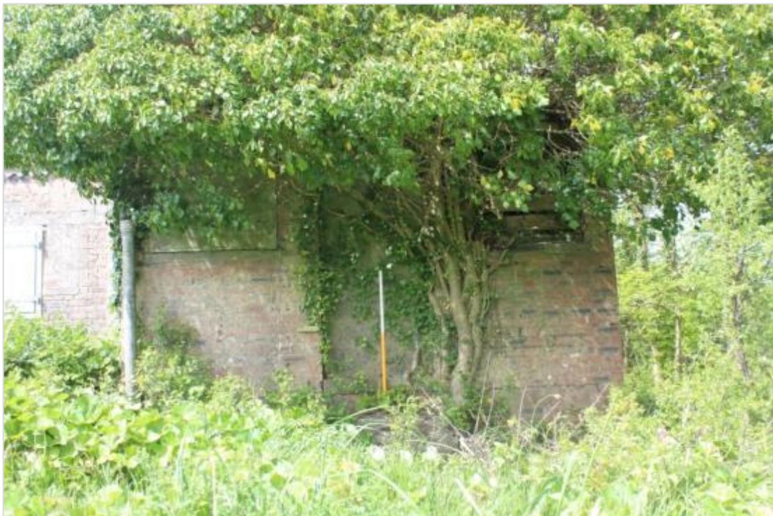
Photo 57: Later brick extension on east elevation with blocked doorway.
