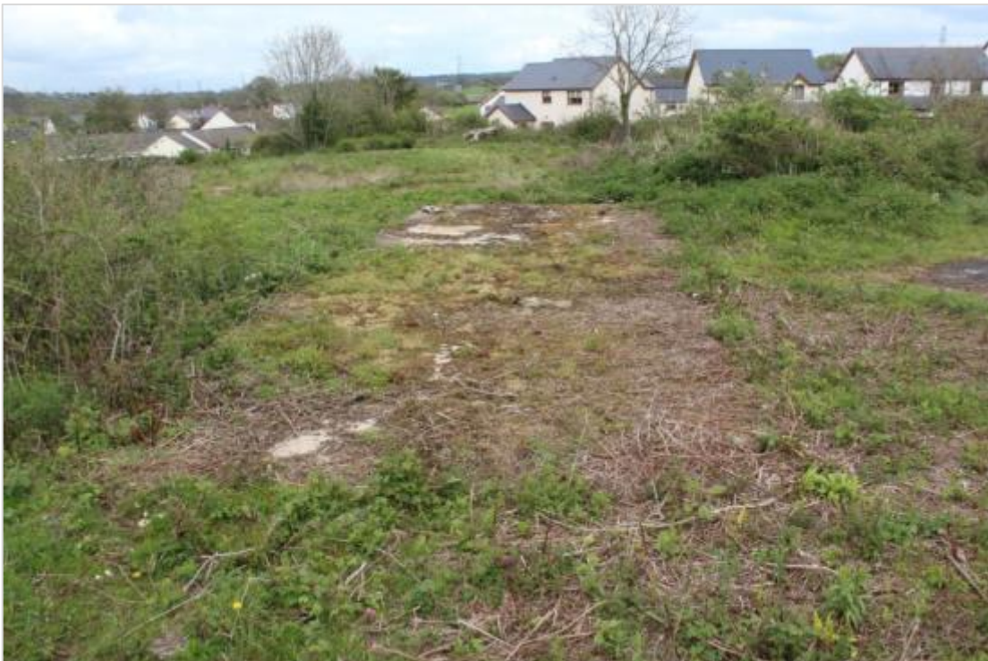
Photo 22: View east: Building 50 (AMWD Office); majority of this concrete raft survives apart from damaged northwest and southwest corners; measures 15.6m by 5.6m. Edge of north side of raft is c. 0.75m high.
