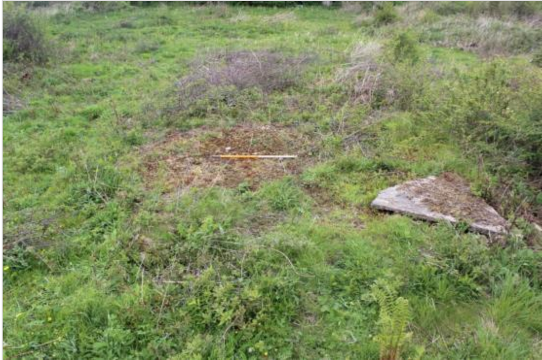
Photo 19: View north; Building 49 (Station Contractors Workshop and Yard); concrete floor measuring c. 4.95m by 3.4m; northeast corner and south edge damaged.
