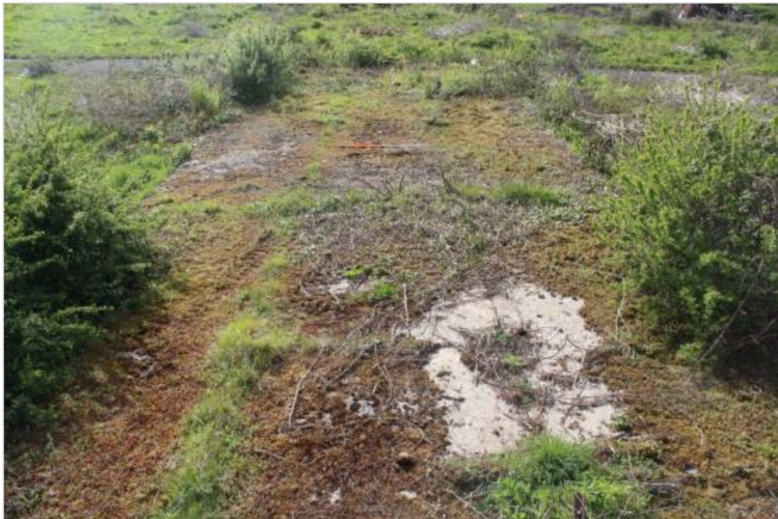
Photo 34: View west: Building 38; well-preserved concrete raft; intact, apart from damaged southeast corner; measures c. 18.6m by 5.6m.
