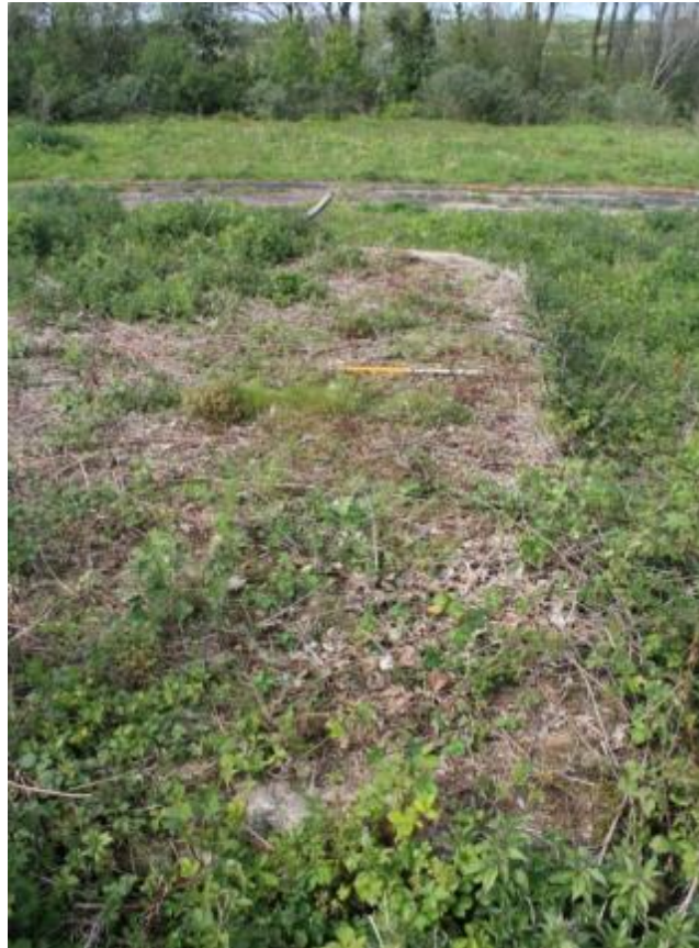
Photo 49: View north: Building 5 (Bath Block and Drying Room); only the northern half of the concrete raft remains; visible area measures c. 7.7m by 5.7m.
