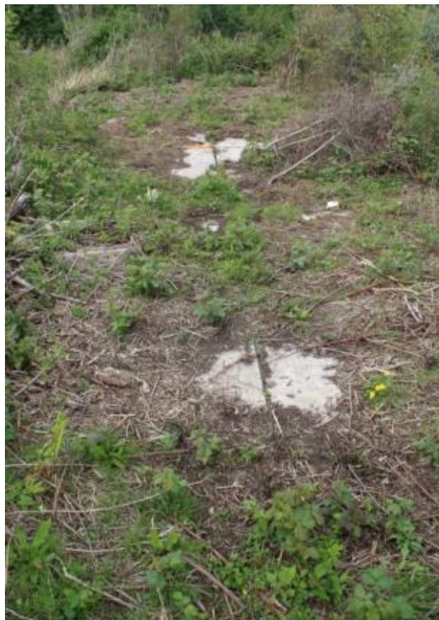
Photo 24: View north: Building 225 (AMWD Stores); concrete floor with seam running down the centre; north edge is damaged, south edge under vegetation; small section of well delineated east and west edges survive; observable area measures c. 14m by 5.6m.
