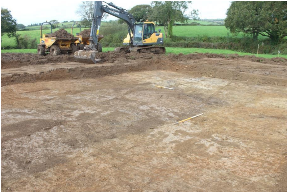
Photo 2: A mechanical excavator with a flat-bladed bucket removing the overburden across the site to reveal archaeological deposits.
