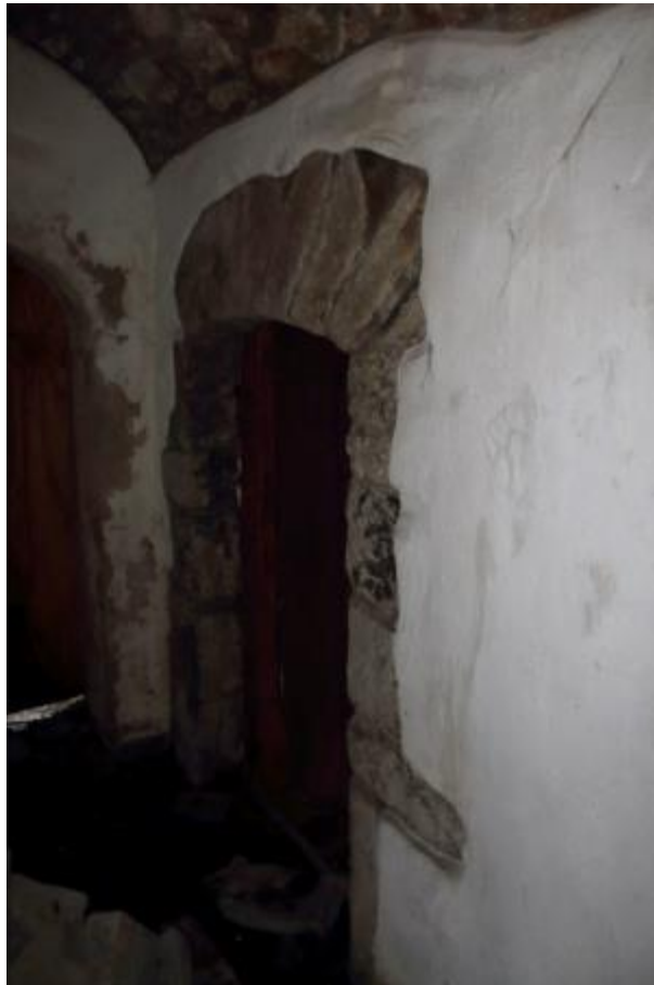
Photo 36: External face of doorway into northern basement unit at its northern end with square reveals and a substantial segmental-headed surround
