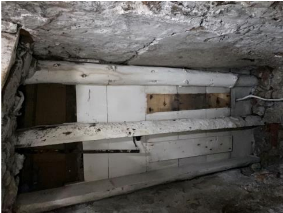
Photo 55: View of roof structure above recess below outshut in No. 6 Castle Terrace, showing modern timber covering with north end to left
