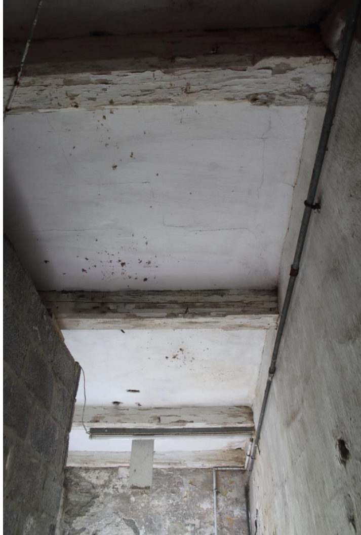
Photo 47: View of ceiling along eastern side of northern cellar below the rear extension of No. 5 showing neat floor joists above with chamfered edges and stops
