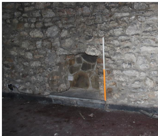
Photo 29: Detail of dummy fireplace in northern part of eastern wall of southern basement unit
