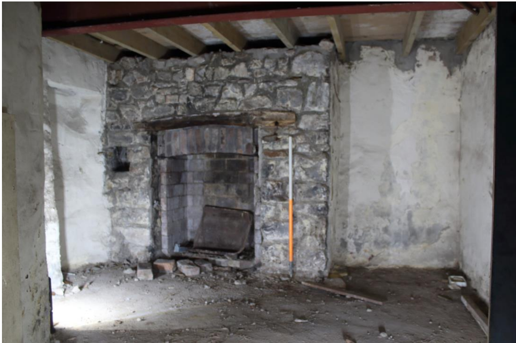
Photo 59: View west of western wall of basement below No. 6 Castle Terrace showing later fireplace addition
