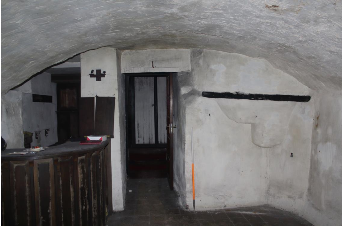
Photo 18: View of south wall of central unit of basement showing square headed entrance passage, corridor through wall (centre), squinch to west (right) and recess to east (left)
