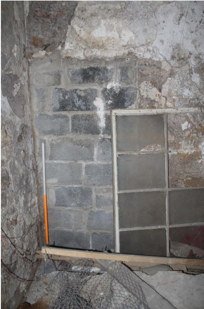
Photo 43: Blocked door way (breeze block) in northern wall of northern basement level of No. 5 Castle Terrace
