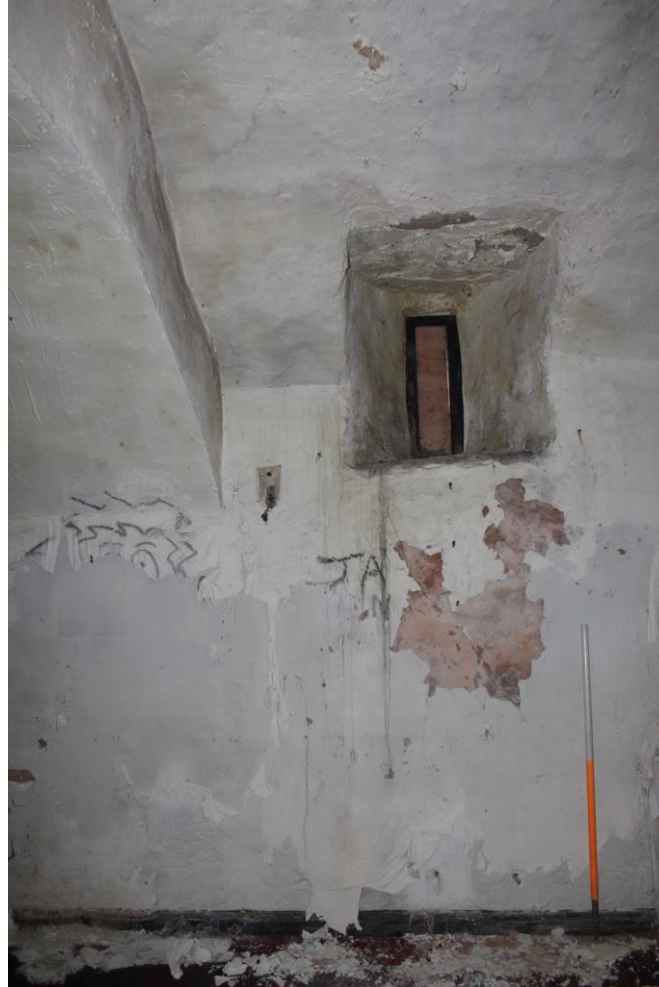
Photo 21: Viewing east of northern small, plain splayed opening in east wall of central unit of basement
