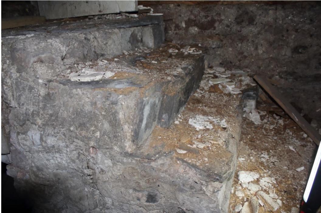
Photo 71: Detail of stone stairs with shale faced treads and risers leading down to basement level
