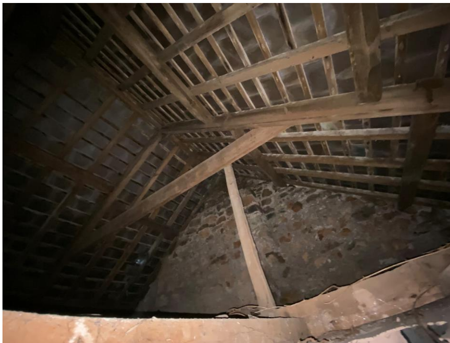
Photo 70: View southeast into roof space showing pegged trusses
