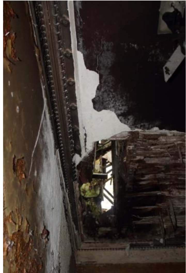
Photo 10: View of cornice detail above central passage from original front door showing partially collapsed roof
