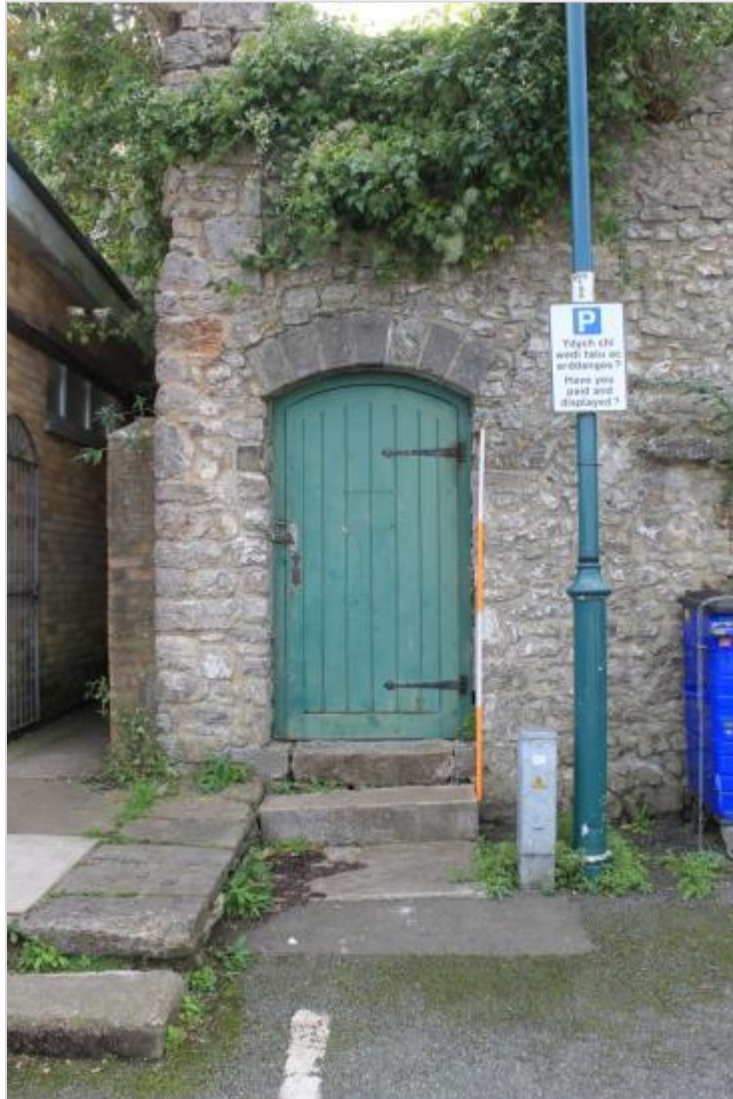
Photo 85: Entrance to No. 4 Castle Terrace from South Quay. The existing segmental head is a modern reconstruction.
