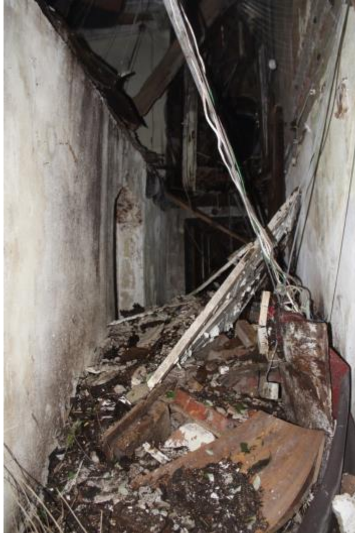
Photo 41: View south along uncovered passage way between Nos. 4 and No. 5 Castle Terrace, showing western wall of central basement unit to east (left) and doorway opening to No. 4 visible (with possible corbels to south) and collapse from structures above
