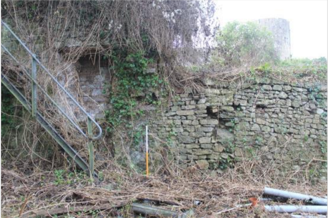
Photo 98: Southern end of east face of wall (PRN 115030) dividing burgage plots at Nos. 5 and 6 Castle Terrace. A joint is visible approximately 2m to the right of the 1m scale. Above the scale the stub of an east-west wall is visible (the other end of which can be seen in Photo 100). A blocked window is visible to the left of the scale (see Photo 115 for other side). 1m scale
