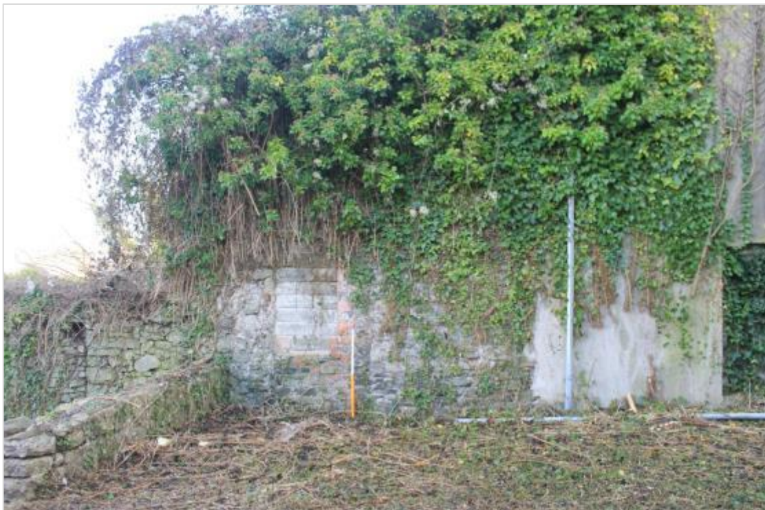
Photo 115: Blocked opening in west facing wall in burgage plot at No. 6 Castle Street (see Photos 98 & 99 for other side). 1m scale
