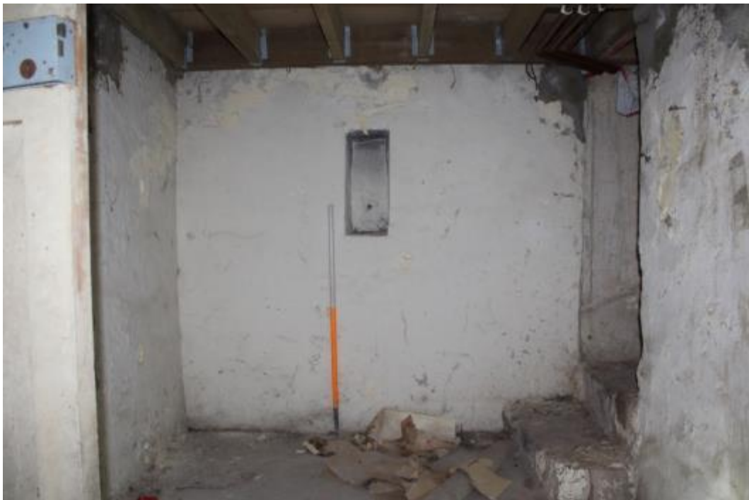
Photo 58: Eastern wall of basement below No. 6 Castle Terrace showing small alcove and stair access to south (northern wall is modern and of breezeblock)
