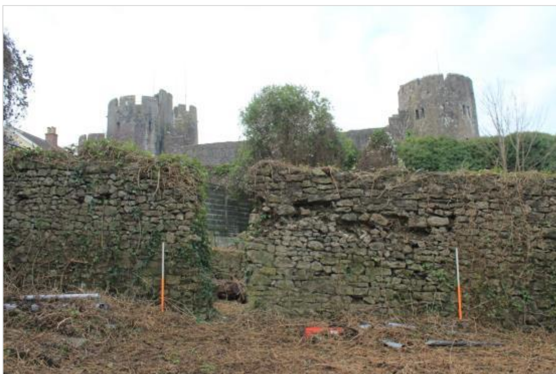
Photo 97: View west towards breach in wall (PRN 115030) dividing burgage plots at Nos. 5 and 6 Castle Terrace. End of wall at north side of breach possibly squared, south side is rough. Wall south of breach is wider than northern wall suggesting different phases of construction. 2 x 1m scale
