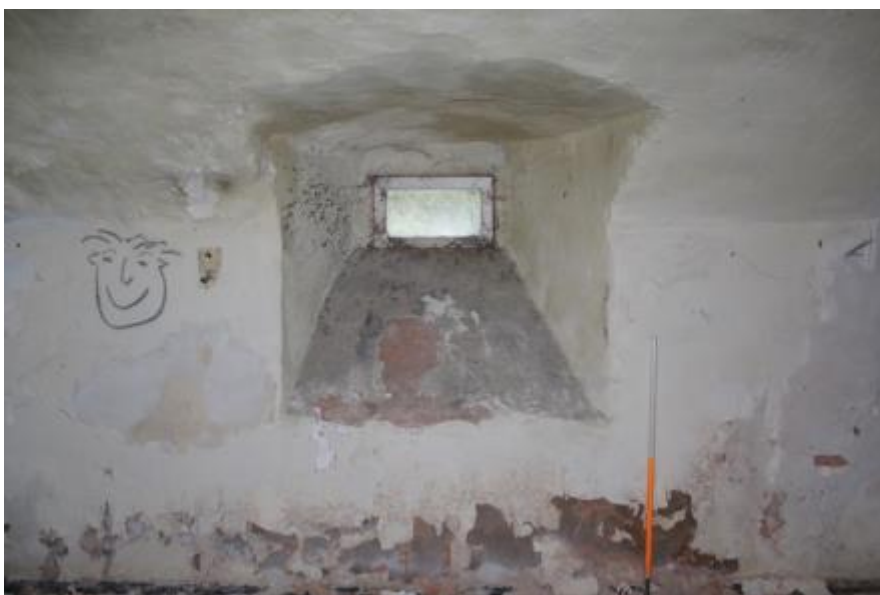
Photo 35: View east of southern light opening in eastern wall of northern basement unit with steep sloping sill
