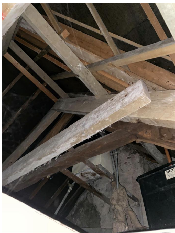
Photo 52: View of roof timbers in No. 6 Castle Terrace through loft hatch to southwestern side, showing modern replacement trusses with earlier ones behind
