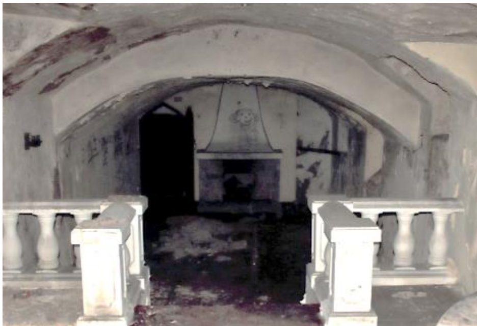
Photo 33: View north from central basement unit to northern basement extension, showing reduction in vault height
