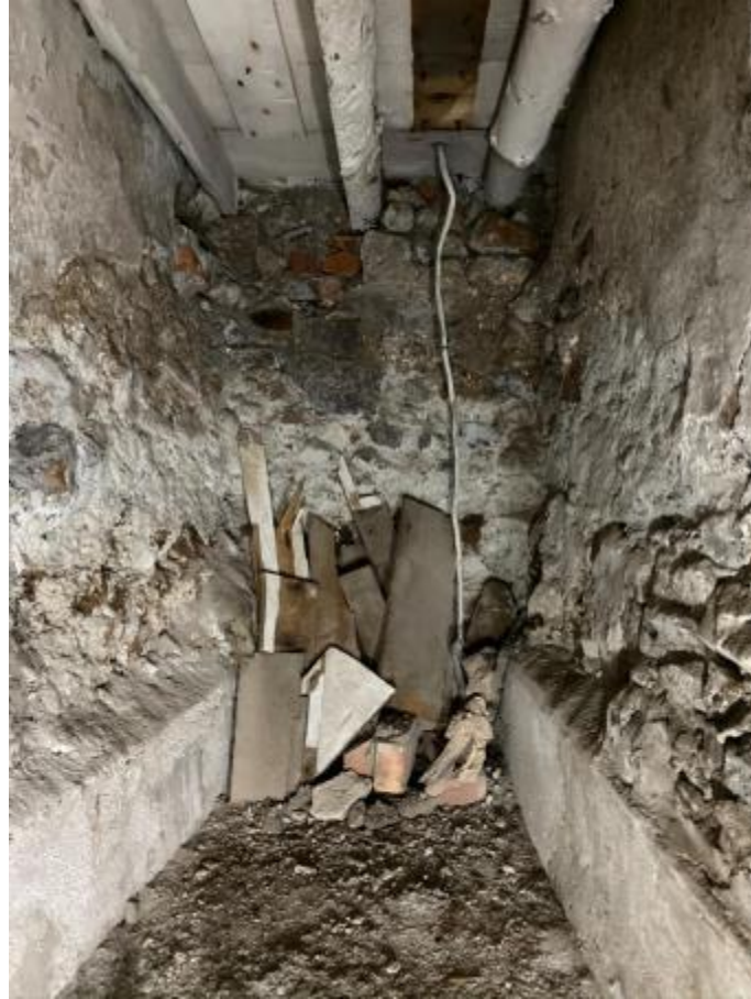
Photo 56: View south along recess to southern end showing bedrock at lower parts of sides with modern concrete underpinning
