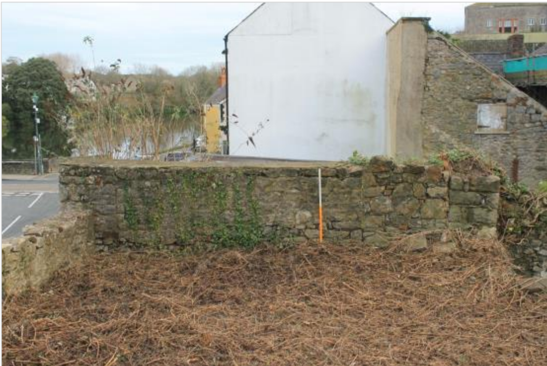
Photo 87: View east towards wall situated above covered passageway in burgage plot at No. 4 Castle Terrace (note blocked opening to right of 1m scale)
