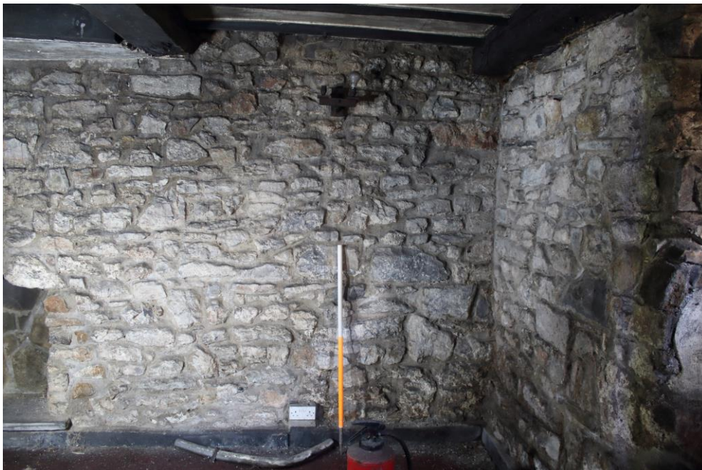
Photo 24: View east of eastern wall of southern basement unit showing the south wall butting against the east wall
