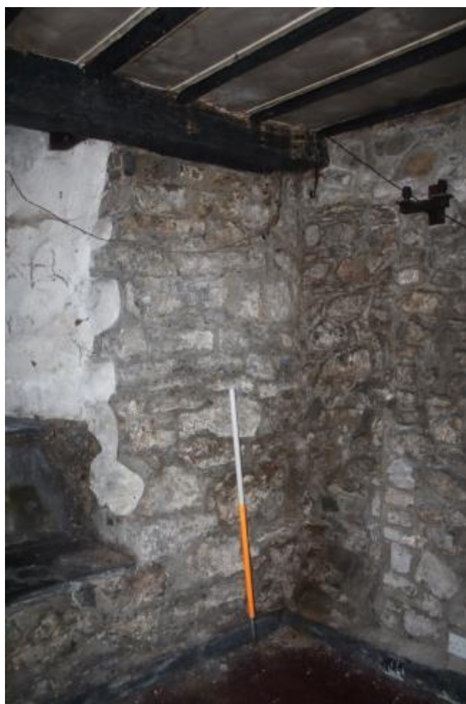
Photo 25: View southwest of corner of southern and western walls of southern basement unit showing bonded walls in the lower part and possibly butting above
