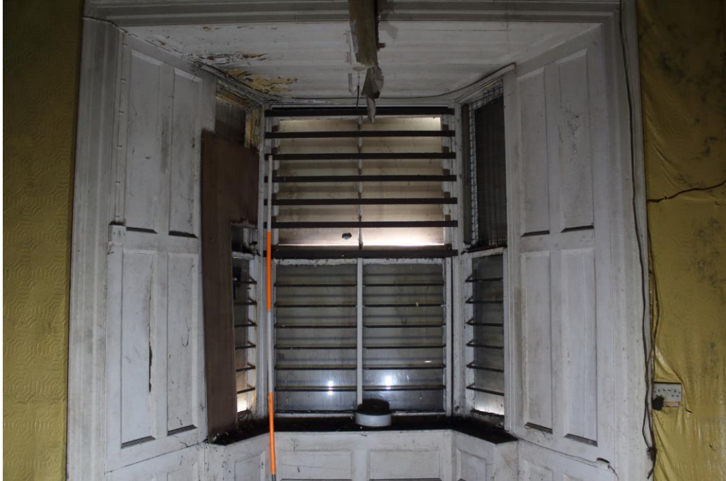
Photo 15: View south of bay window with sunk timber panelling to sides in southern room of No. 5 Castle Terrace
