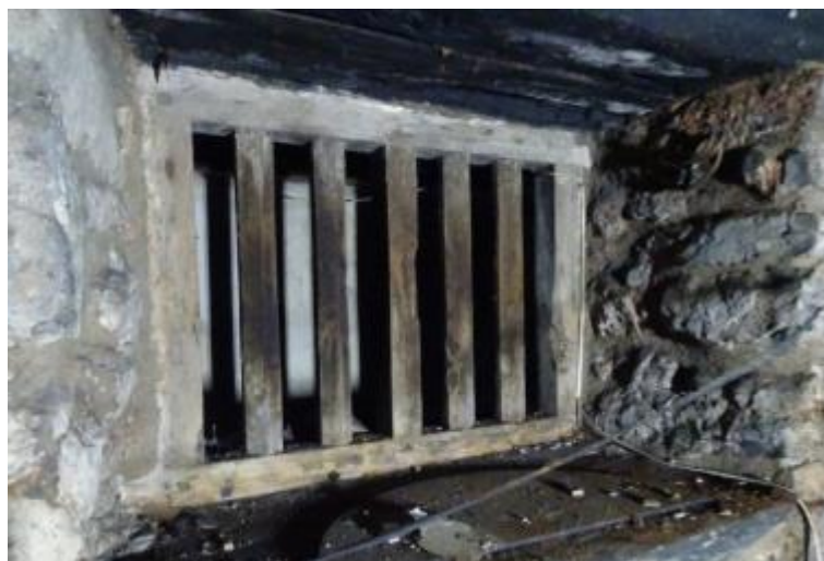
Photo 27: Detail of C16 th -C17 th unglazed timber framed window in west wall
