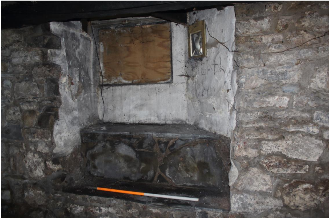
Photo 28: Window light in southern wall of southern basement unit roughly at Castle Terrace pavement level
