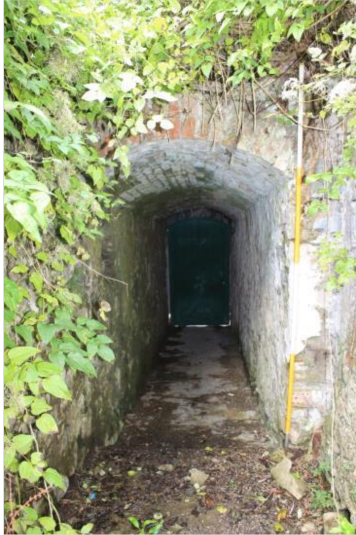
Photo 84: View north of brick vaulted passage leading to South Quay from rear of No. 4 Castle Terrace
