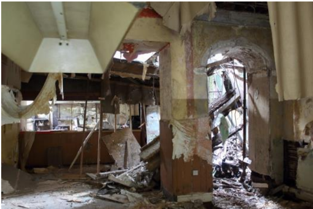
Photo 14: View north across southern room of No. 5 Castle Terrace, showing wide internal partition wall looking through to bar area and collapsed superstructure and roof
