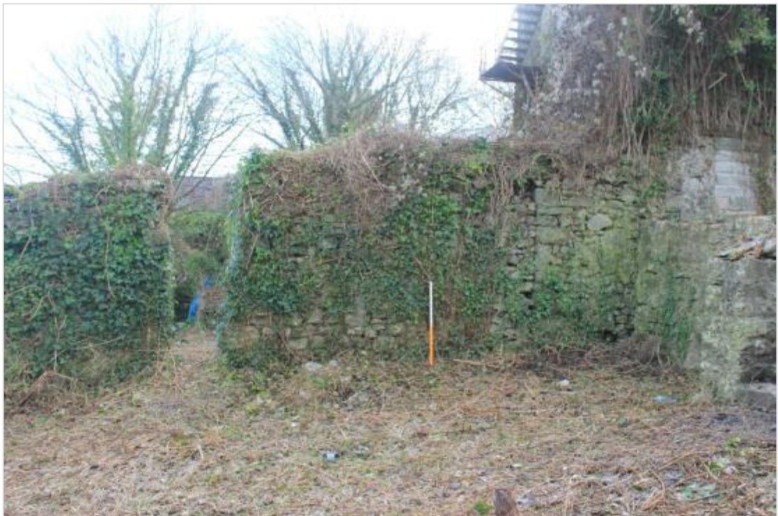
Photo 113: Southern end of west face of wall (PRN 115030) dividing burgage plots Nos. 5 and 6, Castle Terrace. Note masonry joint in wall to the right of the 1m scale: the wall to the left of the joint is quoined and the wall to the left of the breach also has remains of quoin work implying that the wall between the joint and the breach is a later insertion. 1m scale
