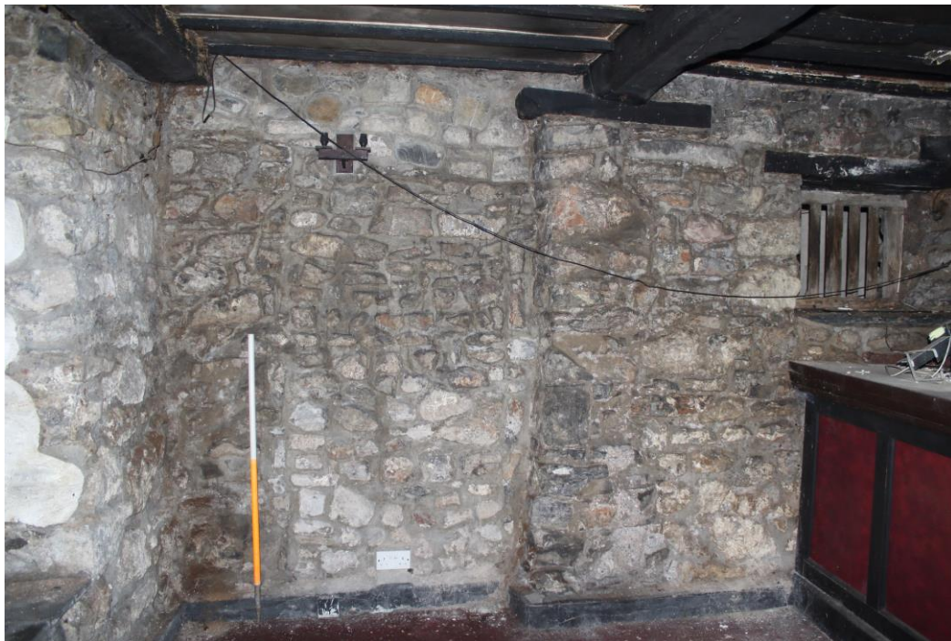
Photo 26: West wall of southern basement unit showing window light to left and blocked doorway by scale
