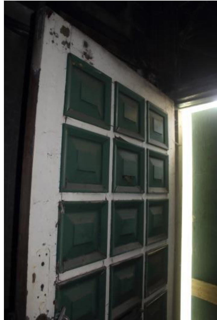
Photo 4: Elaborate fielded 18-panelled door of late-Georgian form within the original doorway to Nos.4 and 5 taken from inside original entrance corridor
