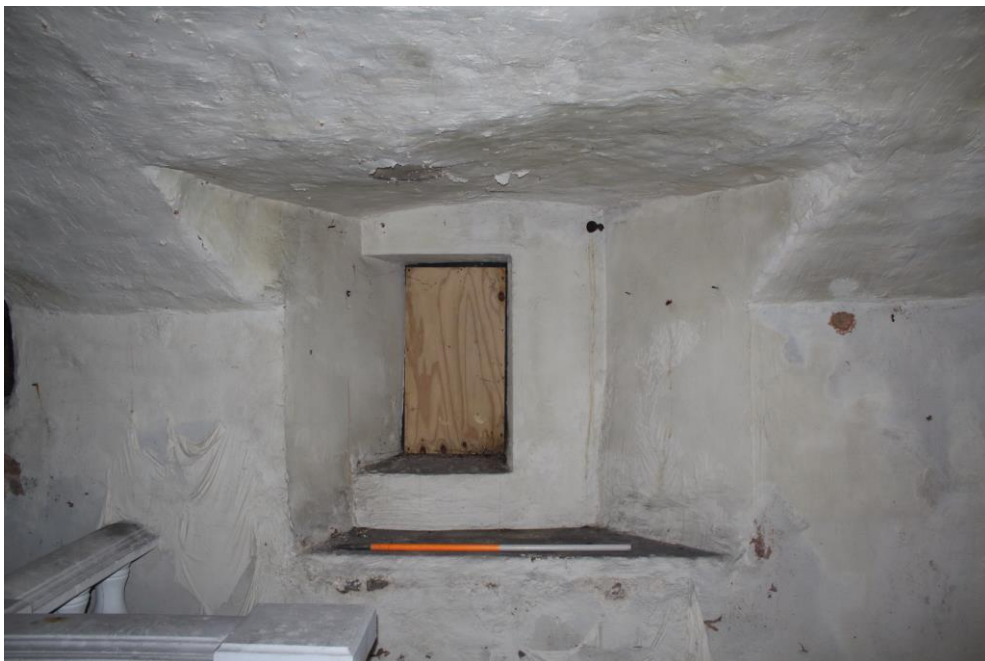
Photo 22: View east of larger splayed window in eastern wall of central unit of basement with lower sill and rectangular opening
