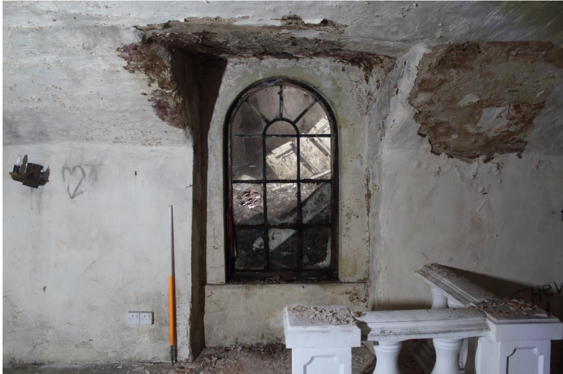
Photo 23: View west of doorway to corridor from central vaulted unit of basement, with modern 'Georgian' window insertion
