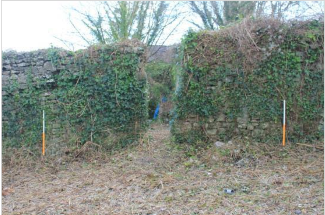
Photo 112: View east towards breach in wall (PRN 115030) dividing burgage plots Nos. 5 and 6 Castle Terrace. End of wall on left side of breach possibly squared: right side is rough. Wall left of breach is wider than wall on right, suggesting different phases of construction. 2 x 1m scale
