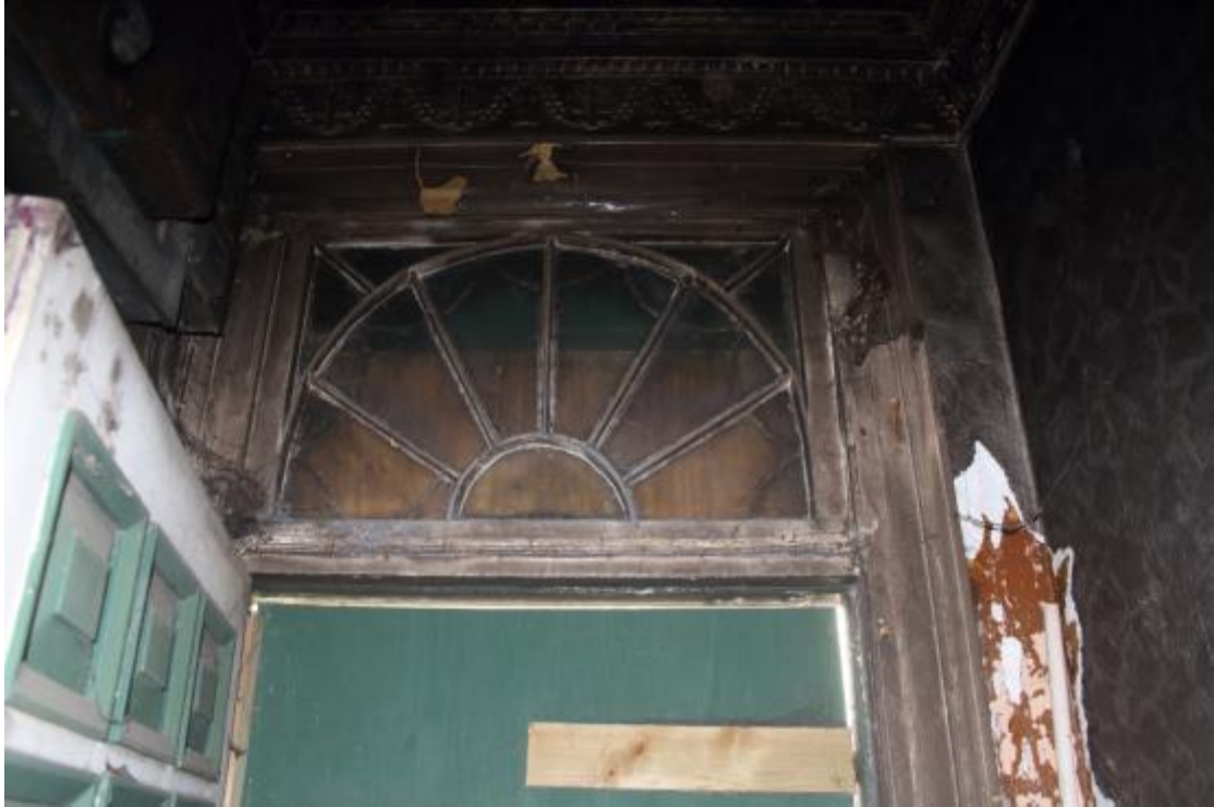
Photo 5: View south of oversight above original doorway in Nos. 4 & 5 showing fine contemporary fan tracery, viewed from original entrance corridor
