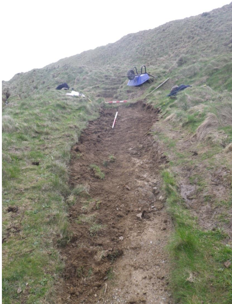
Porth y Rhaw: cut and fill of water erosion gully in path below new step. Scales 0.5m and 1m. View SE. 10/4/2014
