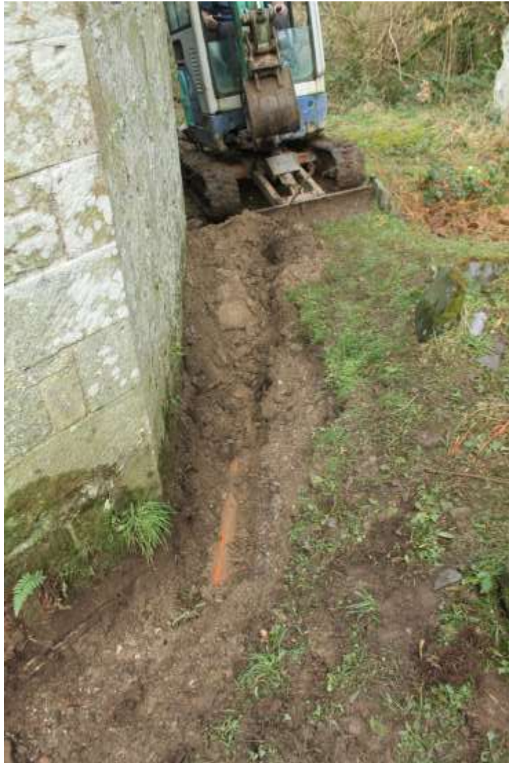
Photo 6: Ceramic drain pipe exposed in the drainage trench on the eastern end of the chancel
