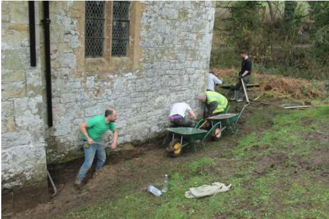
Photo 5: Hand removal of the drainage trench on the southern side of the chancel
