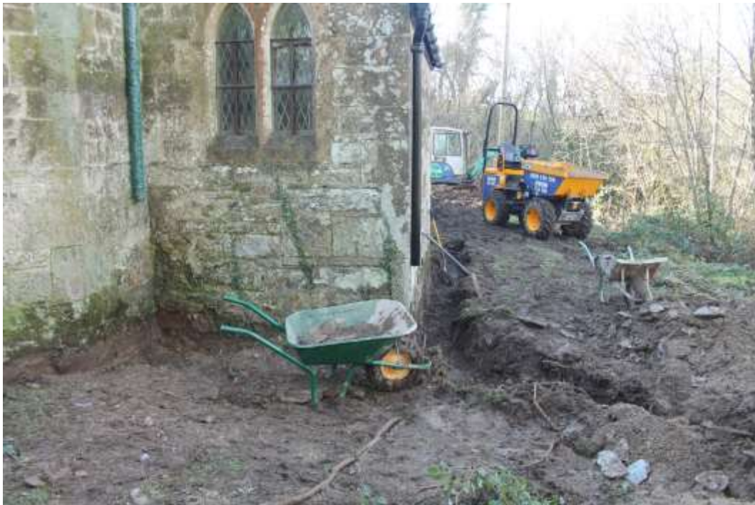
Photo 9: Junction of perimeter drainage trench and run off drain at northeastern corner of chancel
