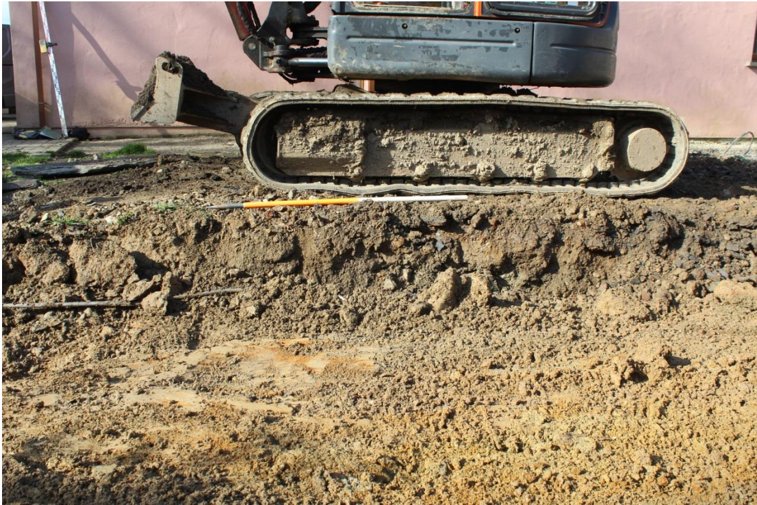
Photo 3: View west, showing depth of made-up ground that was removed (1m scale).
