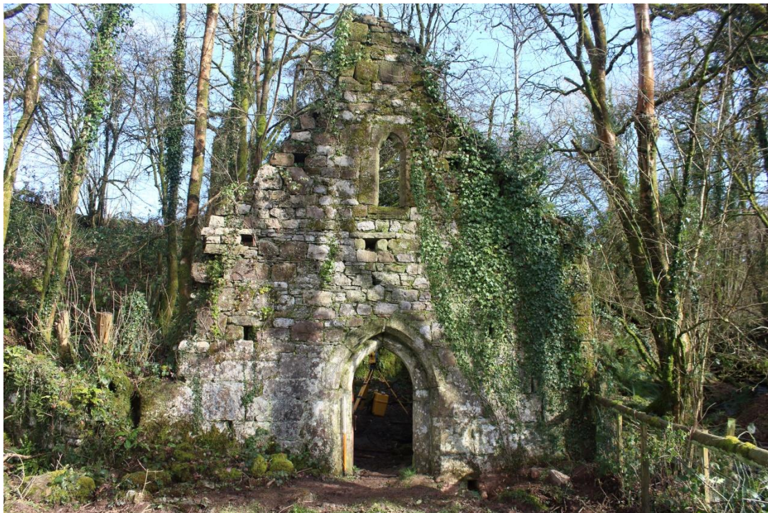
Photo 2: Western wall (exterior view) housing the bellcote, arched entrance doorway, trifoliated lancet window and water spout.
