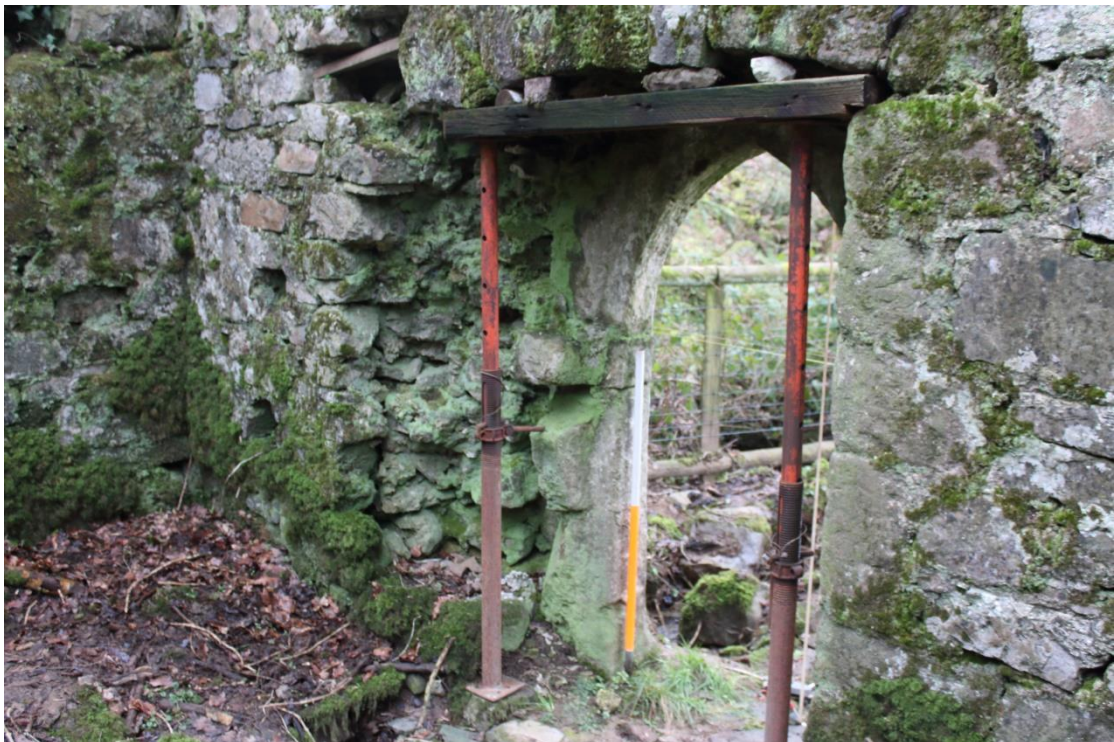
Photo 4: The arched doorway in the western wall, currently being held up by acrow props. To the left of the door the masonry suggests a possible staircase once led to the bellcote.
