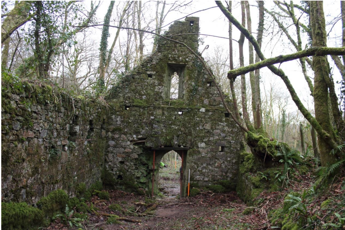
Photo 3: Western wall (interior view) housing the bellcote, arched entrance doorway, trifoliated lancet window.
