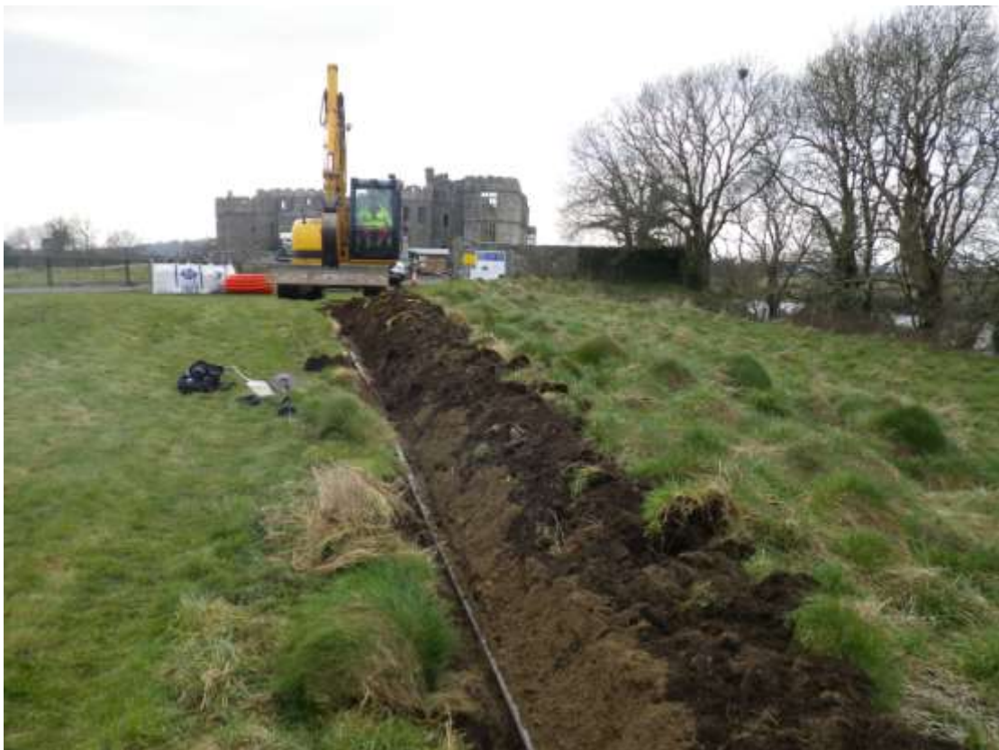
Photo 3: View west towards Walled Garden showing excavation of service trench (for water and electric) across grassed area on brow of slope (PCNPA 2013)
