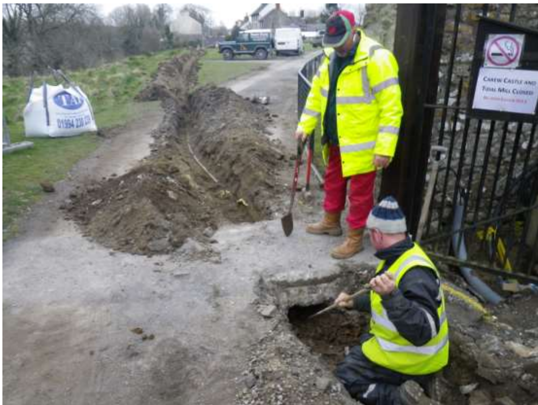
Photo 1: View east from entranceway into Walled Garden showing excavation of service trench (for water and electric) (PCNPA 2013)
