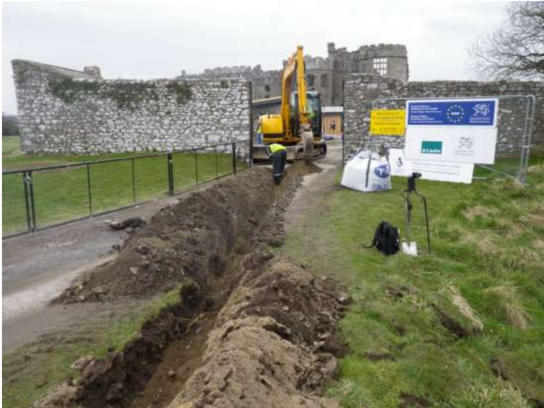
Photo 2: View west towards entranceway into Walled Garden showing excavation of service trench (for water and electric) (PCNPA 2013)
