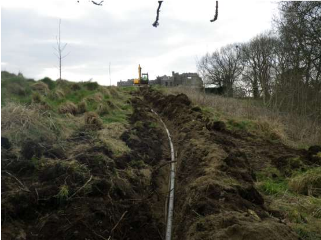
Photo 4: View west towards Walled Garden showing excavation of service trench (for water and electric) on the downslope area leading towards Carew Inn (PCNPA 2013)
