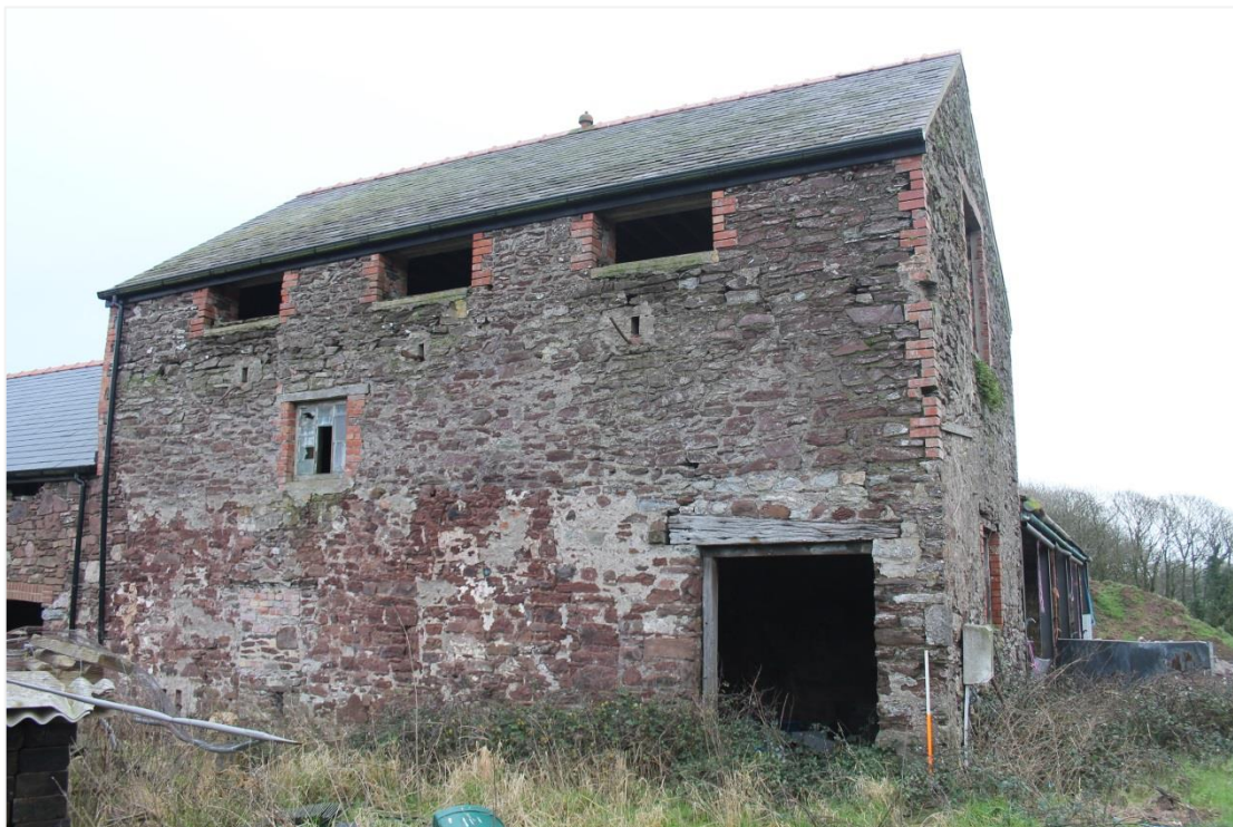
Photo 5: West wall of granary. Quoins denote layer phase of building. 1m scale
