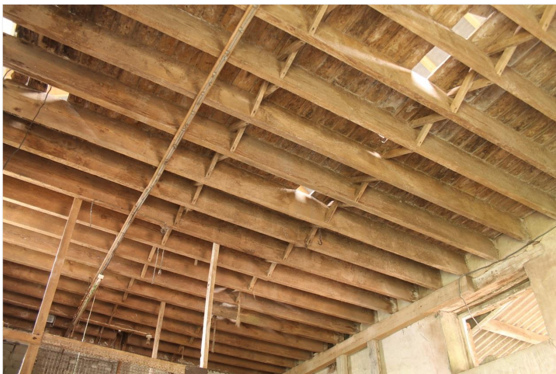
Photo 26: Timberwork in granary ceiling.
