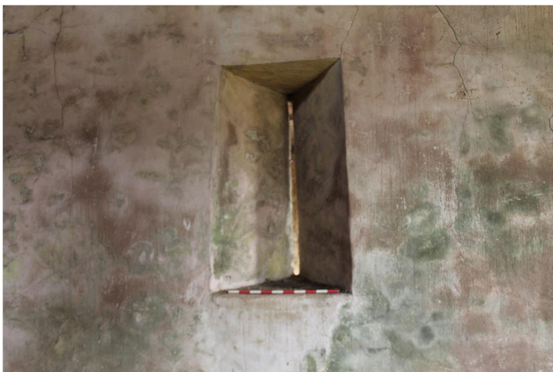
Photo 22: Close-up of ventilation slot. 0.5m scale
