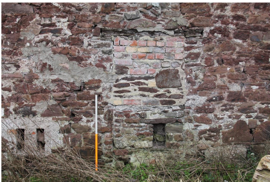
Photo 8: Blocked opening in west wall of granary. 1m scale
