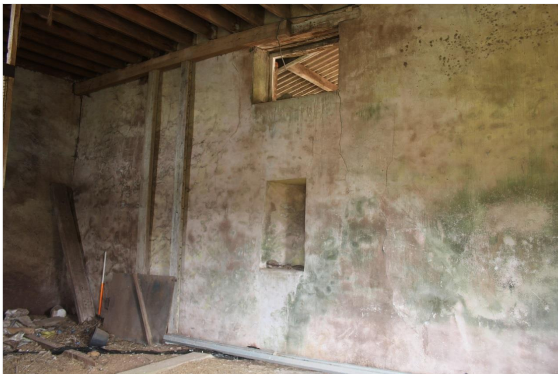
Photo 21: Interior east wall of granary, showing ventilation slot and smooth cement render. 1m scale
