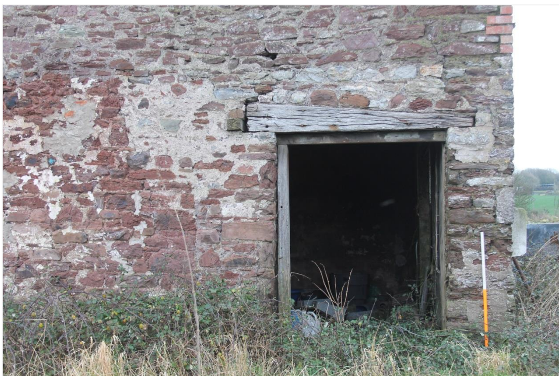
Photo 6: Doorway in west wall. Note change in stonework above lintel indicating later phase. 1m scale
