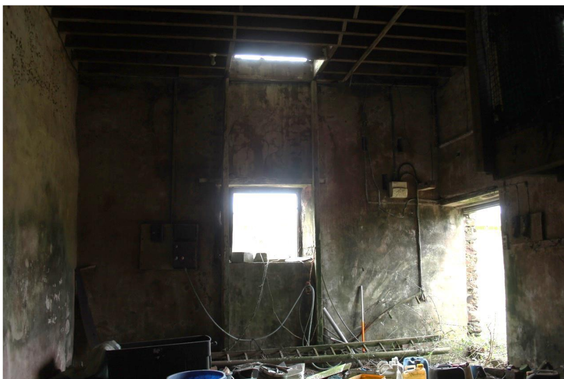
Photo 24: Smooth, cement rendered, south wall of granary. 1m scale
