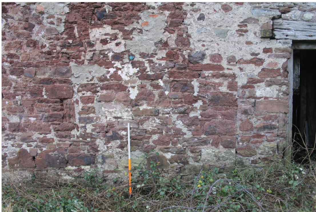
Photo 7: Joints in west wall of granary. 1m scale
