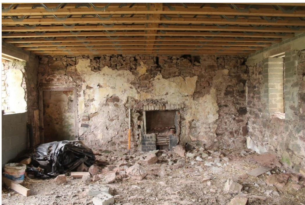
Photo 14: Interior of north wall of farmhouse showing blocked doorway utilised as recessed cupboard and fireplace. 1m scale
