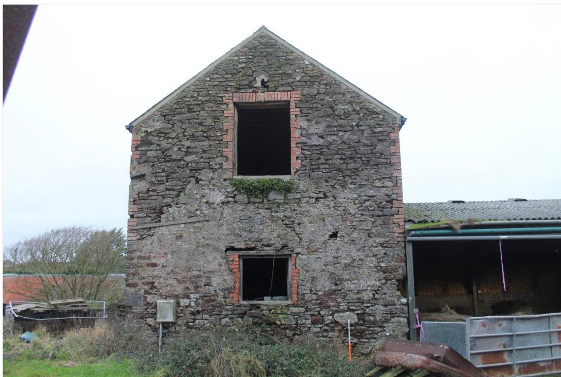
Photo 4: South wall of granary. Lower window might be a later insertion due to brick surround 1m scale
