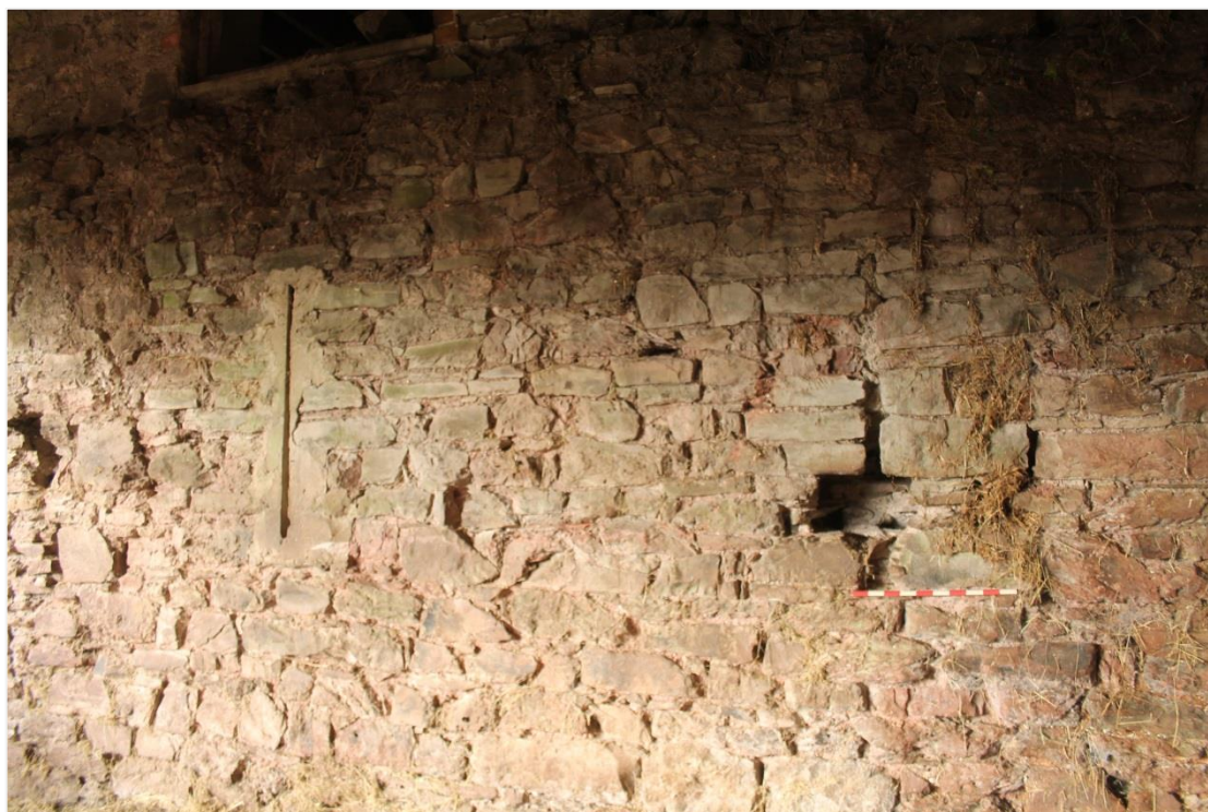
Photo 2: Close up of ventilation slot in east wall and remains of another slot to the right. 0.5m scale.
