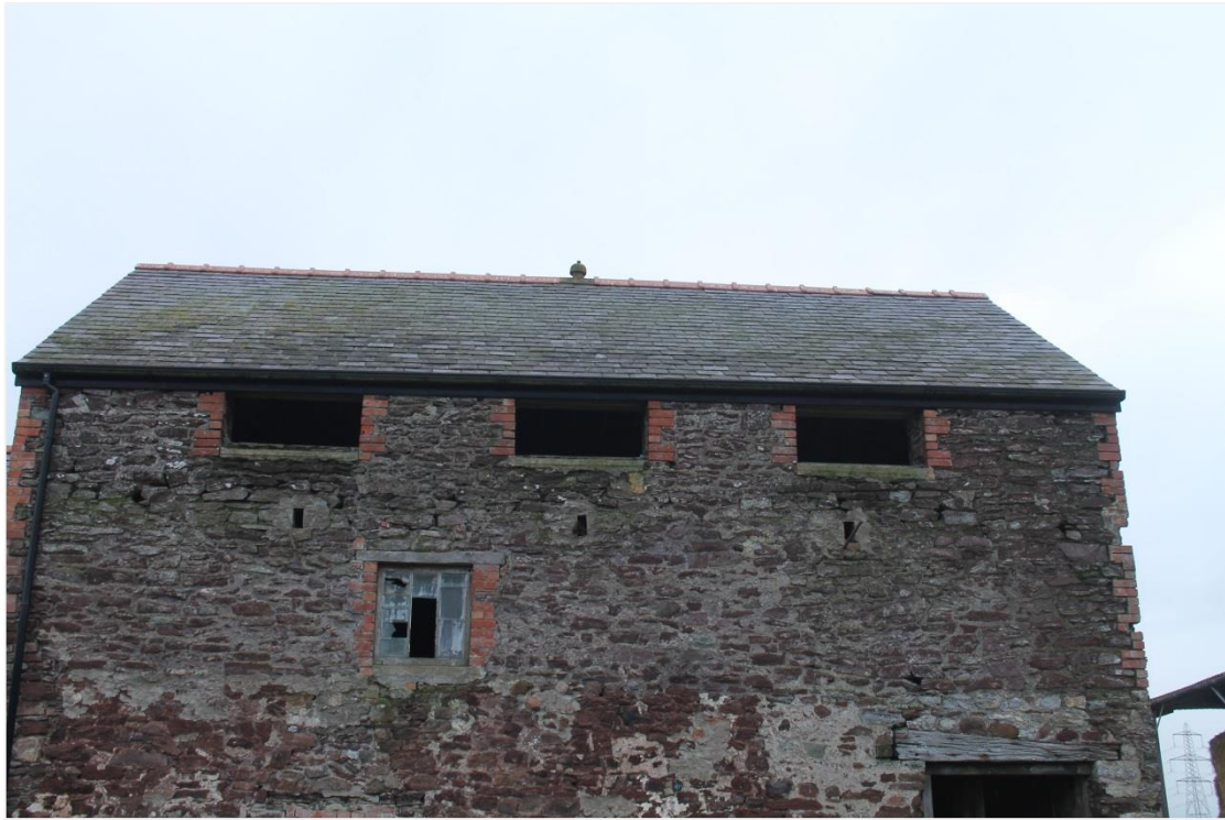
Photo 9: West wall of granary showing later, 1 st floor addition.
