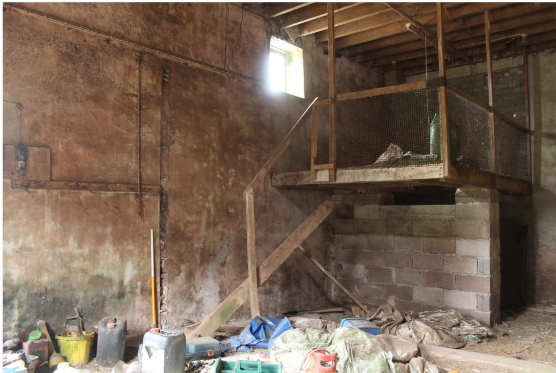
Photo 23: Smooth, cement rendered, west wall of granary. 1m scale
