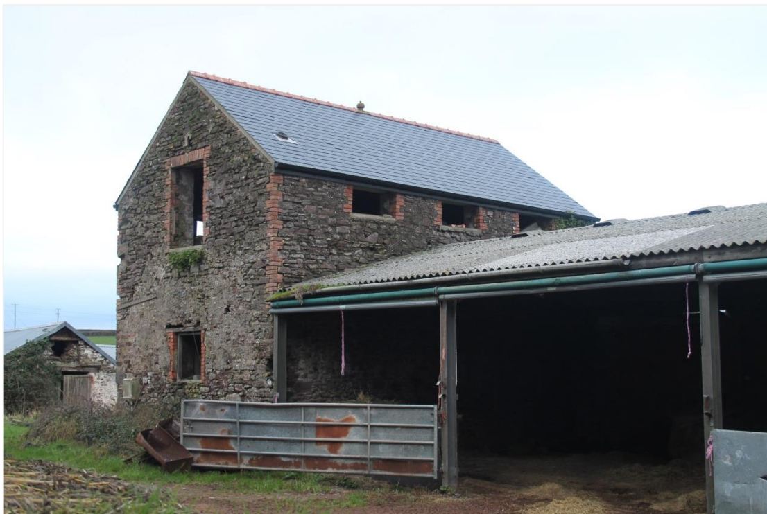
Photo 3: Southeast corner of granary; brick quoins indicate later building phase.
